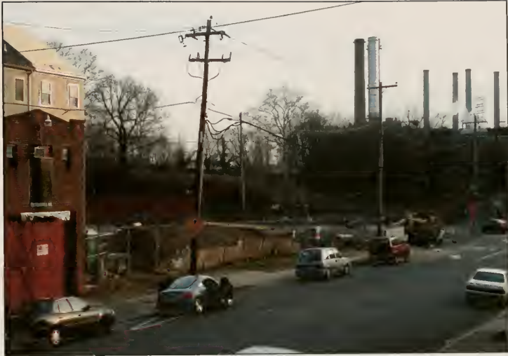
Figure 50 View of the rear of the Naval Home site showing the break in the perimeter wall.
