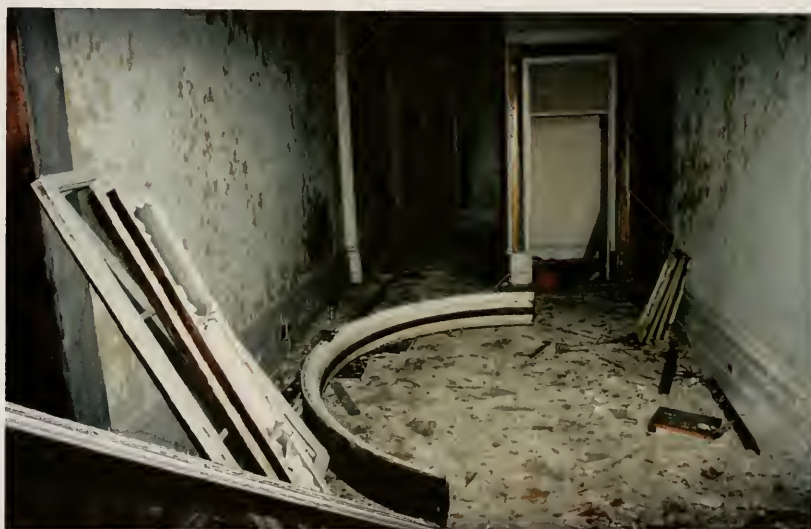
Figure 44 Arched trim in Surgeon General's Residence, January 2000.
