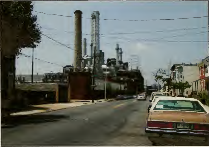
Figure 55 The PECO Energy Plant creates an industrial barrier for residential development.
