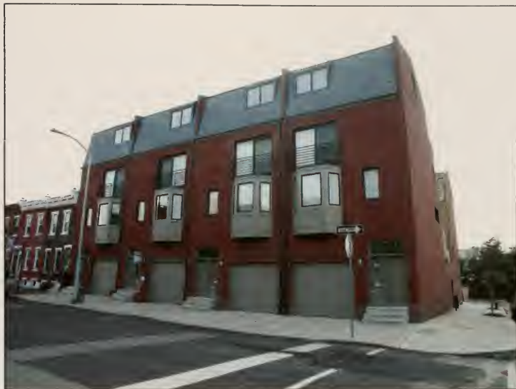
Figure 52 River Park Place Phase I. New townhomes constructed by Prudential Fox & Roach in the residential neighborhood to the north of the Naval Home.
