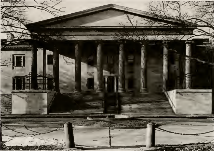
Figure 11 Main Entrance and portico of Naval Home, East Elevation.
