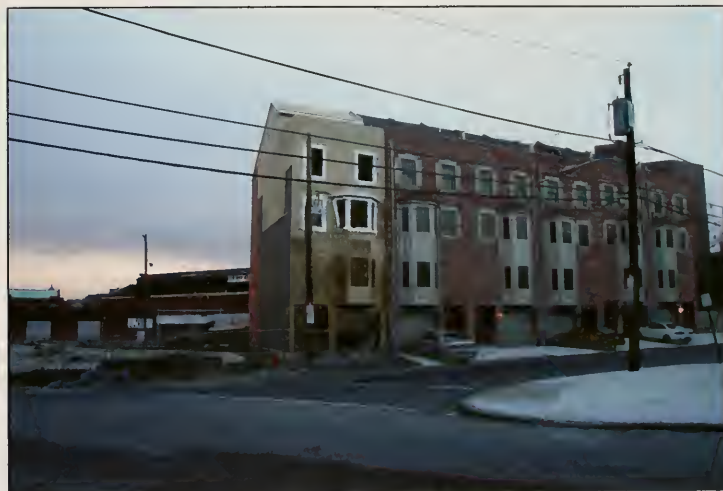
Figure 53 Southbridge. New townhomes built by Coldwell Banker at the corner of Banbridge and 27th Streets.
