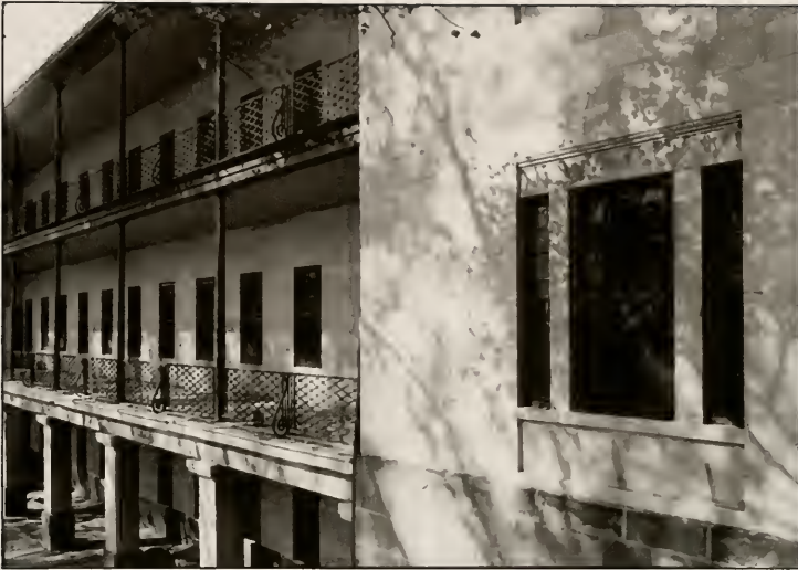
Figure 13 Detail of Verandas, West Wing.
