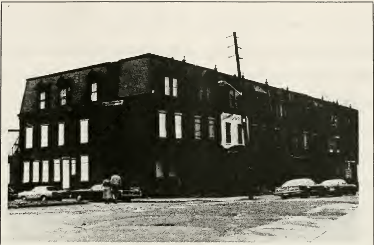
Figure 1. Cooper Plaza Historic District, 638-620 Benson Street Camden, NJ. This photograph shows the condition of the buildings in the district in 1983 prior to rehabilitation. The interiors of these buildings were stripped of all decorative features or were the victims of arson. Many porches had collapsed and windows were smashed. These buildings were in better condition than the majority of buildings in the district. This photograph is typical of those included with the RITC applications. Photograph by Scott Doyle from the Historic Review Committee File, 638 Benson Street, City Hall, Camden, NJ.
