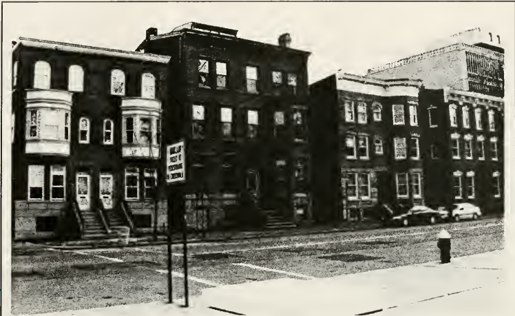
Figure 5. Looking east along West State Street. The setback of the glass-enclosed stairwell is barely visible and does not disrupt the streetscape. Photograph by Scott Doyle.
