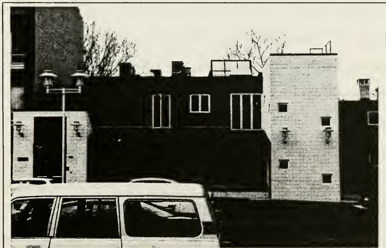
Figure 6. The rear elevation of 186-90 West State Street with the NJEAA building to the left. The back stairwell and elevator are housed in the white tower. The tile work is above the entrance to the left. Photograph by Scott Doyle.
