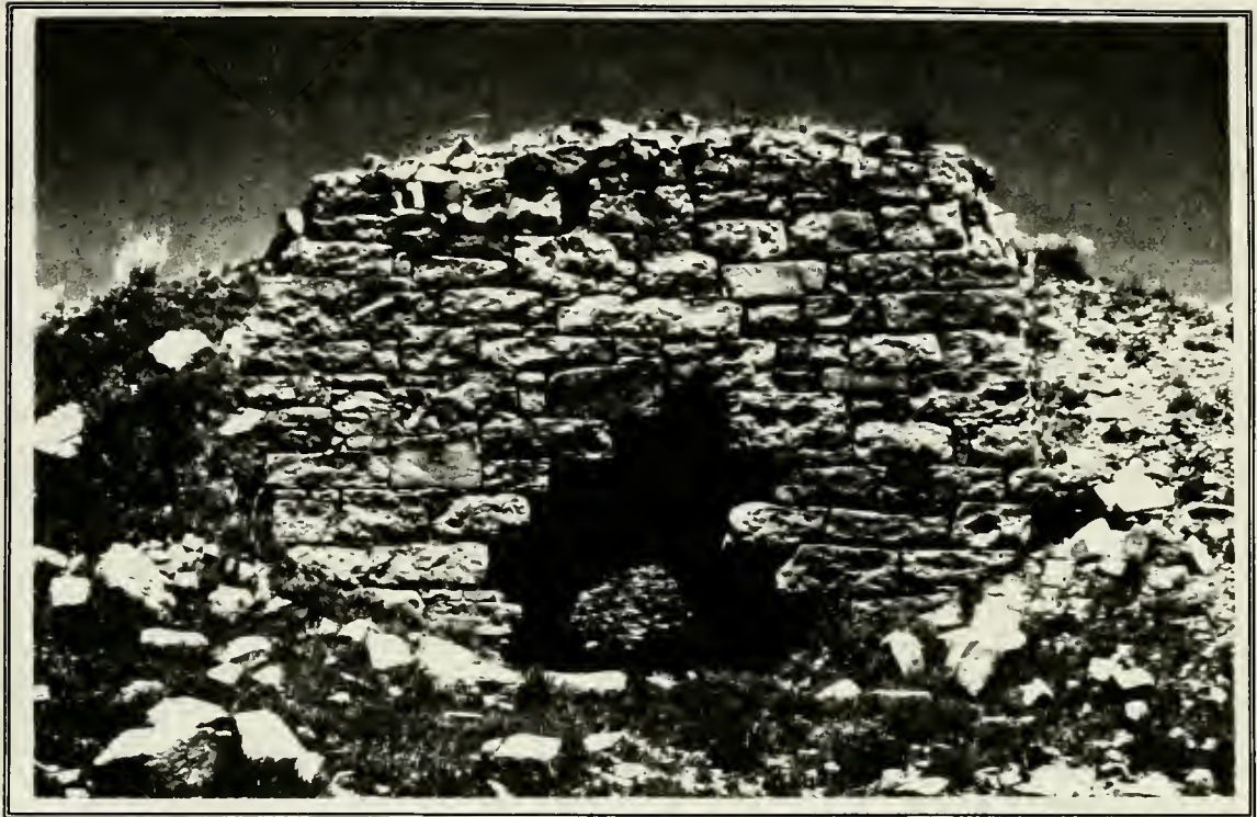
Figure 32: Lime Kiln Ruins Adjacent to Fort Union National Monument Boundaries (Photo by Author)
