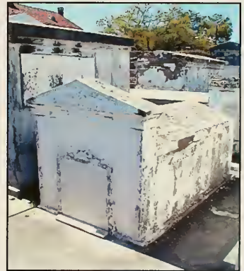
Fig. 6.14 Neglected surface finishes, cracks and biological growth evident. Studio photograph, March 2001.
