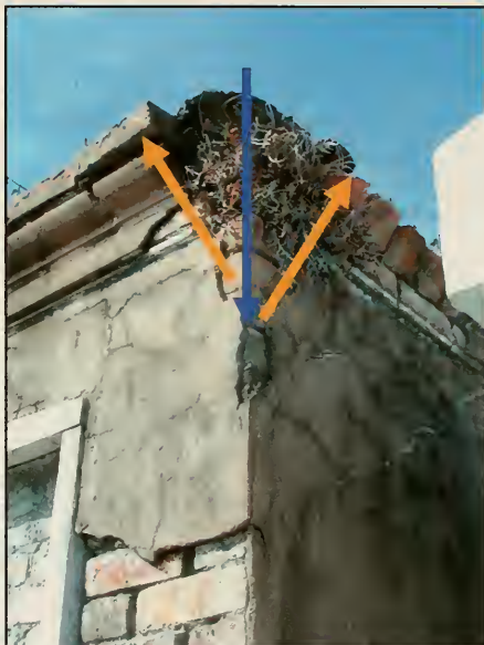
Fig. 4.11 Cornice failure.
