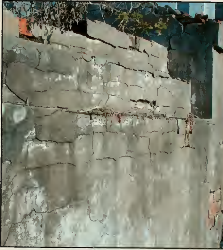
Fig. 4.5 Telescoping brick wall.
