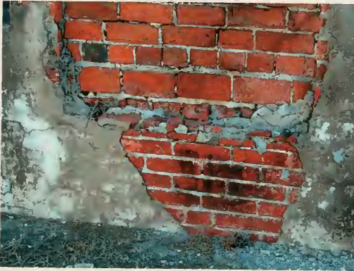
Fig. 3.3 Apparently, this pediment tomb was built over an earlier step or platform tomb. Note the different bricks used for each different period of construction.
