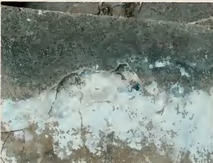
Fig. 6.23 Cement patch pushed off of original due to damaged material and salts.
