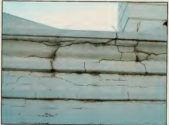
Fig. 4.7 Tomb #518 Sodiedad Cervantes de B.M. Restored in new cement.
