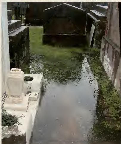
Fig. 3.6 Flooding between the tombs, Oct. 2001.
