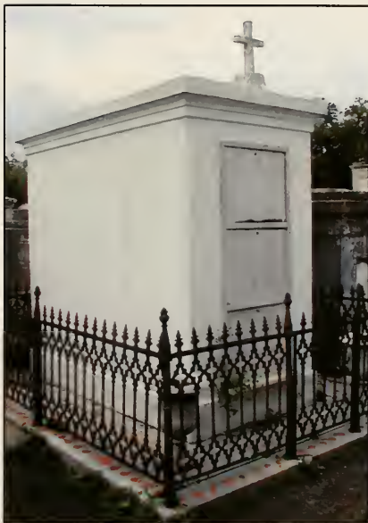
Fig. 6.12 The stucco skin on Tomb #230 has been well maintained. A modern finish coats the tomb, but has been applied over a well-prepared surface and shows no peeling or flaking. Some biological growth and higher vegetation is beginning to take hold and should be removed before problems start. A high integrity tomb on a marble precinct, surrounded by a path of grass. Studio photograph, March 2001.
