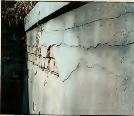
Fig. 6.25 The sides of a cement encased tomb beginning to break up.
