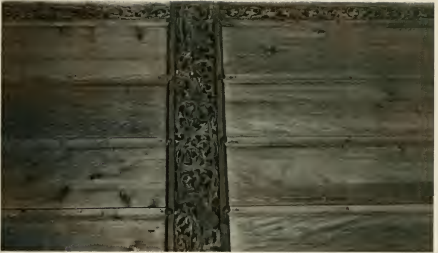
Figure E20. Swiss ceiling circa 1500 installed at the Swiss National Museum. Note the use of large, regularly spaced studs to affix batten and panelled ceiling to substrate. (See page 36.)
