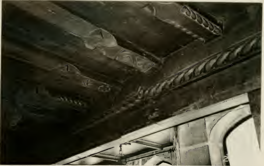
Figure E14. Swiss Room. Detail of the southern portion of the Tirolean ceiling. Note repetitive placement of a random series of carvings. (See page 35.)
