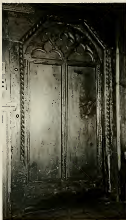
Figure E22. Swiss Room. Exit. Note trapezoidal shape of door surround and the rope molding detail which tapers off approximately 2' from the floor. (See page 37.)
