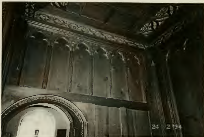
Figure D5. Monastic anteroom from Chur circa 1520. Note the coats of arms infilling the Gothic blind frieze. (See page 35.) Also note the use of blind friezes for both wall and ceiling construction. (See page 36.) Note the placement of moldings on the underside of the heavy timbers clearly visible from below. The ceiling is approximately 15' high. (See page 39.)
