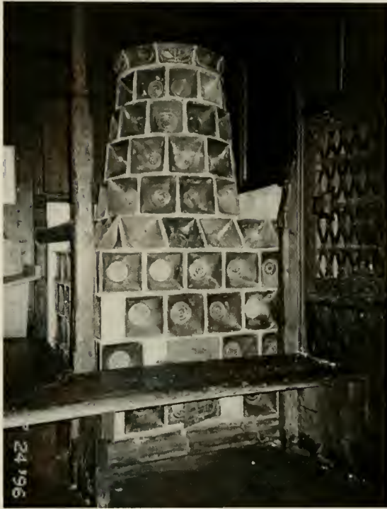
Figure E37. Swiss Room. Alpine stove in northeast corner of the Engadine portion looking north. Note square base and circular chimney. (See page 41.)
