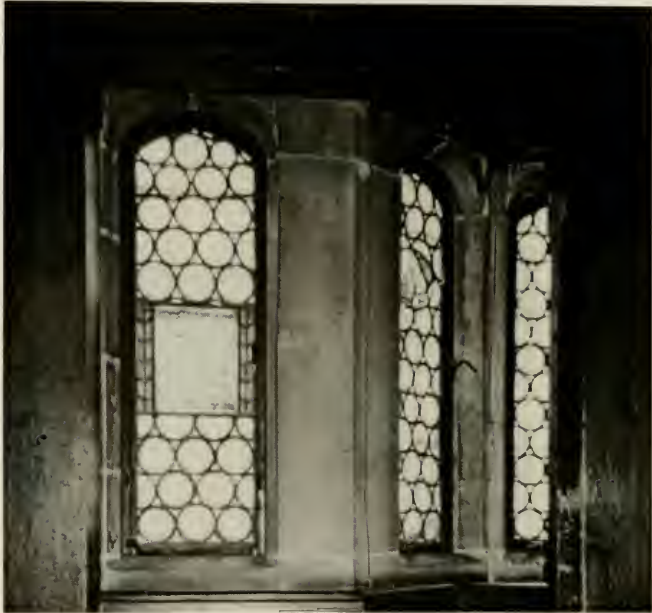
Figure E51. Swiss Room. East portion of the bay window stone surrounds. Note staining. (See page 61.)
