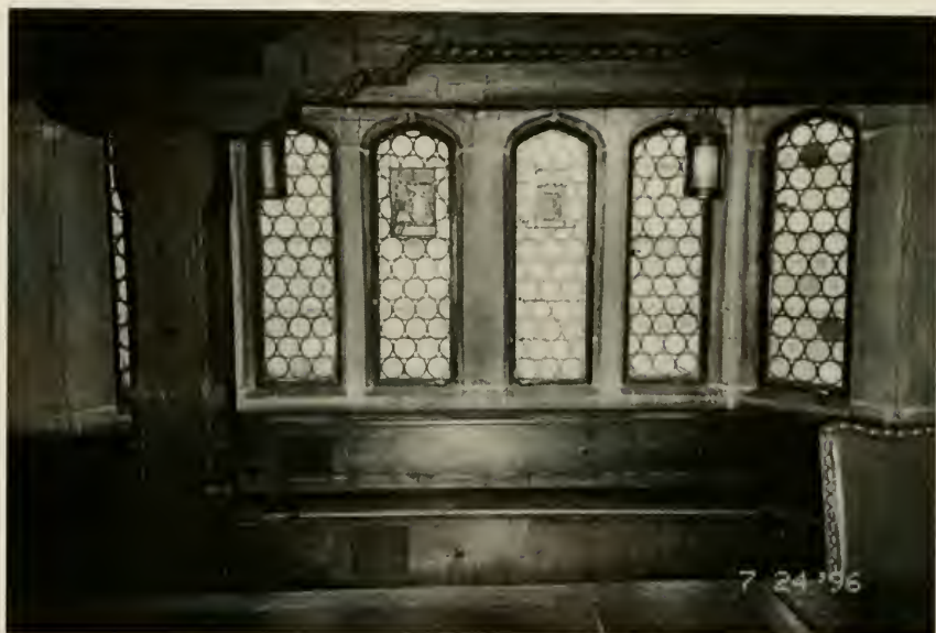
Figure E3. Swiss Room looking east at bay window comprised of old glass roundels and inset with glass panels. (See page 27.)
