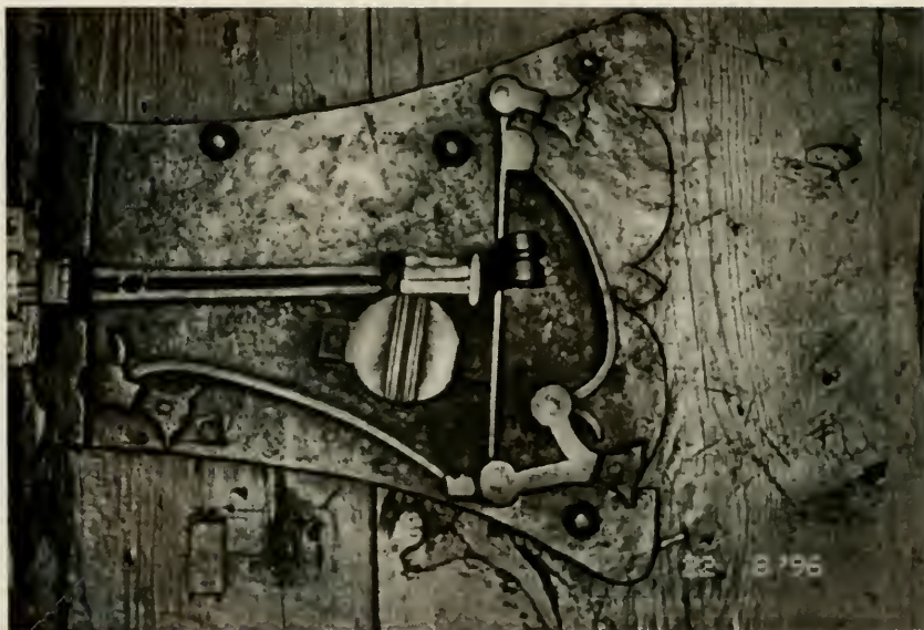
Figure E32. Swiss Room. Detail of lock on china closet door on the east wall of the Tirolean section. Note multiple generations of attachments. (See page 38.)
