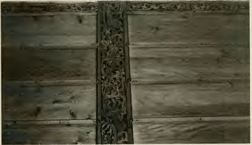
Figure E6. Swiss ceiling. Note the wider transverse molding and the thinner perimeter molding with related designs. (See page 32.)
