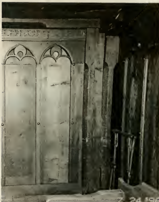
Figure E21. Swiss Room. West wall and northwest corner of the Tirolean section. Note how the blind frieze and panel construction meets at two corner posts of varying sizes while the ceiling springs from one small beam. (See page 37.)
