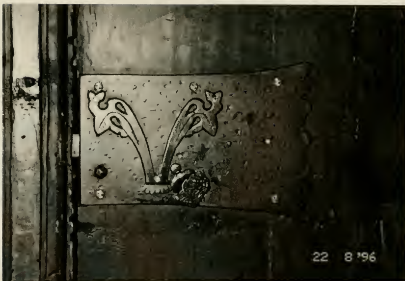
Figure E29. Swiss Room. Detail of latch and keyhole plate on the non-functioning door on the western section of the Engadine wall. Note multiple generations of attachments. Compare overall shape to Figure E30 and lock ornament to Figure E31. (See page 38.)
