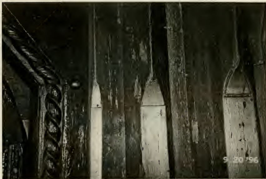
Figure E12. Swiss Room. Detail of the northeast corner of Tirolean section. Note variety of “ski” motifs carved into the corner posts. (See page 34.) Also note the significant amount of dirt on door surround to the left. (See page 56.)
