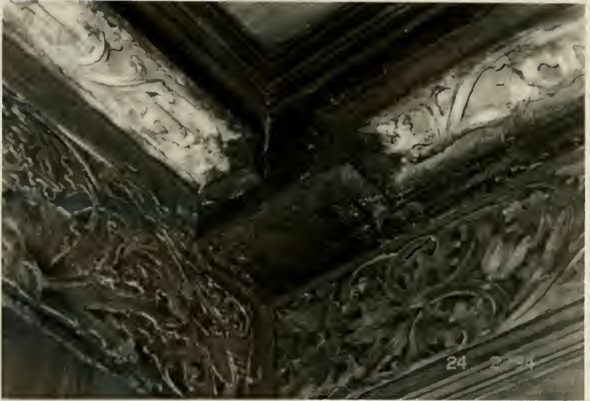
Figure E17. Corner detail of a room in the Fraumünster Abbey in Zurich circa 1490. Note the multiple decorative elements on distinct planes meeting flush at the corner. (See page 35.)
