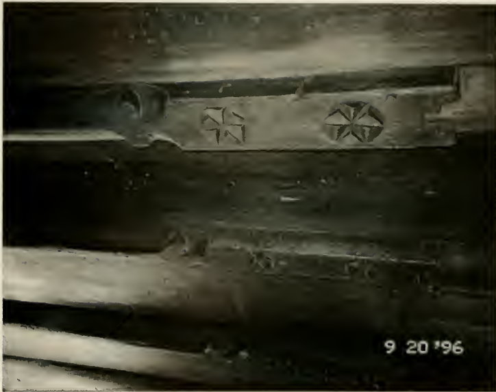
Figure E10. Swiss Room. Detail of Tirolean ceiling. Note rosettes carved into joists. Compare with Figure E11. (See page 33.)
