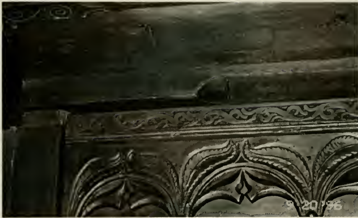
Figure E4. Swiss Room. Detail of the east Tirolean wall. Note the inappropriately placed molding overlaying the blind frieze. (See page 32.)
