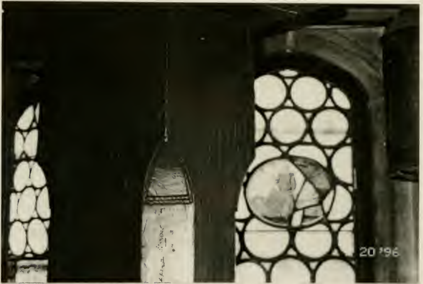
Figure E2. Swiss Room. Detail of 1930s column carved to match original motifs and stained with a red aniline dye used in the Berkeley Dining Hall. (See page 26.)
