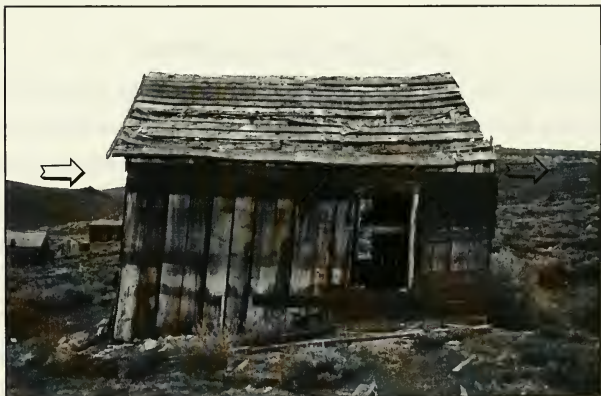
Figures 3.8a & 3.8b. Diagram of load induced by wind. Photograph of result of shear stresses on Owen. South Elevation taken 21 May, 1997 by P.D. Schulz.
