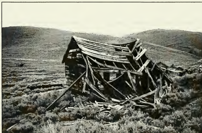
Figure 3.10a. Diagram of buckling and wall collapse (combination of loads) Figure 3.10b. Photograph of wall collapse. South-East elevation Building "N" taken 13 June, 1996 by Lee Motz.
