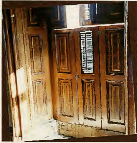
Fig. 7. Second floor interior shutters at the Lockwood-Mathews Mansion folded into recesses when opened. Louvred panels provide ventilation.
