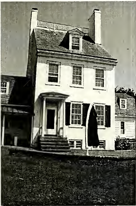
Figure 7 View of 1837 Addition from the South
