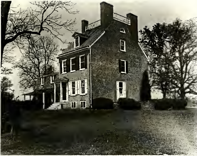
Figure 7 View from the Southeast, 1935. VF - Cecil County - Houses (Cecilton) Rose Hill Façade 3, c.1935 The Maryland Historical Society, Baltimore, Maryland
