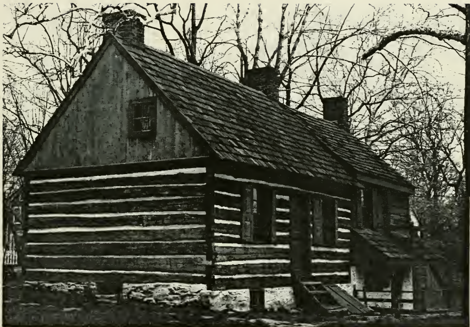
Fallsington - Moon-Williamson Log House, front facade
