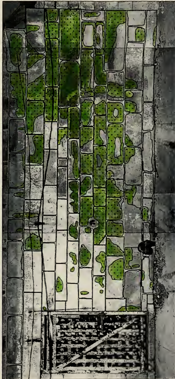
Figure 9: Salt Efflorescence
