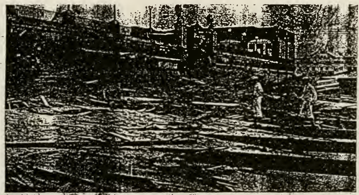
What's left of Asbury Park Boardwalk in front of Casco. Debris is piled up in front of Solarem.
