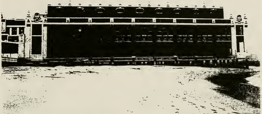
Ill. 66. South elevation of Convention Hall/Paramount Theater Arena, 1996.
