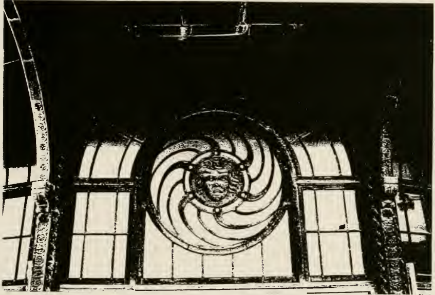
Ill. 74. Copper window detail on Carousel Pavilion, 1996.
