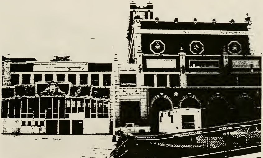
Ill. 63. Section of north elevation of Convention Hall/Paramount Theater showing water tower (slated for restoration under 1996 New Jersey Historic Trust Grant), 1996.
