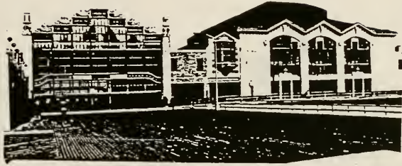
Casino, view North (from boardwalk)
