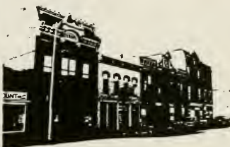
above: The Union Avenue Commercial District in Pueblo, Colorado, is one of the most common types of historic places in a community downtown central business district. — Jim Moore
