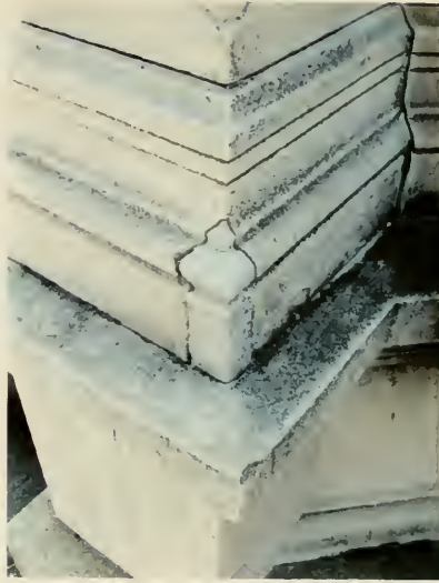
Figure 29: Dutchman repair in pedestal (Photograph by author, March 2002)
