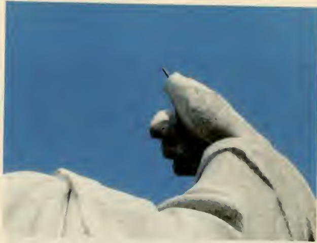
Figure 21: Exposed metal pin from previous repairs to the hand of Moses
