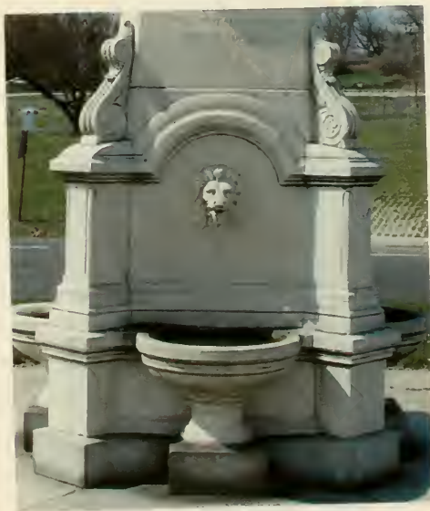
Figure 34: Stain on pedestal under lion head spout (Photograph by author, March 2002)
