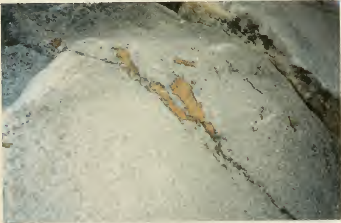
Figure 20: Inclusions in marble blocks of the rock mound base
