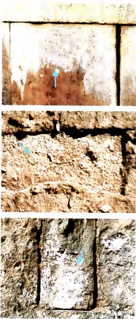
Fig. III.1 (Top) Thin salt crust on Comité replacement stone; (middle) salt veil and (bottom) salt bloom on Ayyubid stone. From AKTC, 2001.
