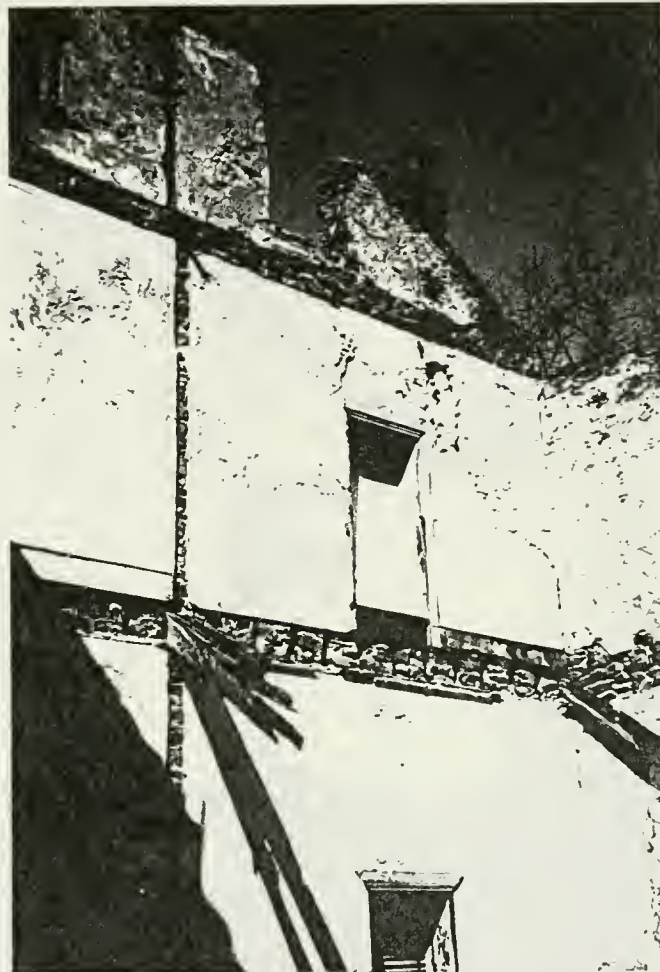
Figure 20: North interior elevation of the Wetherill addition, showing two remnants of beams and finished attic
