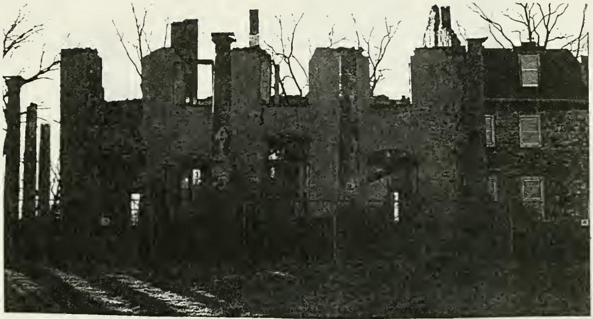
Figure 4: Eastern Elevation of the Pawling/Wetherill House
