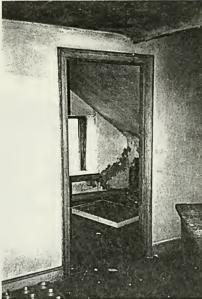
Figure 18: Third story finished attic space of the Pawling section
