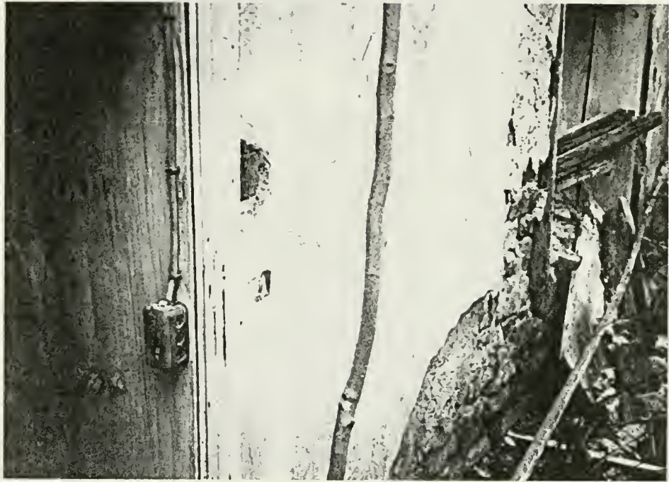
Figure 22: Basement Level lighting fixture and children's drawings on plaster
