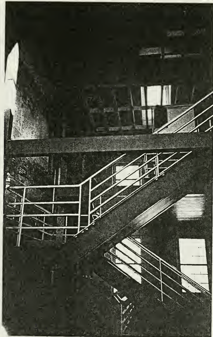
Figure 41: Franklin Court, "Fragments" Section, Modern vertical circulation.
