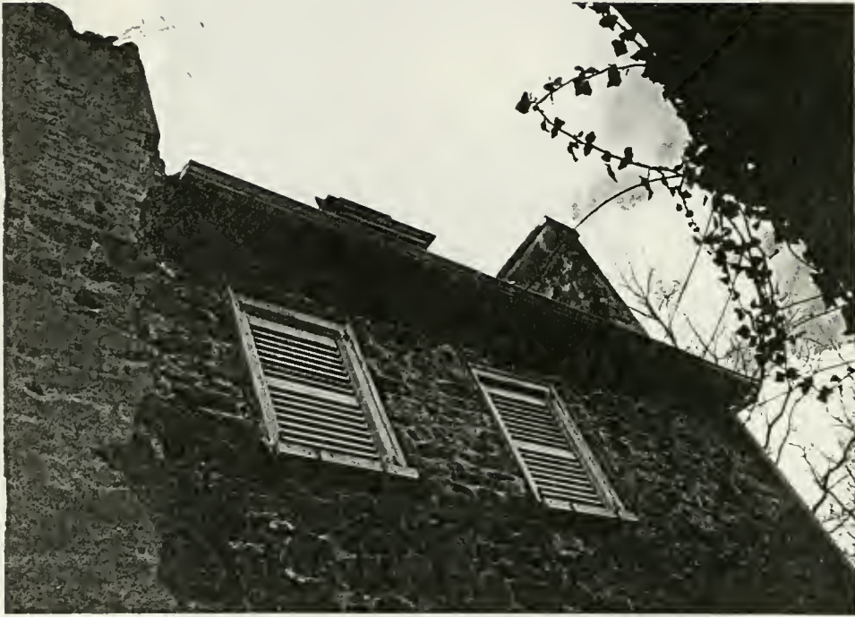
Figure 16: Exterior of the Pawling section, east elevation
