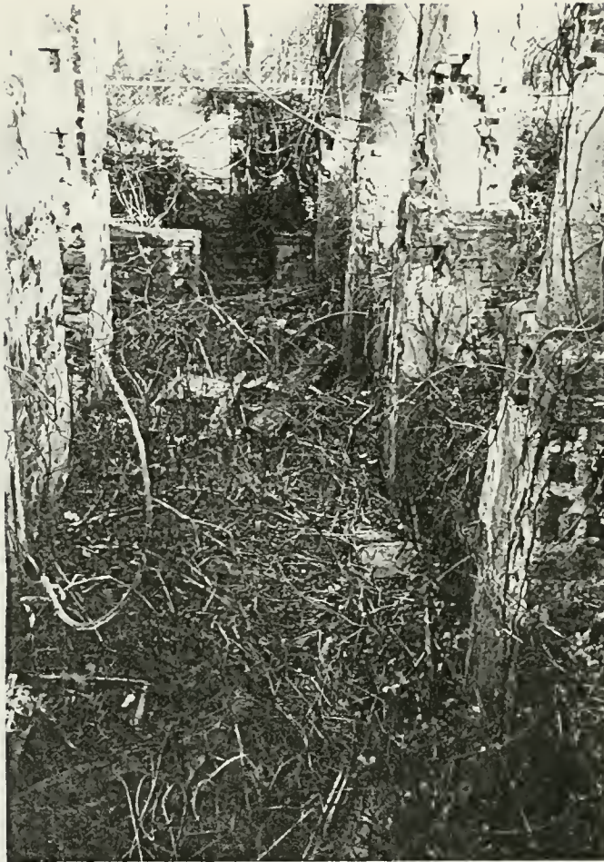
Figure 39: Ground level of south porch
