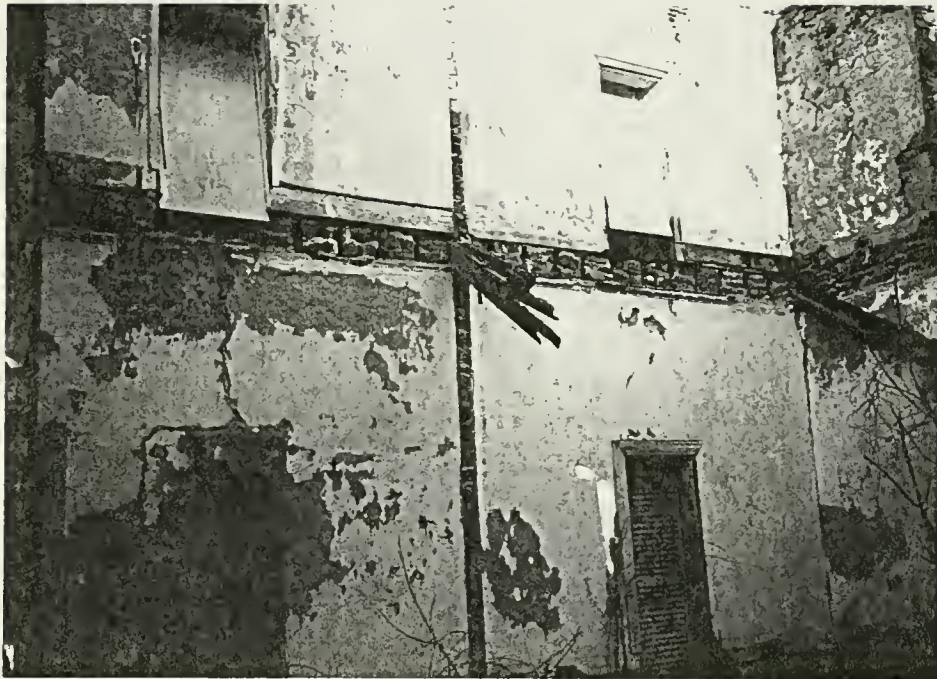
Figure 35: Northern interior wall of addition (connected to Pawling portion of house)
