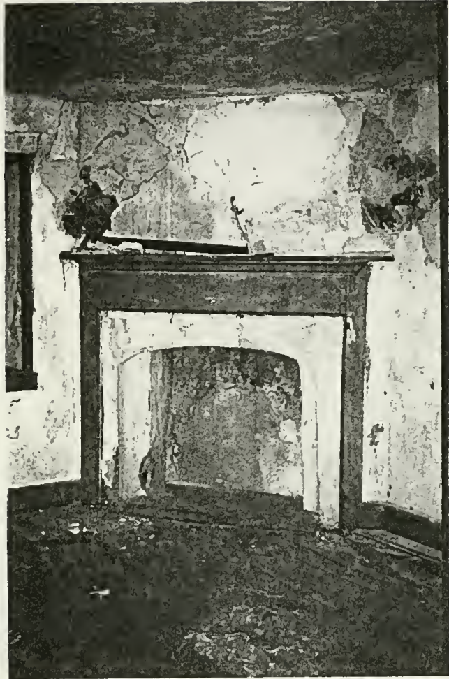
Figure 17: Second story corner fireplace of the Pawling section
