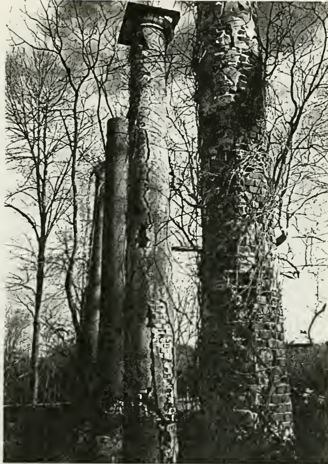
Figure 38: View of columns showing overgrowth of vines
