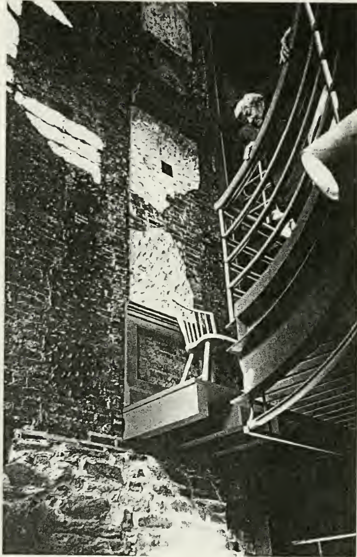
Figure 42: Display of architectural fabric at Franklin Court
