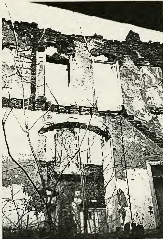
Figure 26: Interior masonry wall of addition
