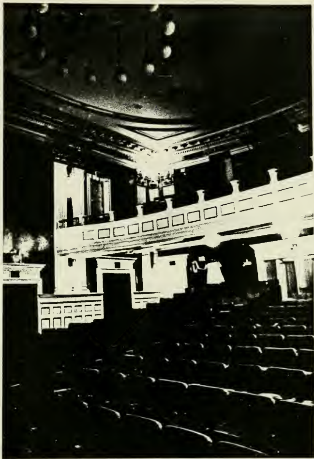
Figure 24 Auditorium looking from stage toward balcony Photo: David Harrington, 1985
