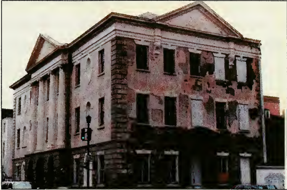
Figure 3.4. Charleston County Courthouse (under restoration).
