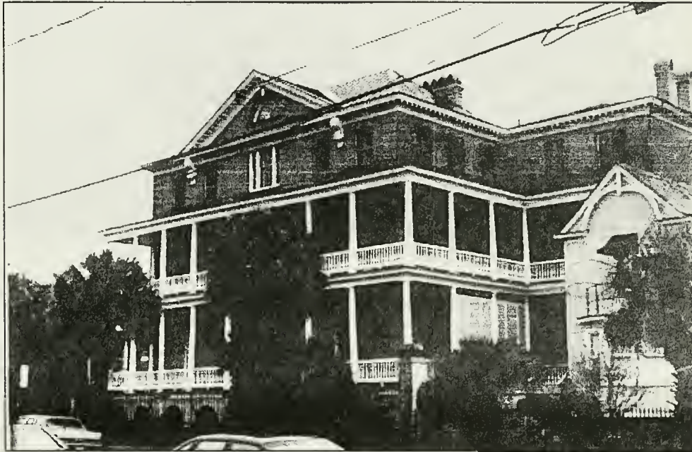
Figure 4.5. Stucco applied to the building in the 1830s was, in part, represents an aesthetic intention of providing unified, updated appearance to parts of the building which had been altered. View from southeast.
