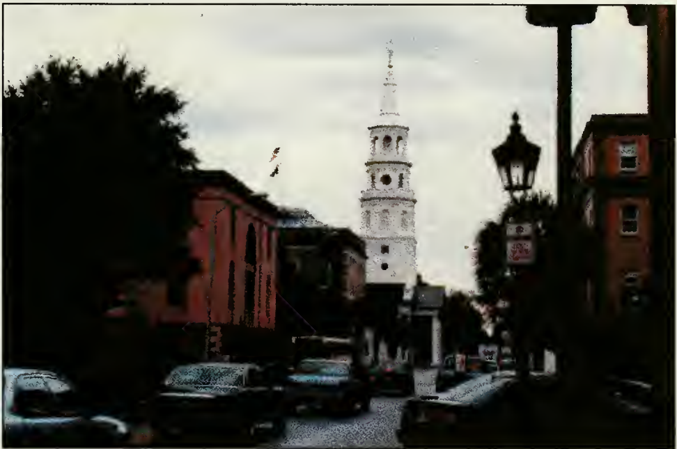
Figure 3.2. Stuccoed facades on Meeting Street, Charleston.
