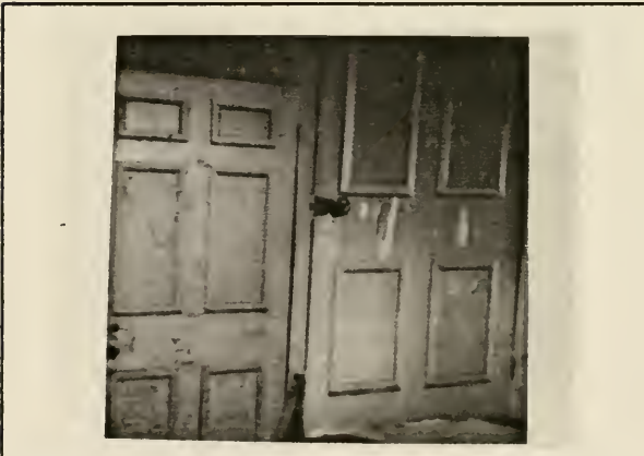
456-458 Belgrade Street, ca. 1783, Interior.
