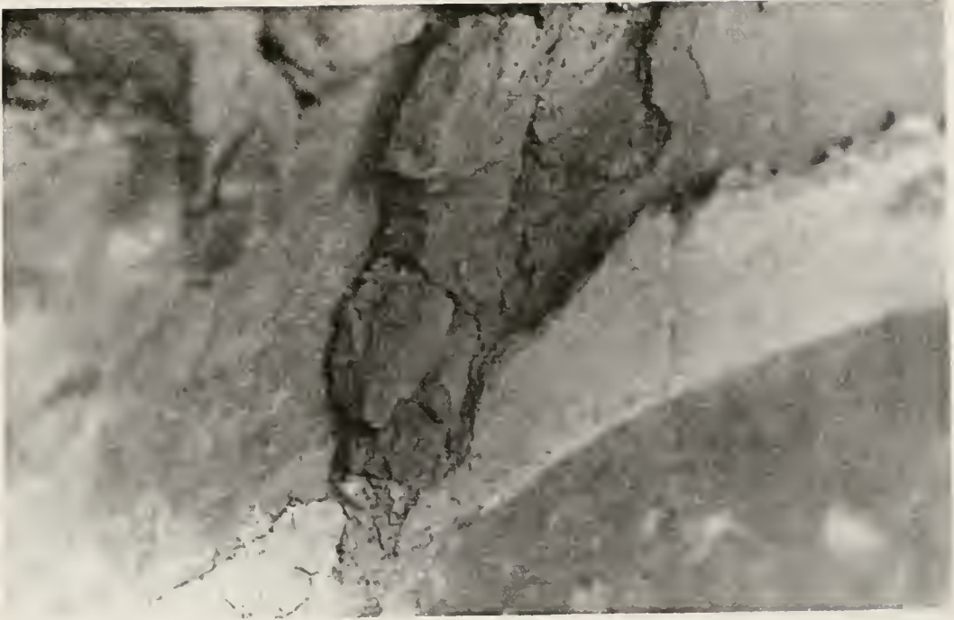
Fig. 21 Detail of Base Coat Plaster in Kiva C
