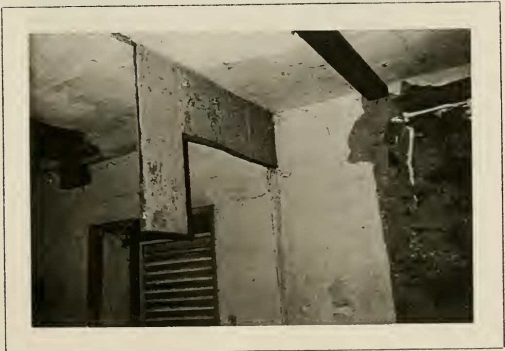
Plate 60: Detail of 19th century beaded-board partition at west wall of Rm.202, 1991.
