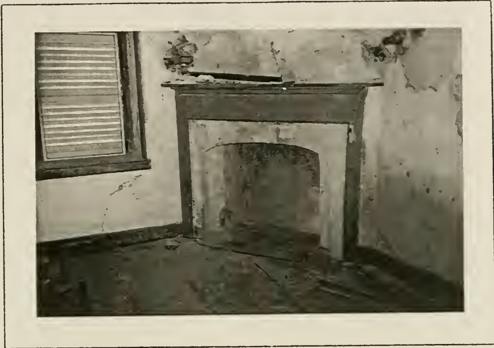
Plate 49: Detail of corner fireplace in Rm.201, 1991. Mantel is 19th century addition.
