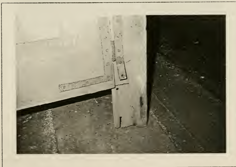
Plate 48: Detail of lower hinge on cupboard from Rm.102, 1991.
