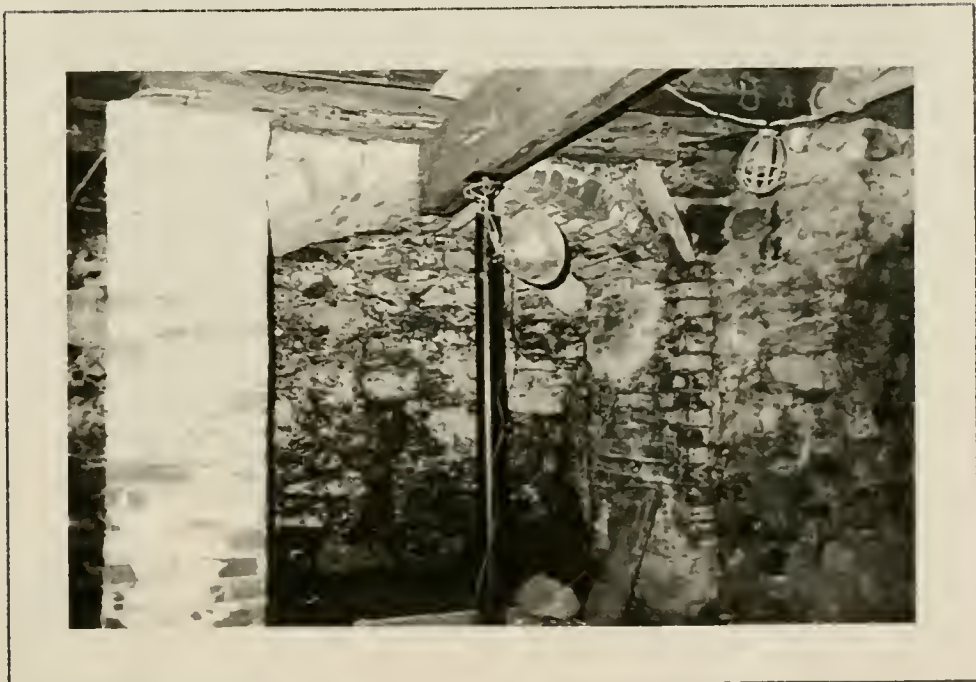
Plate 32: Detail of brick arch supporting late 19th century hearth in Rm.102, 1991.
