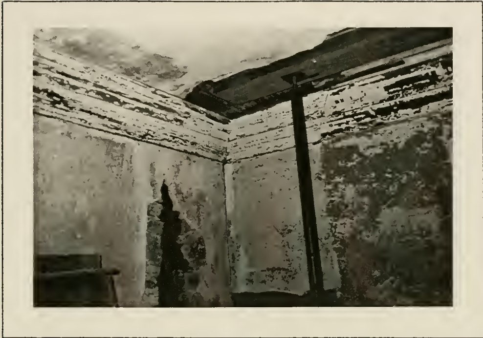
Plate 38: General view of location of corner cupboard in Rm.101, 1991.
