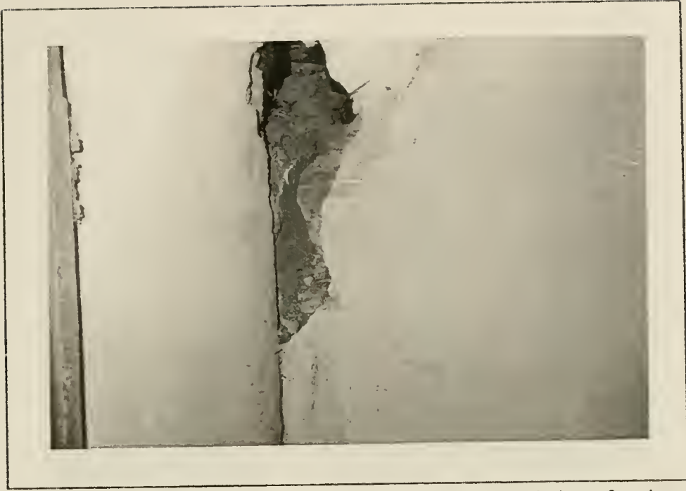
Plate 51: Detail of 18th century finish plaster continuing behind 19th century masonry, Rm.201.
