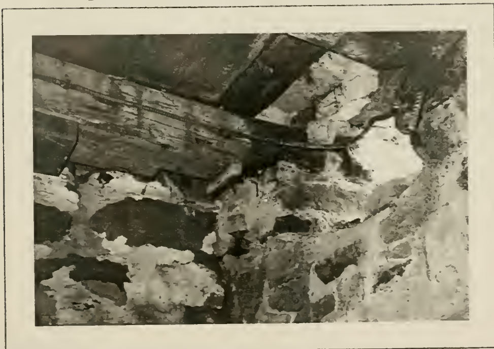
Plate 28: Detail of first floor joist bearing in 18th century south wall of cellar, 1991.
