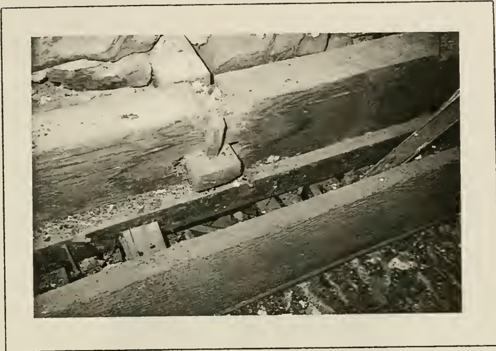
Plate 18: Detail of interior mortised connection of door hood supports, 1991.
