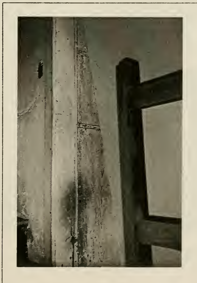
Plate 66: Detail of door opening onto stair through south wall.
