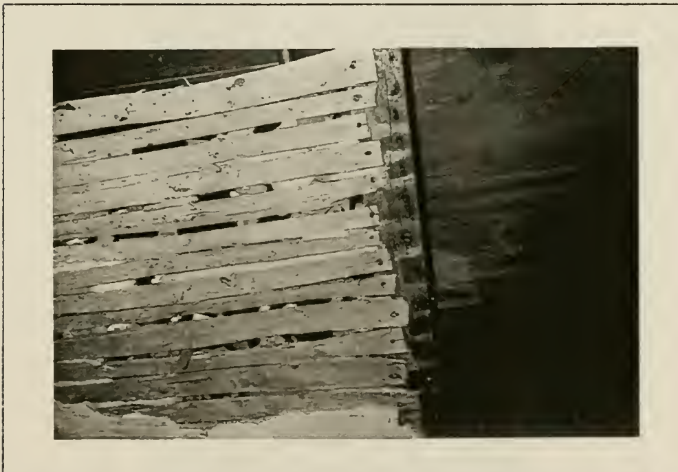
Plate 43: Detail of ceiling of Rm.102, 1991. Note handsplit oak lath with wrought nails, renailed with cut nails, covered with 19th century plaster.
