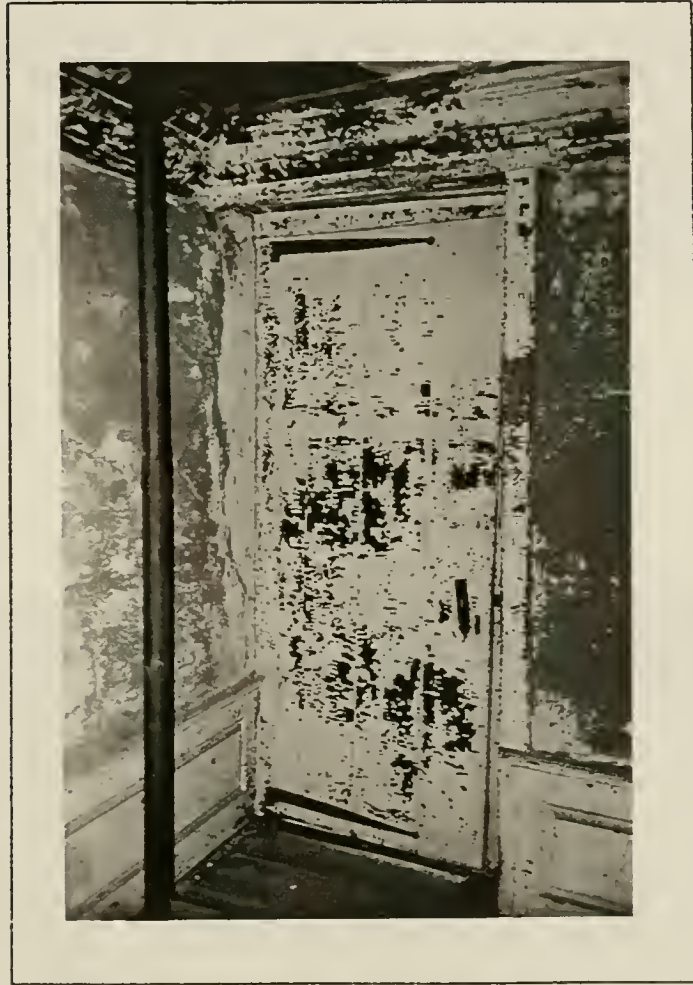
Plate 22: Interior elevation of 18th century door and frame, 1991.
