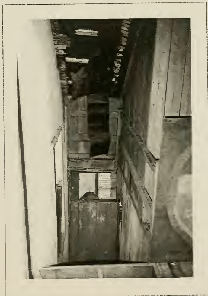
Plate 64: View down stairway from attic, 1991. Note 1836 railing.
