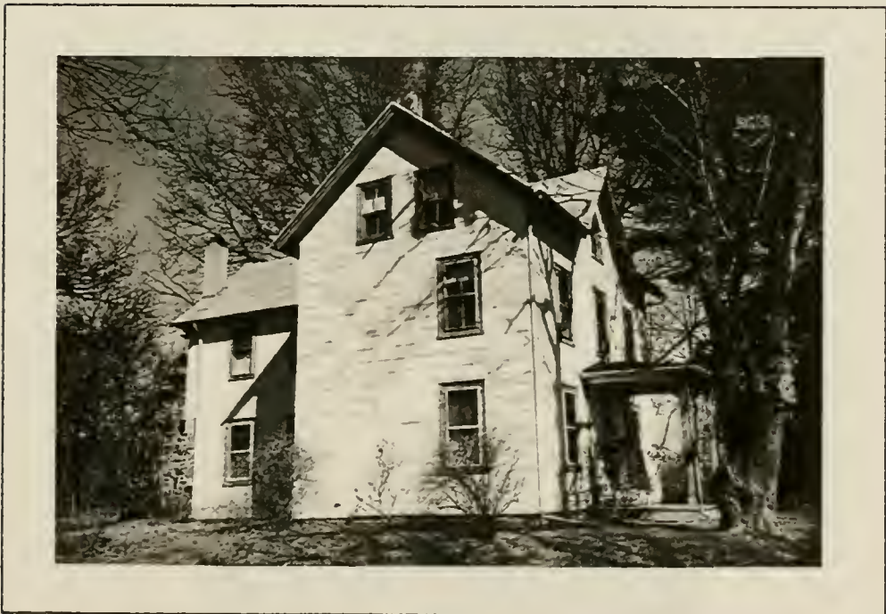
Plate 72: View of late 19th century tenant farmer's house at Walnut Hill, 1991.
