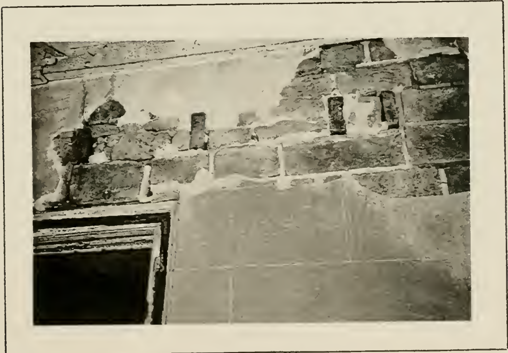
Plate 17: Detail of supports for cantilevered door hood on north facade, 1991.
