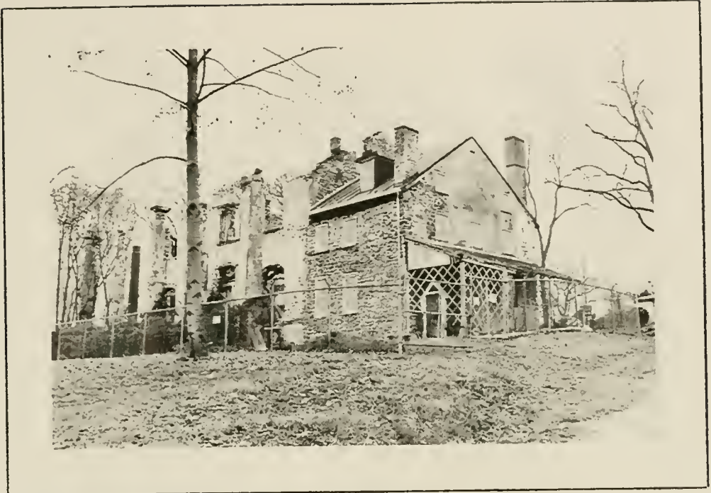
Plate 12: View from northeast, 1991.
