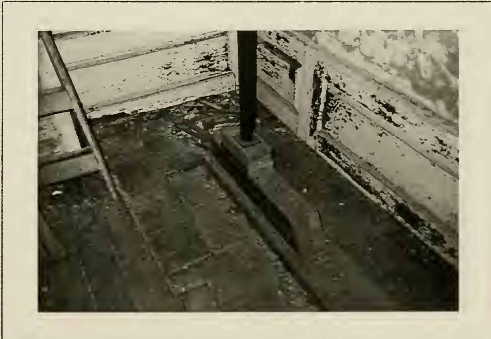
Plate 39: Detail of panelling at location of corner cupboard in Rm.101, 1991. Original dado panelling at right, 19th century infill at left.
