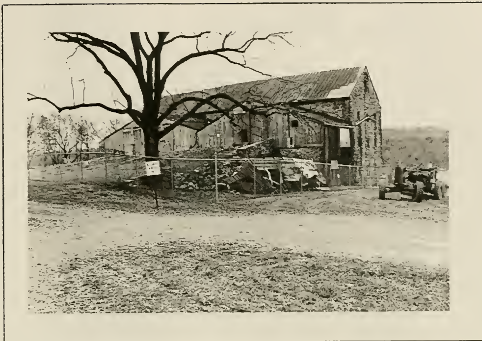
Plate 69: General view of Wetherill barn at Walnut Hill, 1991.
