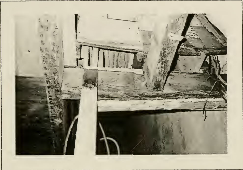
Plate 55: Detail from below of second floor framing around stair opening, 1991. All 3x8 joists and headers appear original and in original locations.
