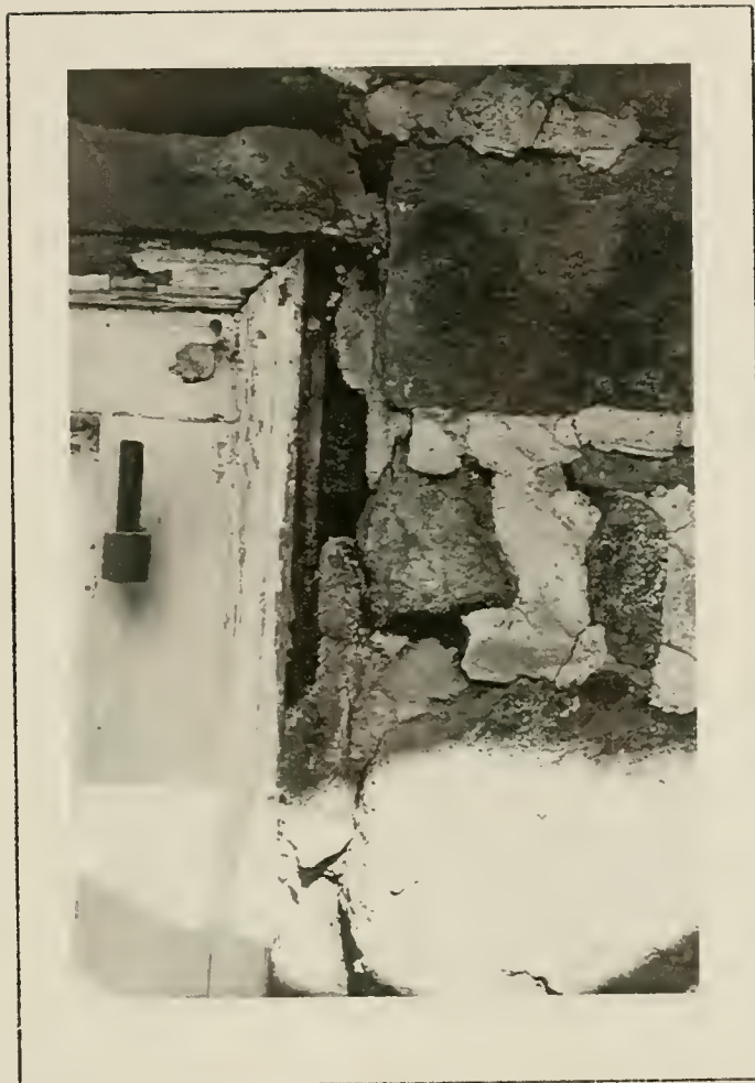
Plate 25: Detail of replacement window frame, first floor west.
