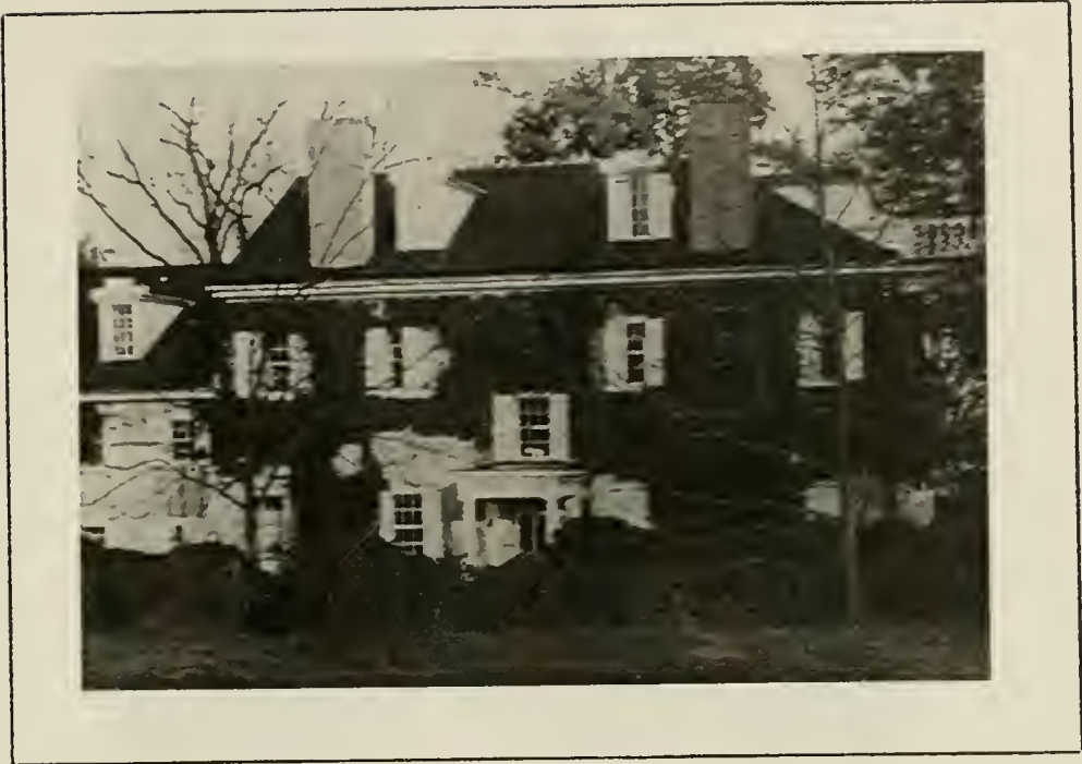
Plate 3: View of rear of house from west, circa 1955.
