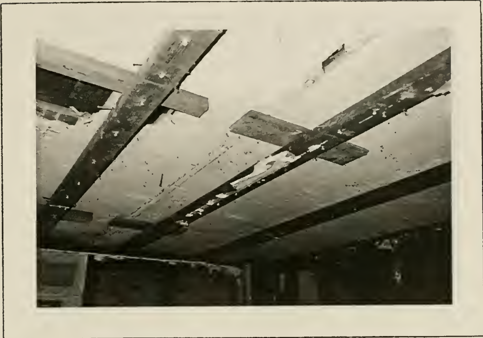
Plate 61: Detail of 19th century ceiling in Rm. 202, 1991. Note presence of beaded-board partition, installed with plaster ceiling and later removed.
