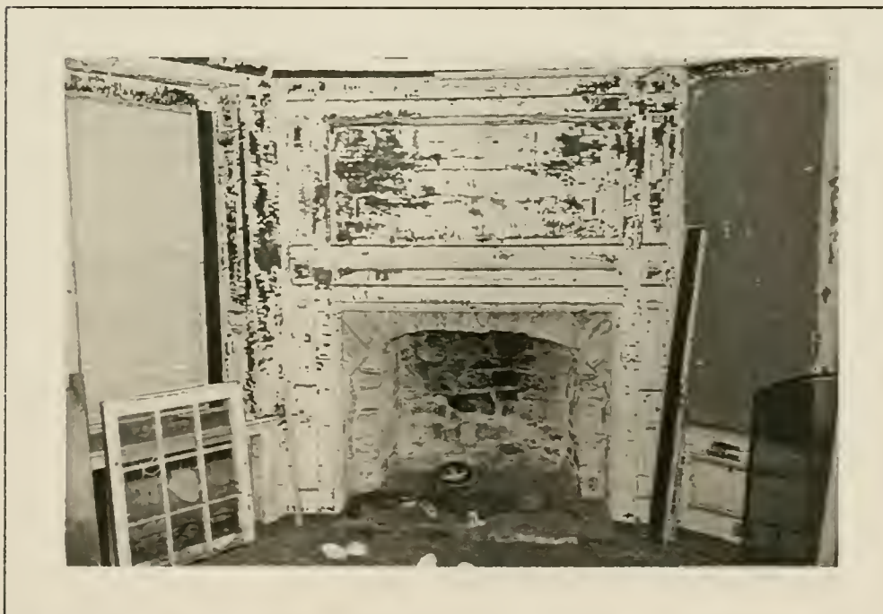
Plate 34: Detail of corner fireplace in Rm. 101, 1991.
