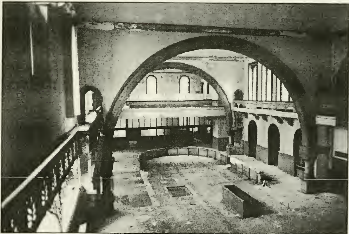
Figure 111. East view from Northwest corner of mezzanine, November 2000 photograph.
