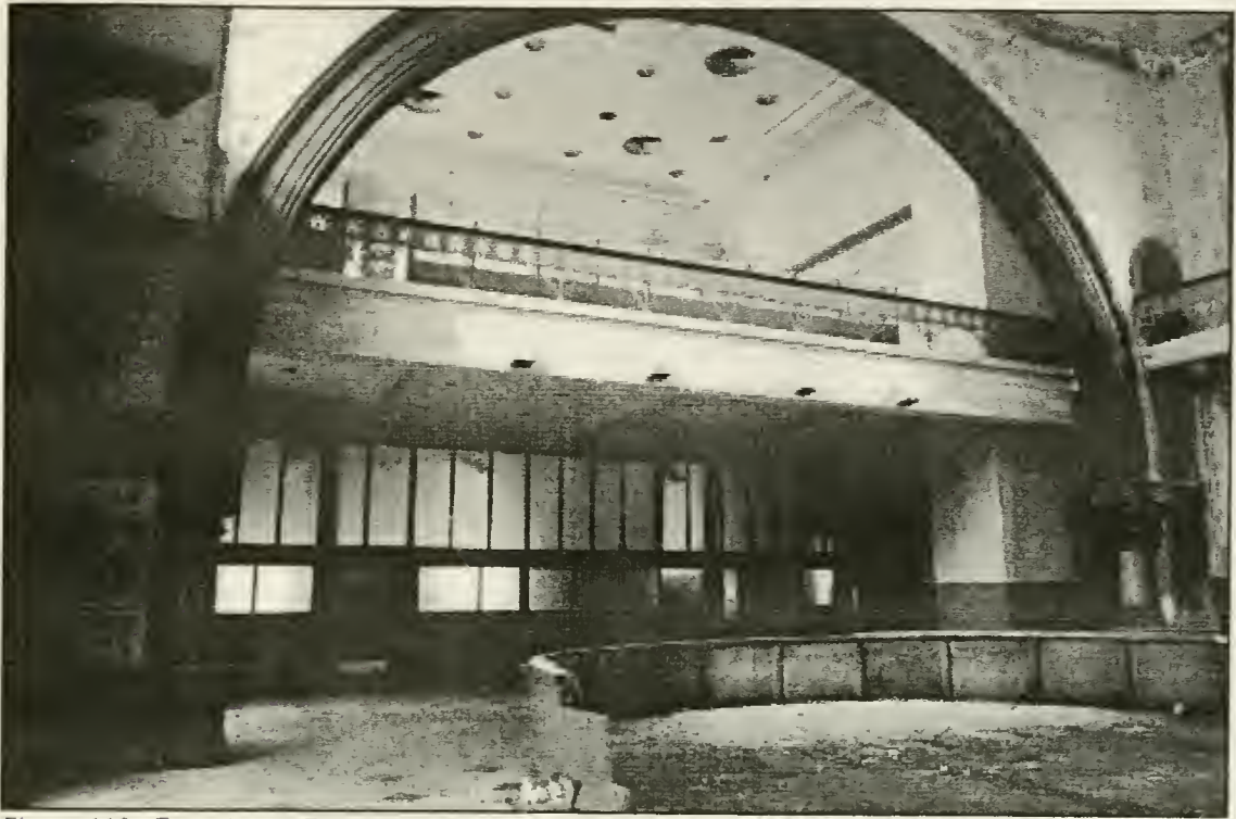
Figure 110. East view to East mezzanine, November 2000 photograph.
