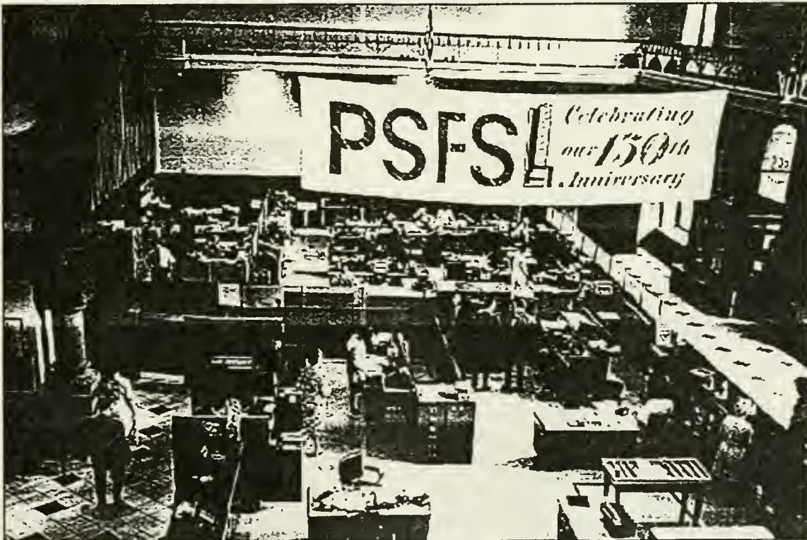
Figure 69. West view of banking room floor, 24 June 1966 photograph.
