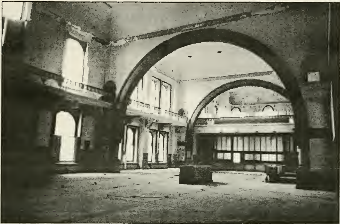
Figure 114. View East from West wall, November 2000 photograph.
