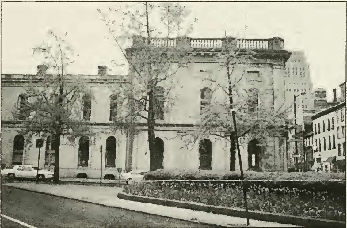
Figure 99 East façade, North section, April 2000 photograph.
