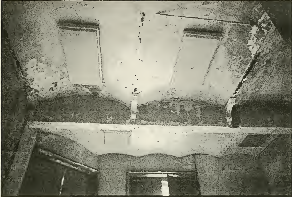
Figure 124. Arch ceiling construction in East wing, November 2000 photograph.
