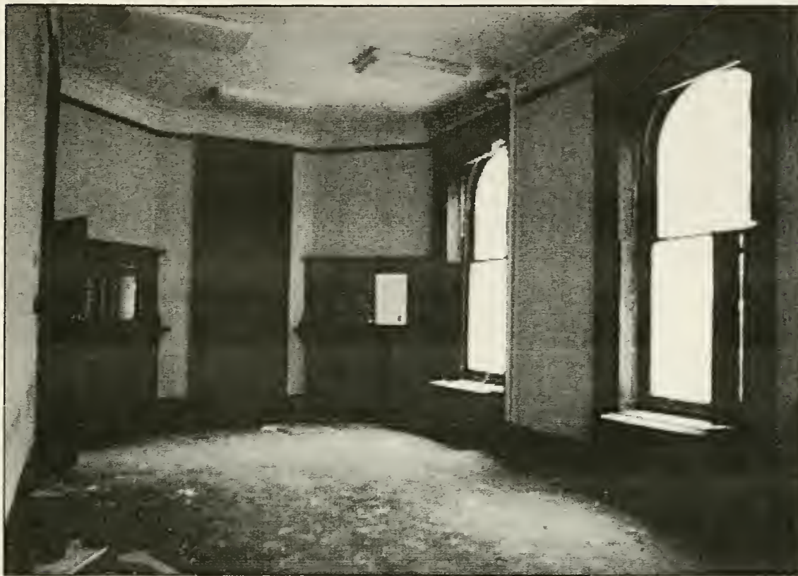
Figure 106 East wing, first floor interior, November 2000 photograph.
