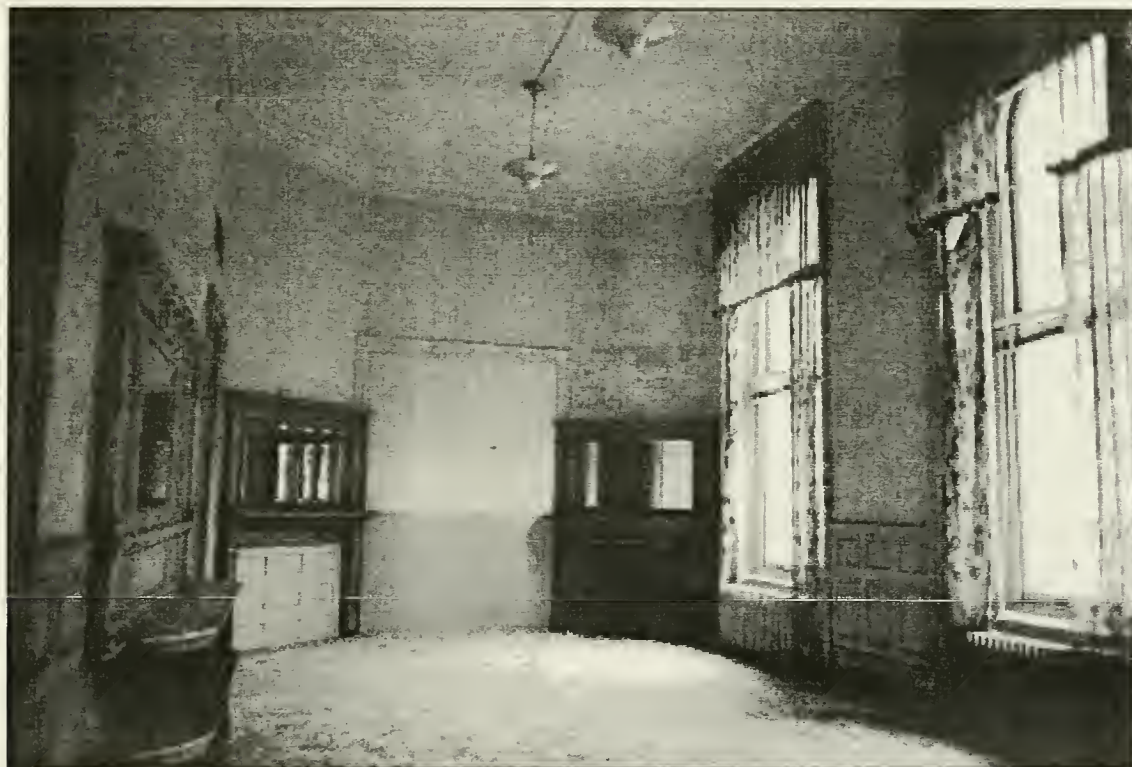
Figure 105 East wing, second floor interior, November 2000 photograph.
