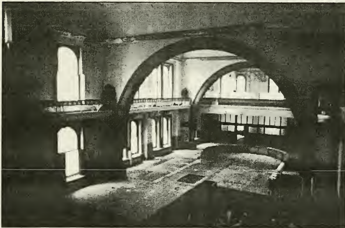
Figure 113. View East from West mezzanine, November 2000 photograph.
