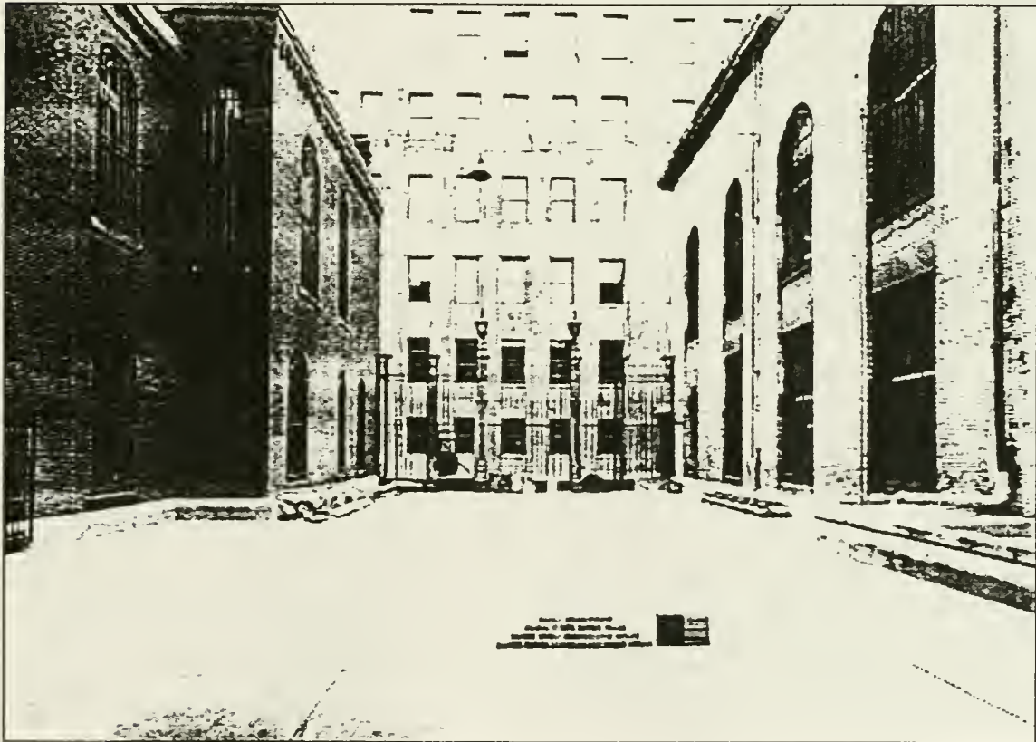
Figure 87. South view of completed courtyard, paved, 18 May 1931 photograph.
