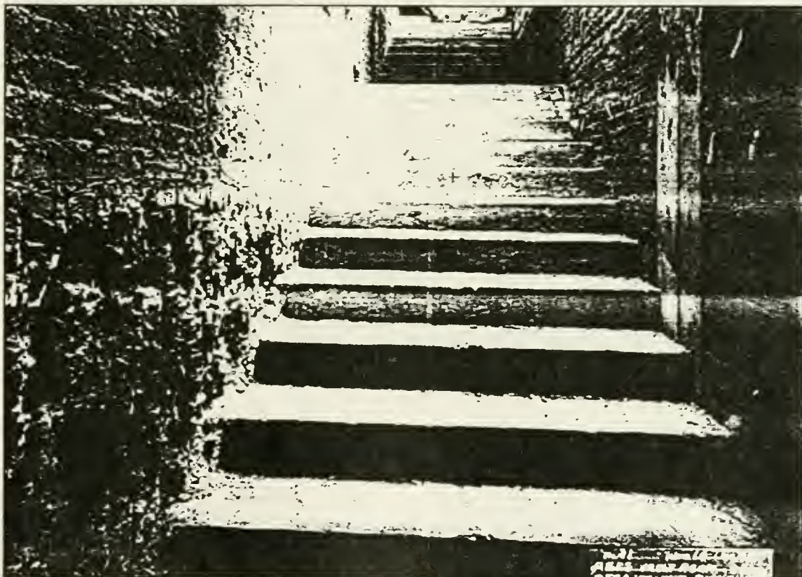
Figure 85. Vault room stairwell, 14 October 1930 photograph.
