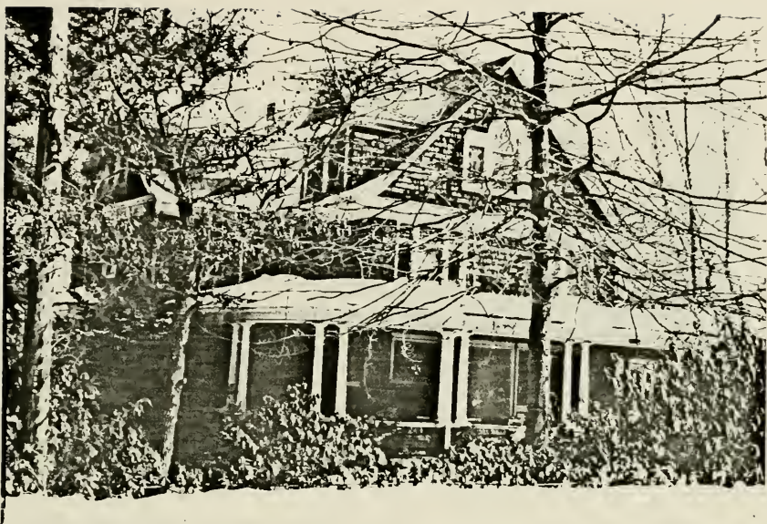
31. Fitch Cottage, Eagles Mere Avenue, facing North (1993 Photograph).
