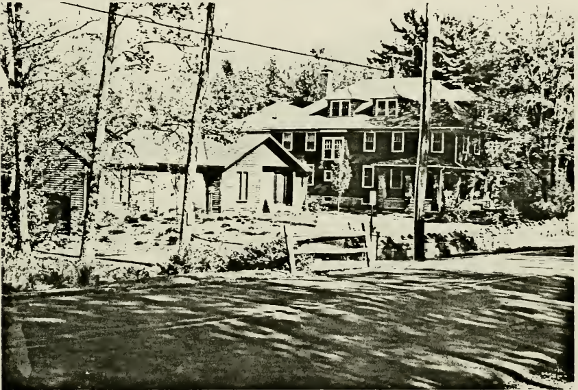
14. (P9) Pennsylvania Avenue, facing Southeast, showing modern cottage in foreground (1990); Madeley Cottage, "Sunnyside", on right (1912). The construction of the 1990 cottage was the catalyst behind the creation of the Eagles Mere Historic Preservation Committee.
