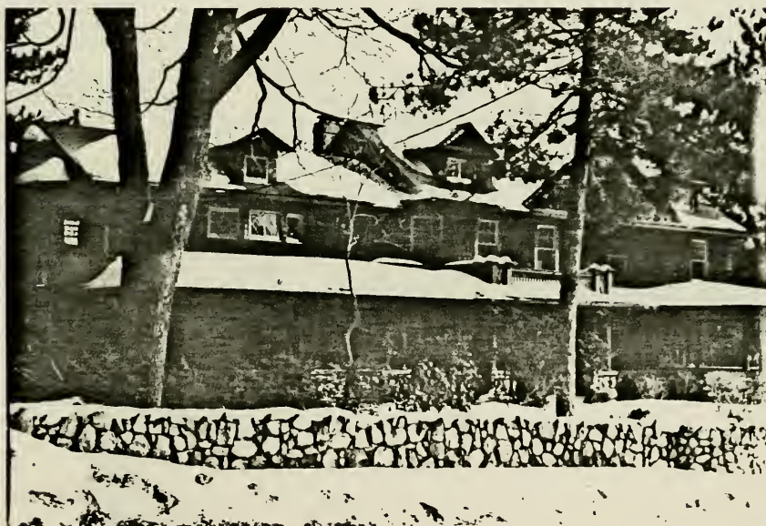
34. Ryan Cottage, Eagles Mere Avenue, facing North (1885, rebuilt 1888).
