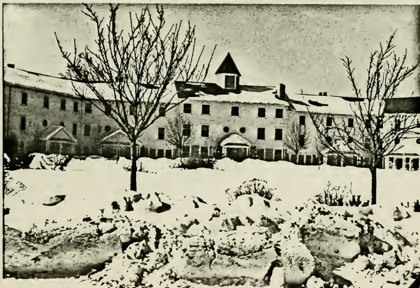
20. Crestmont Condominiums, facing South, (1984).
