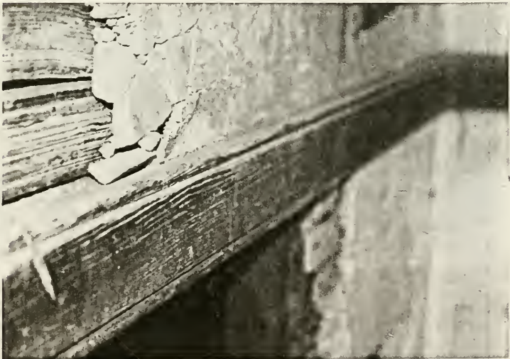
Detail of Chair Rail in Georgian South Chamber
