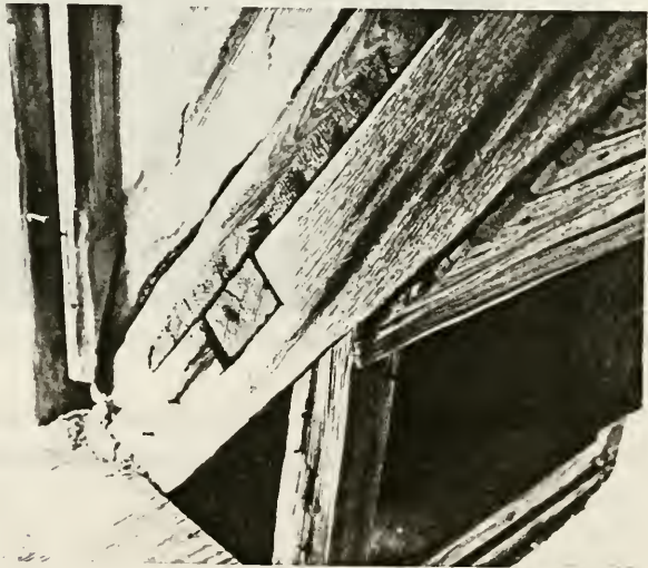
Figure 79: Wind Brace in Georgian Dormer Frame
