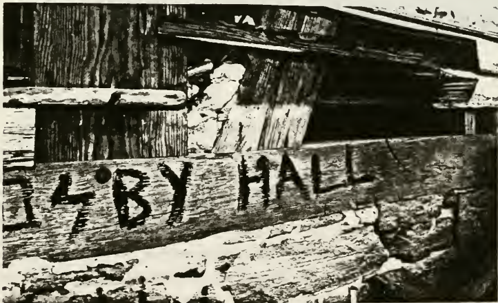
Figure 16: Federal Section Post and Brace Near Main Door
