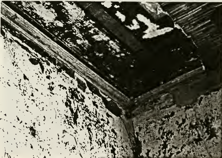
Figure 55: Paint Finishes in Federal East Parlor
