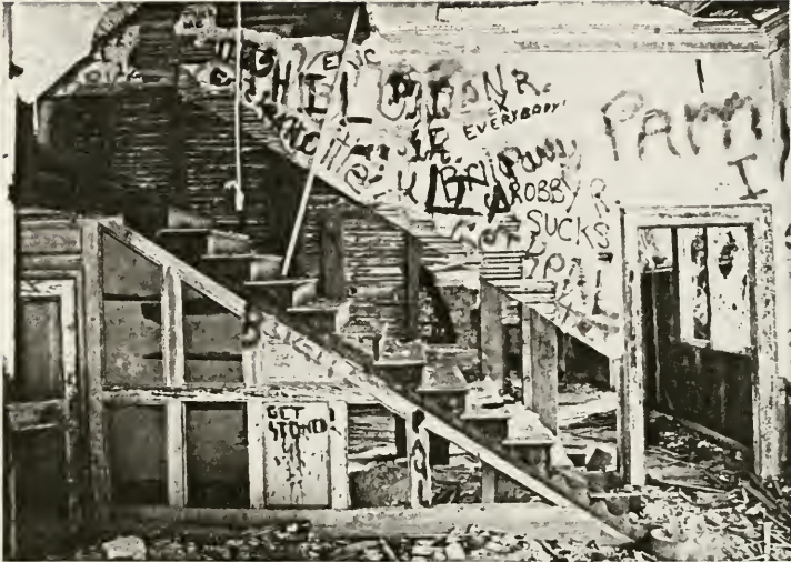
View of Federal Cross Hall Stairs
