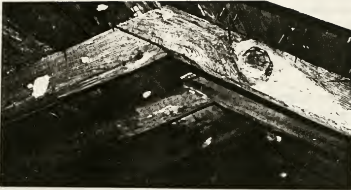
Figure 37: Federal Main Portico Roof Rafters
