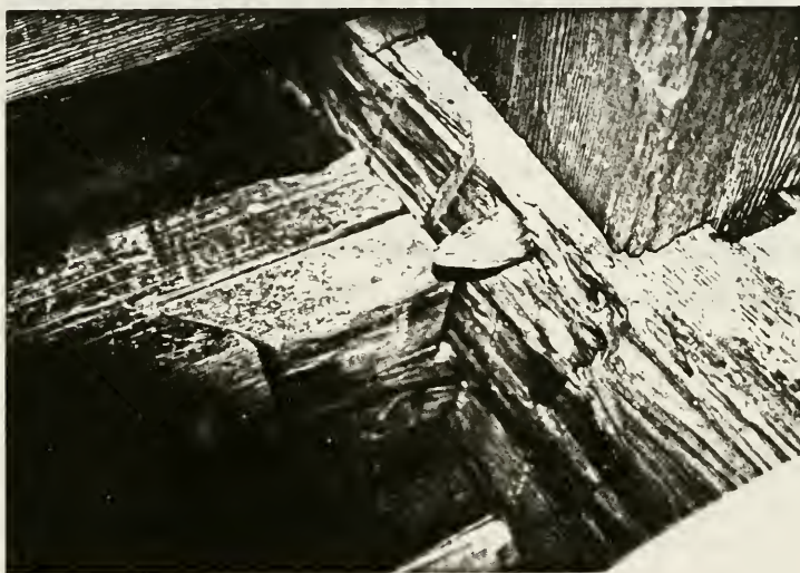
Figure 33: Joinery at the Base of the Federal Section Gable Center Post
