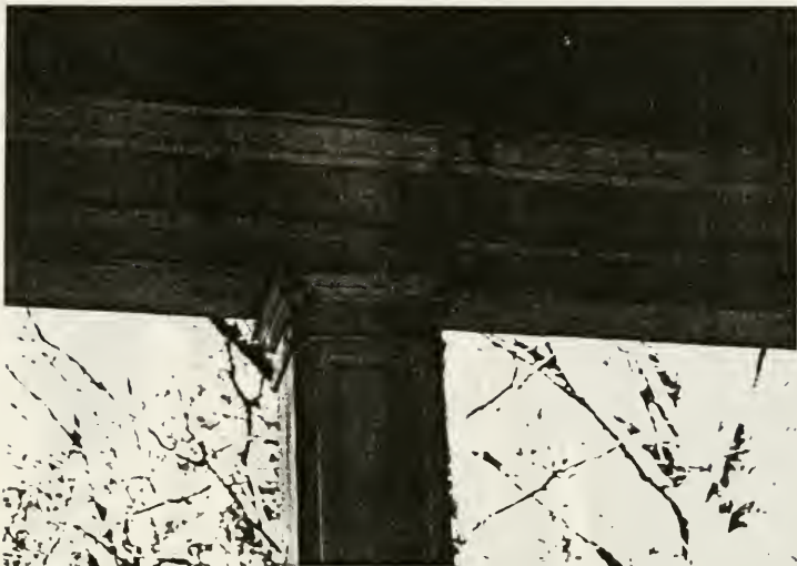
Figure 49: Detail of Main Portico Pier
