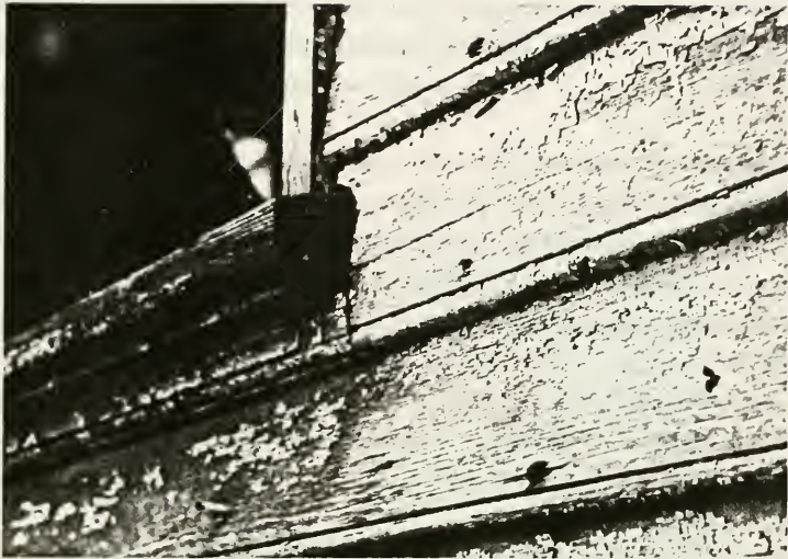
Figure 44: Federal West Parlor South Window and Siding
