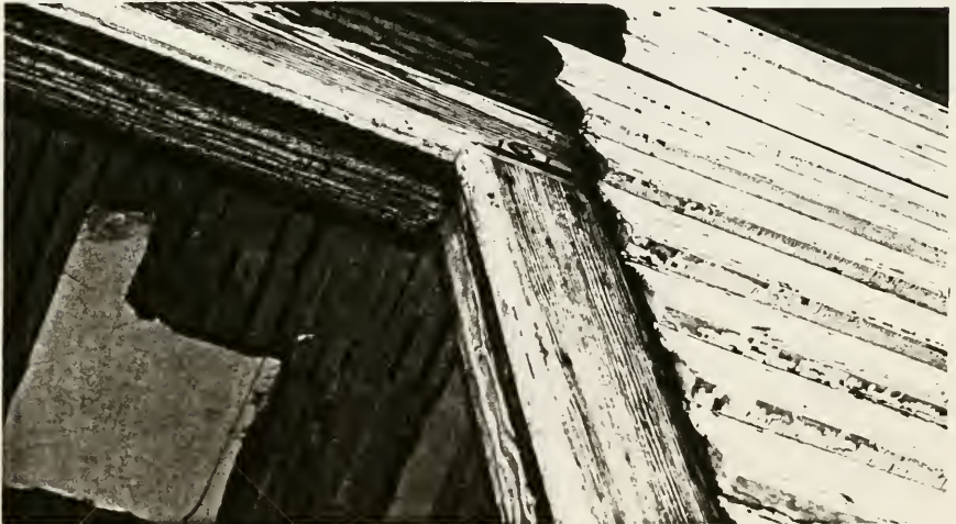
Figure 25: Federal Section First Floor Window Frame
