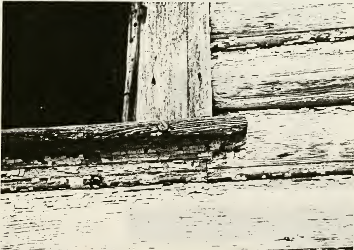
Figure 45: Georgian West Parlor Window and Weatherboard
