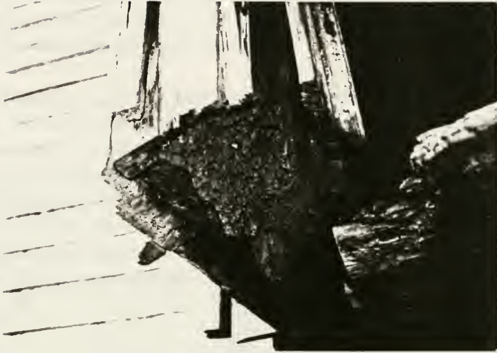
Figure 24: Federal Cross Hall East Door Jamb
