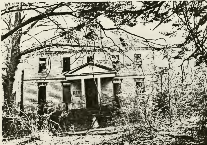
Figure 87: North Elevation Damage
