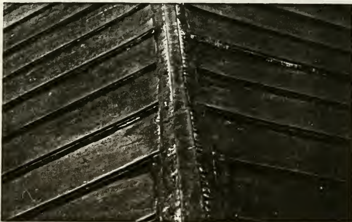
Figure 52: Main Portico Standing Seam Roof
