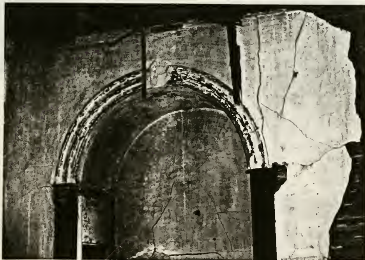
Figure 57: Arch Detail of Recess in Federal West Parlor
