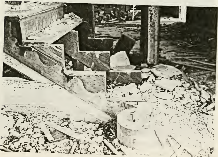
Detail of Federal Cross Hall Stairs
