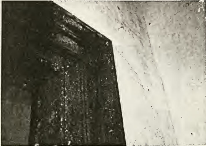
Figure 66: Door Architrave of Georgian Hall
