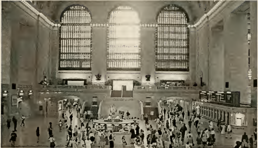
Figure 27 Present Main Concourse looking East Staircase
