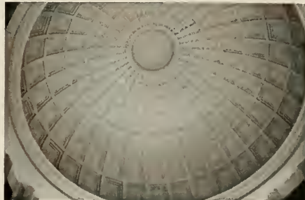
Figure 60 Present ceiling Photo taken by the author
