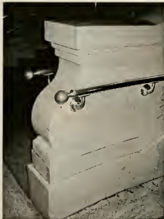
Figure 29 Modern East Staircase
