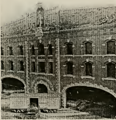
Figure 4 Hudson River Railroad Depot
