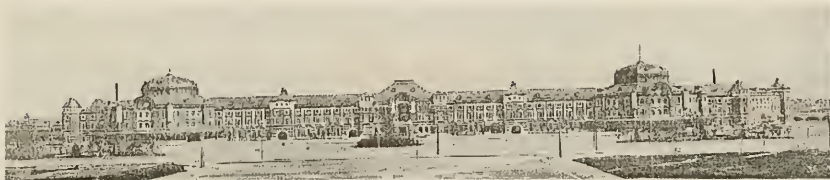
Figure 48 Tokyo Station in 1914
