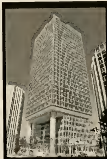
Figure 72 Japan Pacific Century Group Building
