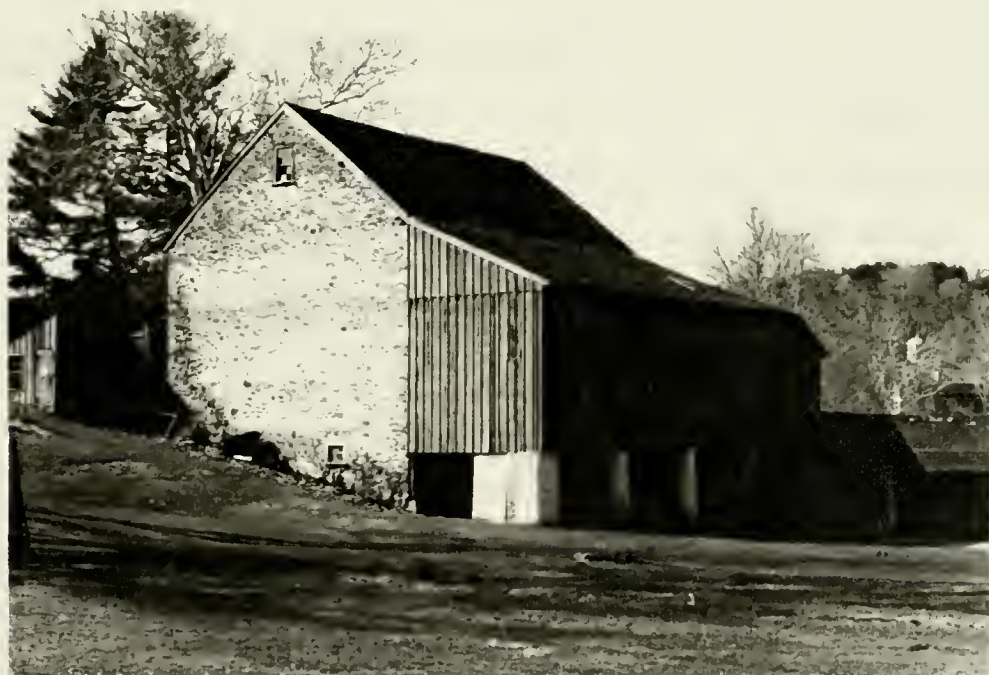
Fig. 10. Open Forebay. (Goldwater /Link) Bank Barn. Ridley Creek State Park.
