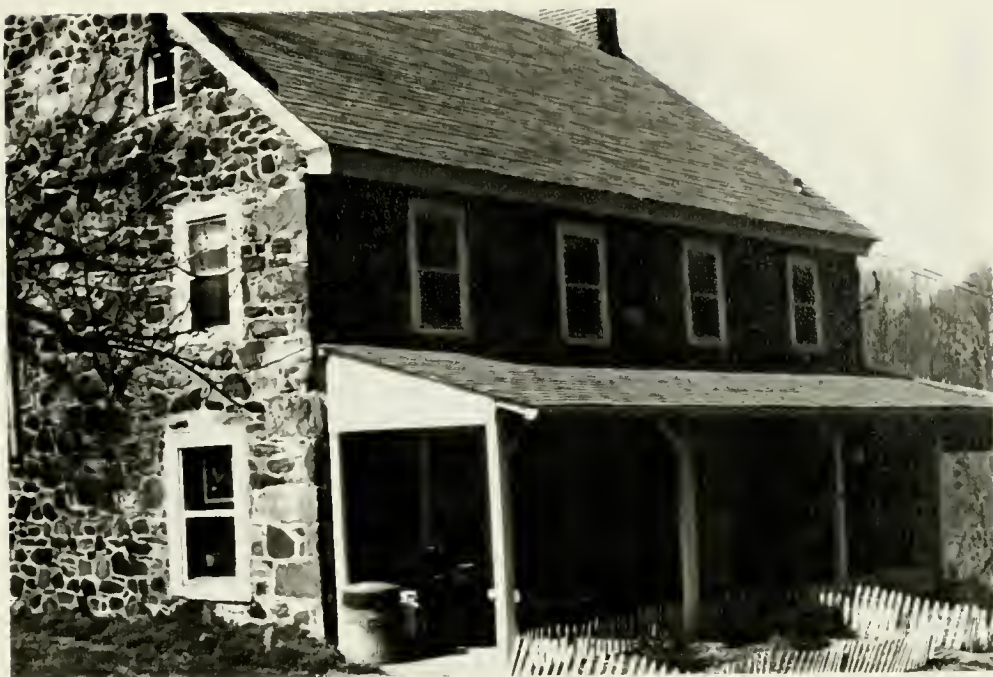
Fig. 21. Thomas Minshall II House (mid 18th c.). Ridley Creek State Park.
