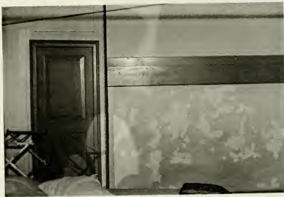
Fig. 1.10. John Worrall House. Detail of original 17th c. woodwork. Second Floor.
