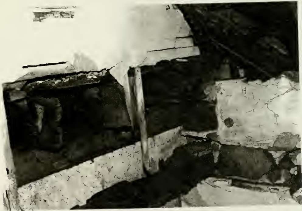
Fig. 2.12. Jacob Minshall House. Outlooker framing for original soffit on north facade.
