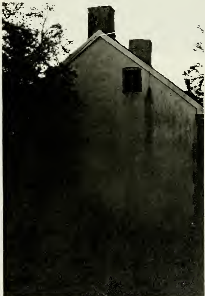
Fig. 3.4. Regester - Black House. East Facade.
