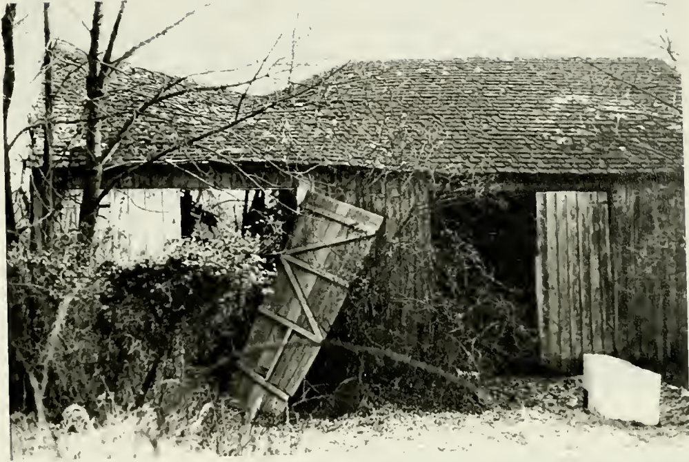
Fig. 3.7. Barn on Regester - Black farm.
