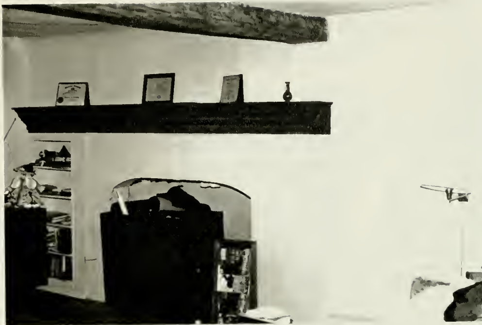
Fig. 1.9. John Worrall House. Detail of renovated fireplace elevation.
