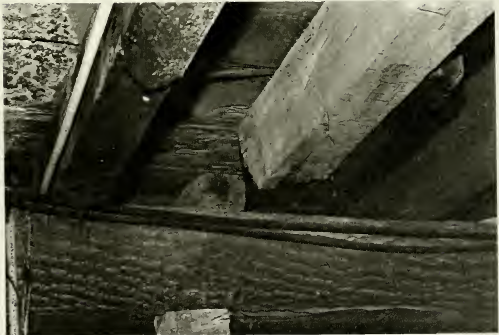
Fig. 1. 12. John Worrall House. Detail of original joists in 1703 section.
