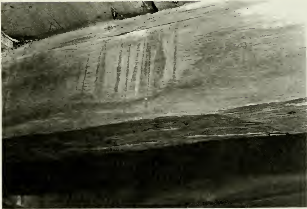
Fig. 1.8. John Worrall House. Detail of original pit sawn floor joists.
