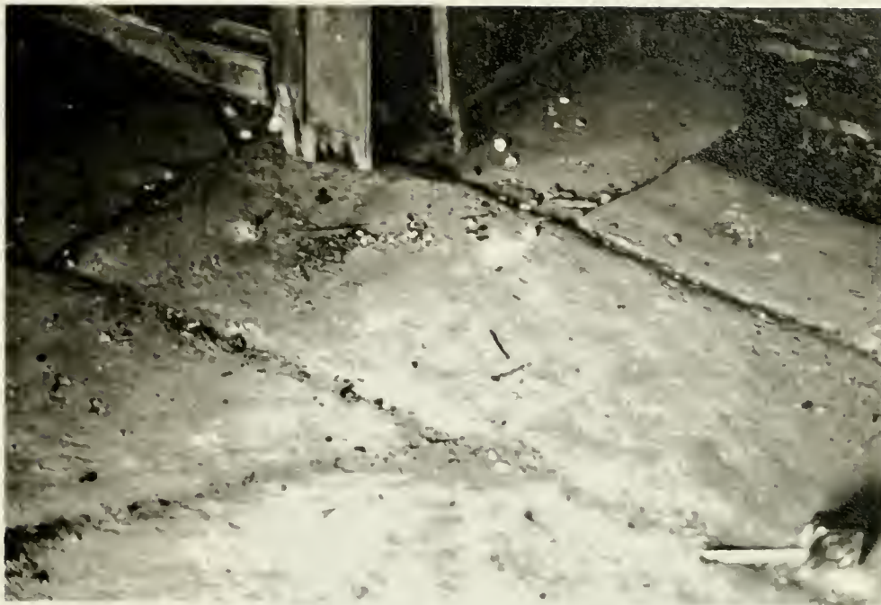
Fig 2.13. Jacob Minshall House. Original flagstone floor in kitchen ell.
