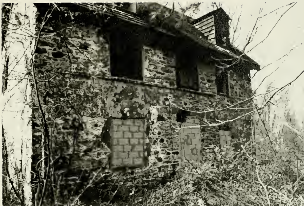
Fig. 2.1. Jacob Minshall House. South Facade.
