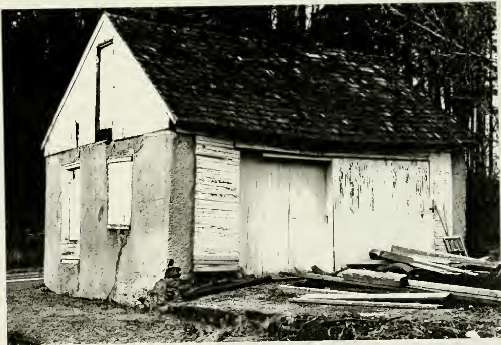
Fig. 3.8. Carriage House/ Chair Factory on Regester - Black farm.
