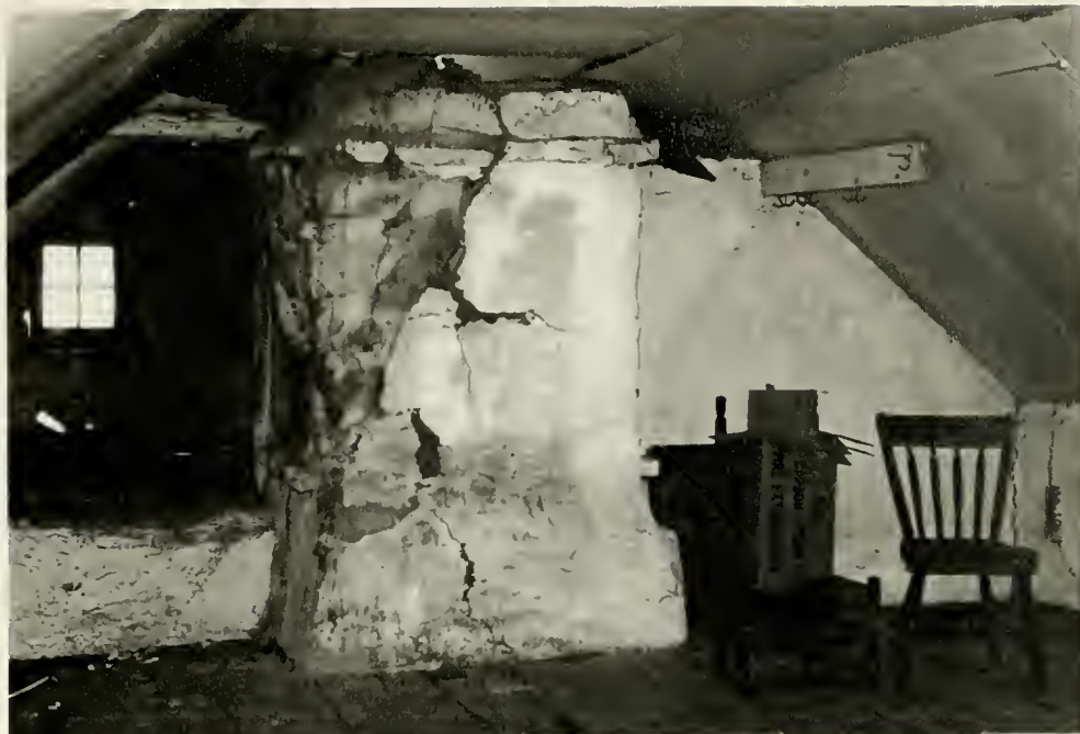
Fig. 3.9. Regester - Black House. Original terminus of chimney.
