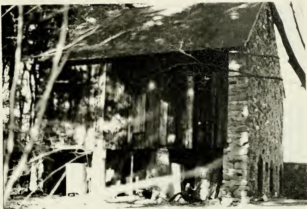
Fig. 1.5. John Worrall Barn. General View.
