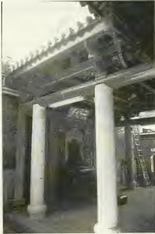
Fig. 3.6 Four pillars rebuilt in the Sichuiting (four-ridge pavilion) (photographed by the author)
