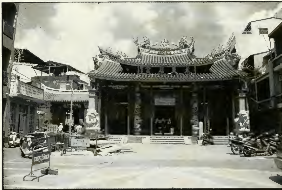
Fig. 3.4 Sanchuan Hall of the Da Tianhou Gong showing the pseudo- sichui roof (the second tier of roof) (photographed by the author)
