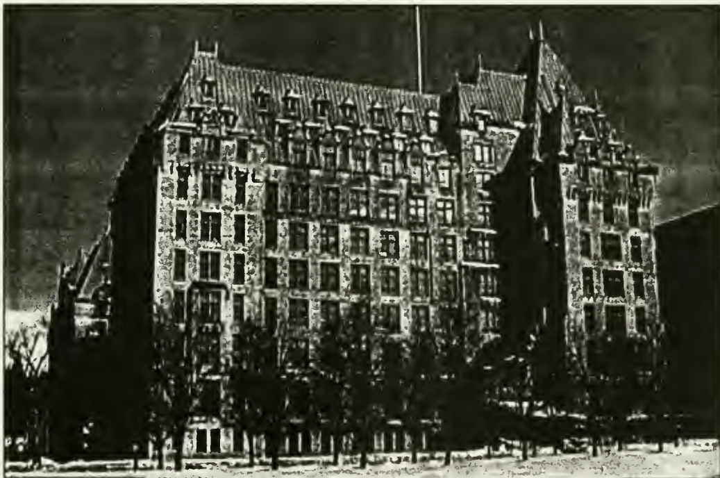
Fig. 32. The Justice and Confederation Buildings. Photo from the Long-Term Architectural Planning Office, Ottawa.
