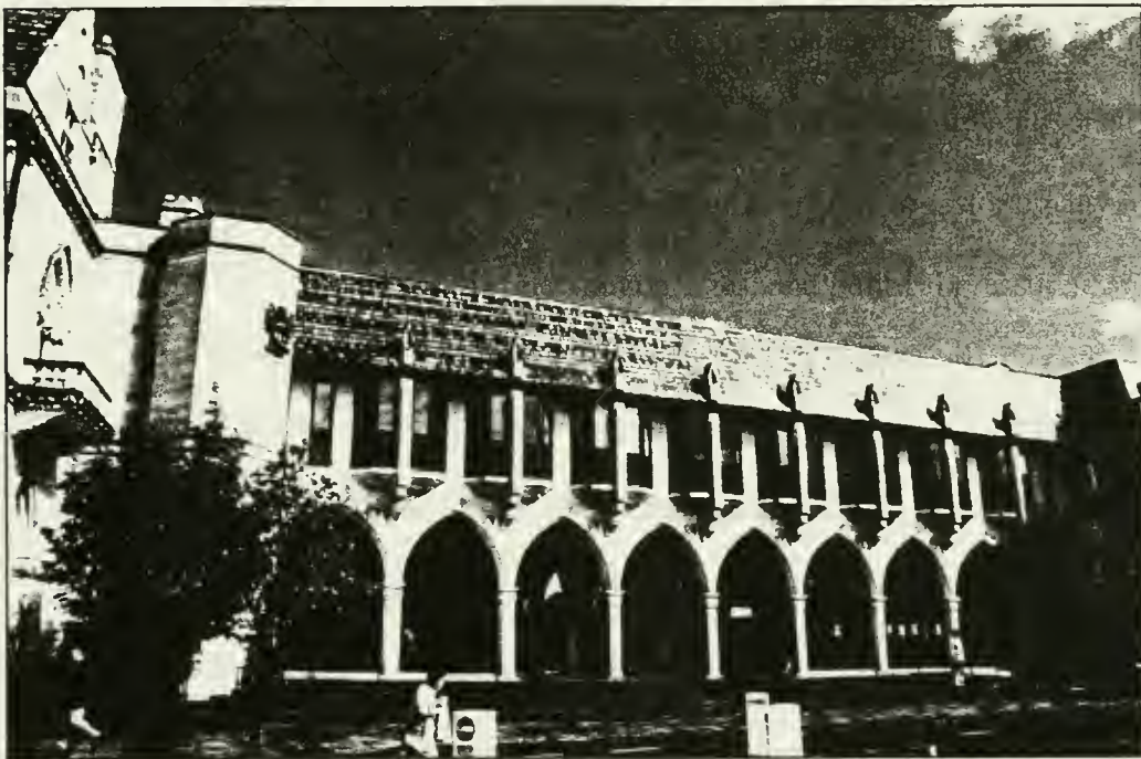
Fig. 39. The New Addition to the Guildhall . Photograph by the author, July 2001.
