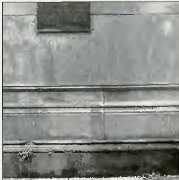
Fig. 20 - (2e.a) Microbiological colonization - algae, fungi, lichen and bacteria. Fig. 20 (2e.b) Colonization by higher plants.
