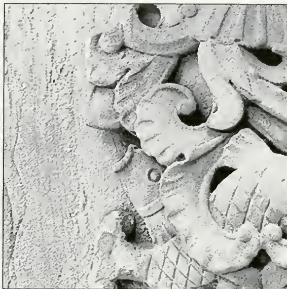
Fig. 9 - (1b.d) Exposure of stone components - raised exposure of stone aggregate through loss of less stable stone components.
