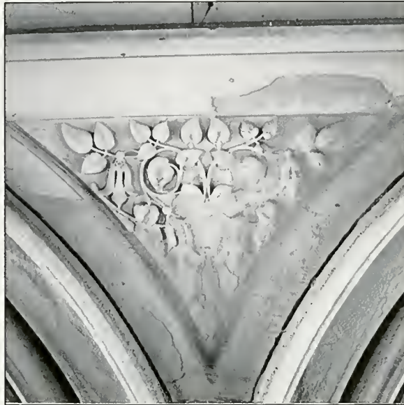
Fig. 19 - (2d.a) Dark/light or colored crust tracing the surface - crust tracing the morphology of the stone surface usually due to moisture related processes.
