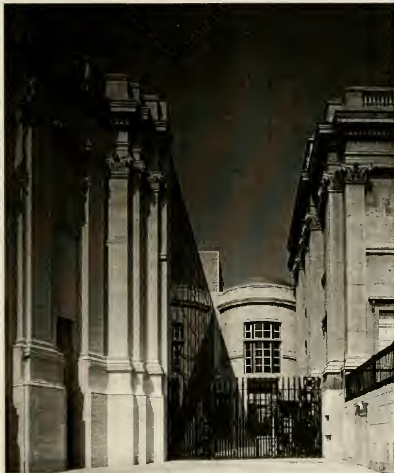
Fig. 4.10 – Old and new facades at Jubilee Walk.
