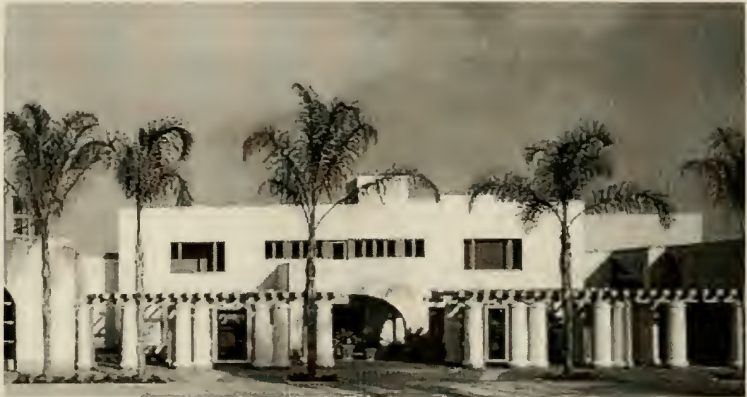
Fig. 3.8 – Detail of restored Scripps House façade.
