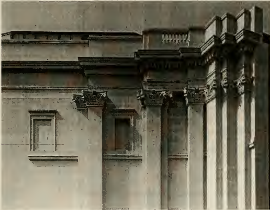
Fig. 4.12 – Applied pilasters on Sainsbury Wing façade.
