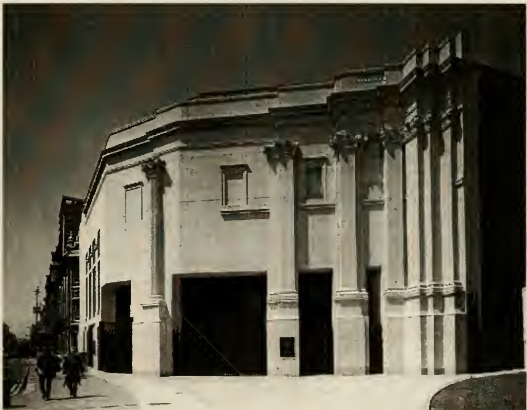
Fig. 4.5 – The Sainsbury Wing, Trafalgar Square façade.
