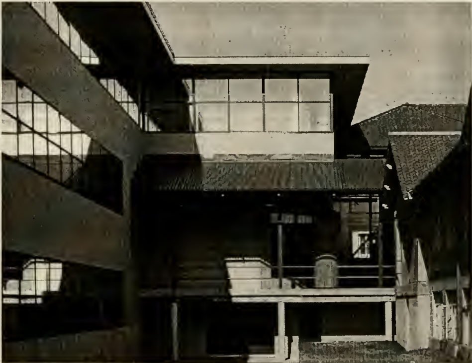
Fig. 2.8 – Rear façade at the connection between old and new.
