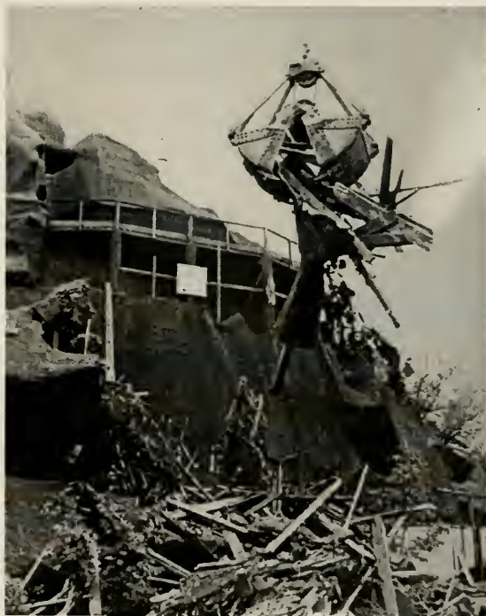
Fig. 3.24 Demolition of the Alps roller coaster, Willow Grove Park, 1980, in preparation for construction of the new Willow Grove Park mall.
