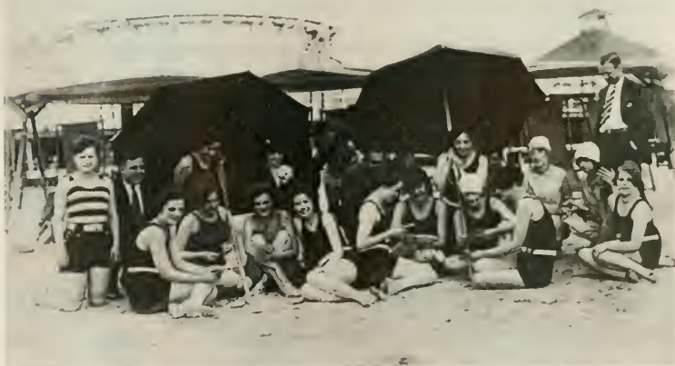
Fig. 4.14 Posing on the Wildwood beach, with the Jack Rabbit roller coaster in the background, 1927
