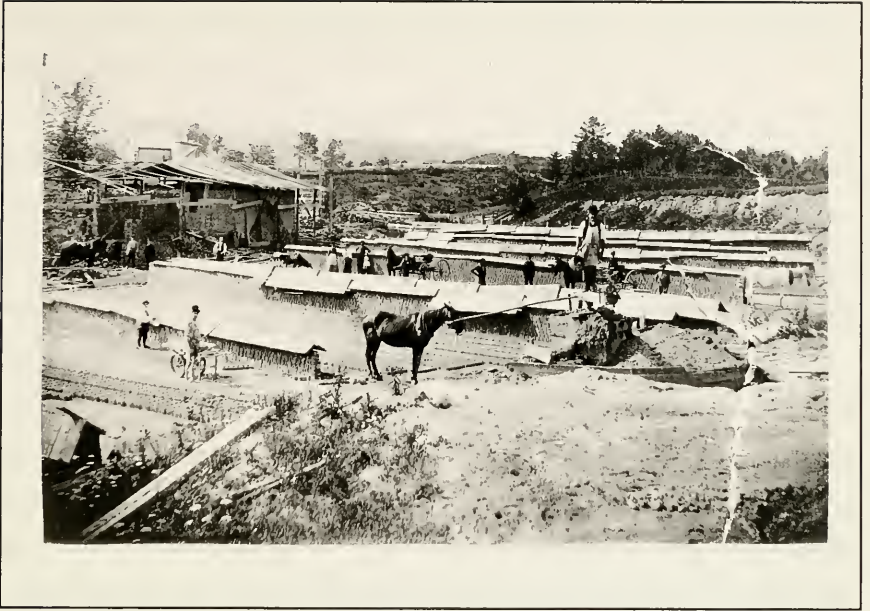
Figure 2. 1890 view of Fuller and Cony's Brickyard in Augusta, Maine. Note the horse powered pug mill and green brick s drying background.
