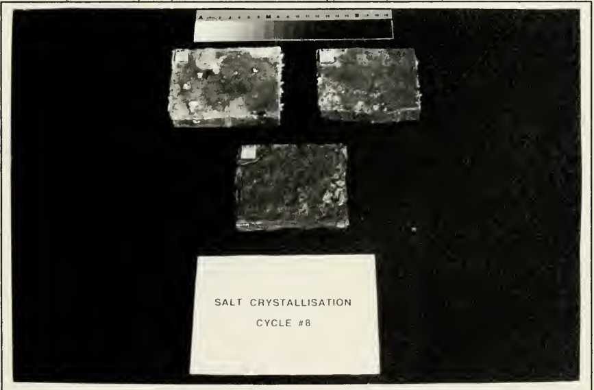
Figure 11 Brick Samples After Eight Cycles . Note the blistering, cracking, and decohesion of the bottom center (Type 1 sample). Both top (Type 2) samples exhibit salt crusting .
