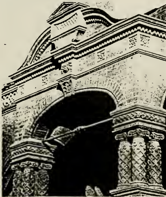
Textured Uimestone ELASTO WALL 351 provided a new stone-like finish without complete abrasive removal of existing paint from this church's cast stone elements.
