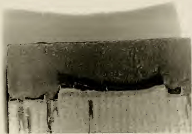
Figure B.28 Edison Aquathane UA-210-H specimen 1C mortar after 30 cycles. Note continued peeling of coating from glaze surface and map cracking.
