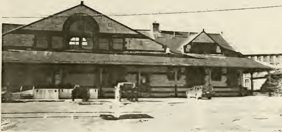
FIGURE 41: Connecticut River Railroad Station.
