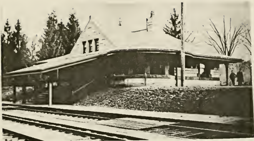
FIGURE 21: Photograph of Wellesley Hills Station.
