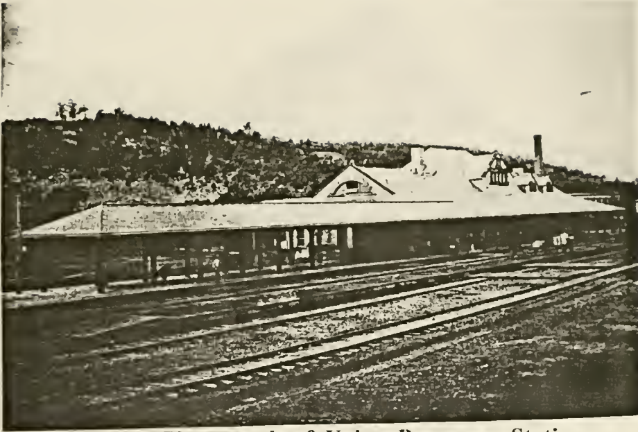
FIGURE 51: Photograph of Union Passenger Station.
