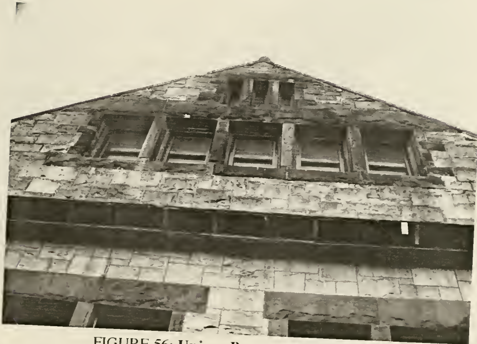
FIGURE 56: Union Passenger Station.
