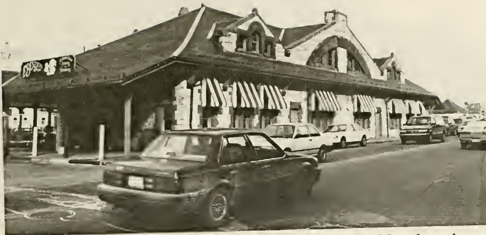
FIGURE 65: South Framingham Station, street-side elevation.
