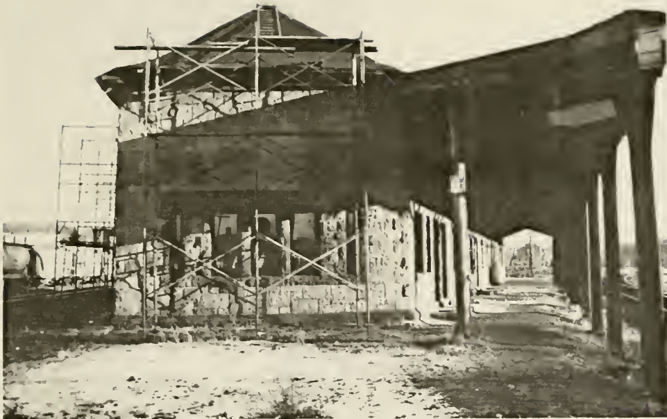
FIGURE 57: Union Passenger Station.
