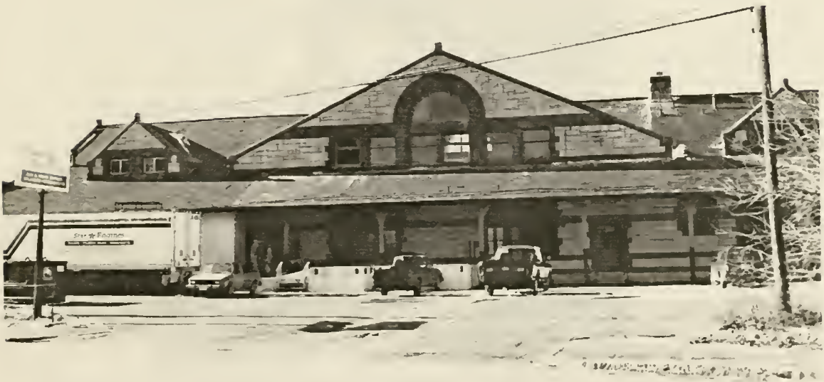
FIGURE 40: Connecticut River Railroad Station, now Auto-Parts shop.
