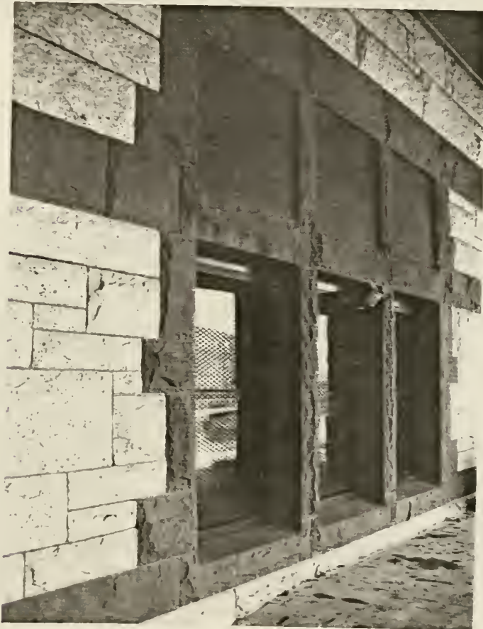
FIGURE 42: Connecticut River Railroad Station, cement-block filled windows.
