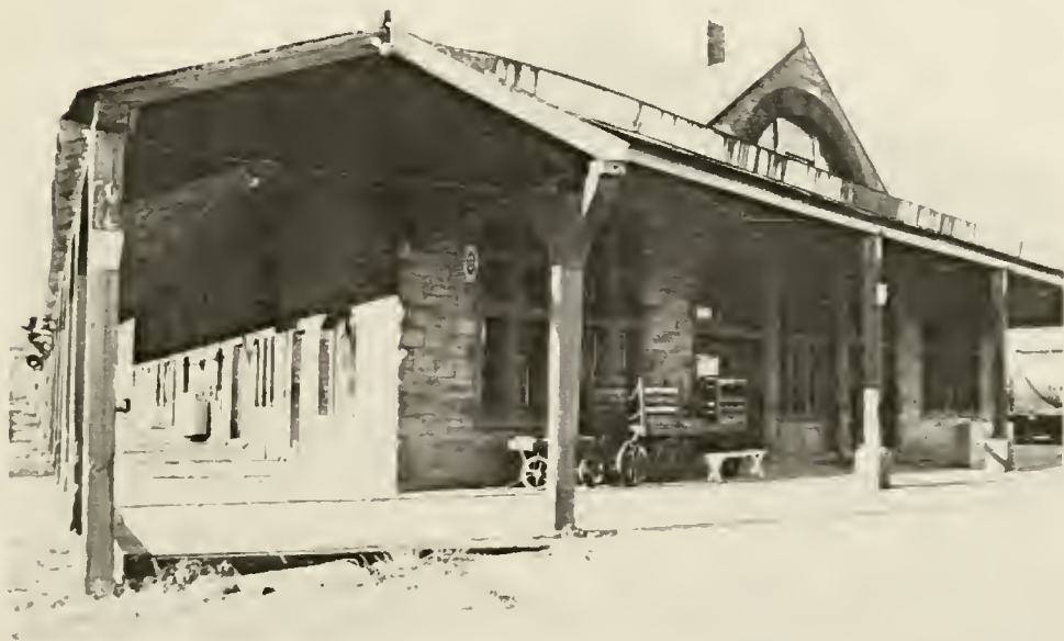
FIGURE 54: Union Passenger Station.
