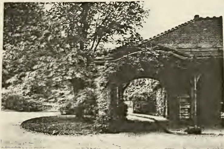
The entrance to the station through a vine-clad porte cochere
