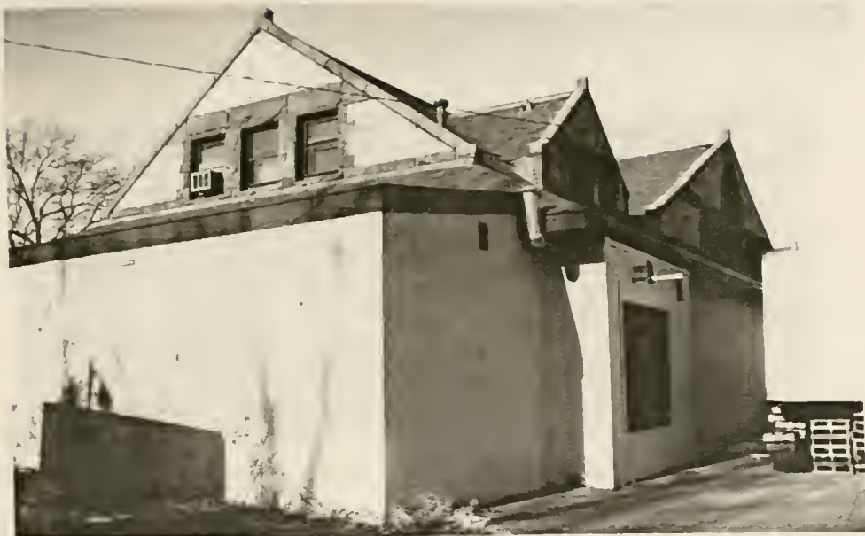
FIGURE 43: Connecticut River Railroad Station, alterations.
