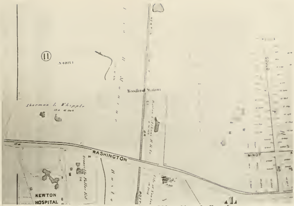
FIGURE 15: Atlas showing Woodland Station.
