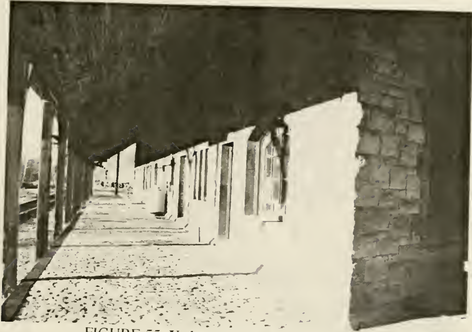
FIGURE 55: Union Passenger Station.
