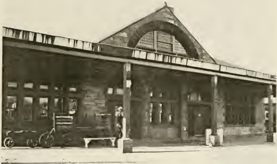
FIGURE 53: Union Passenger Station.
