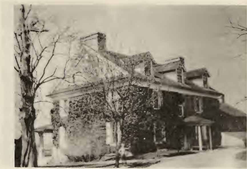
Figure 58. North elevation with three dropped-pendant style dormers, circa 1928. (Mutual Assurance Company, Policy No.10,478, June 21, 1928.)
