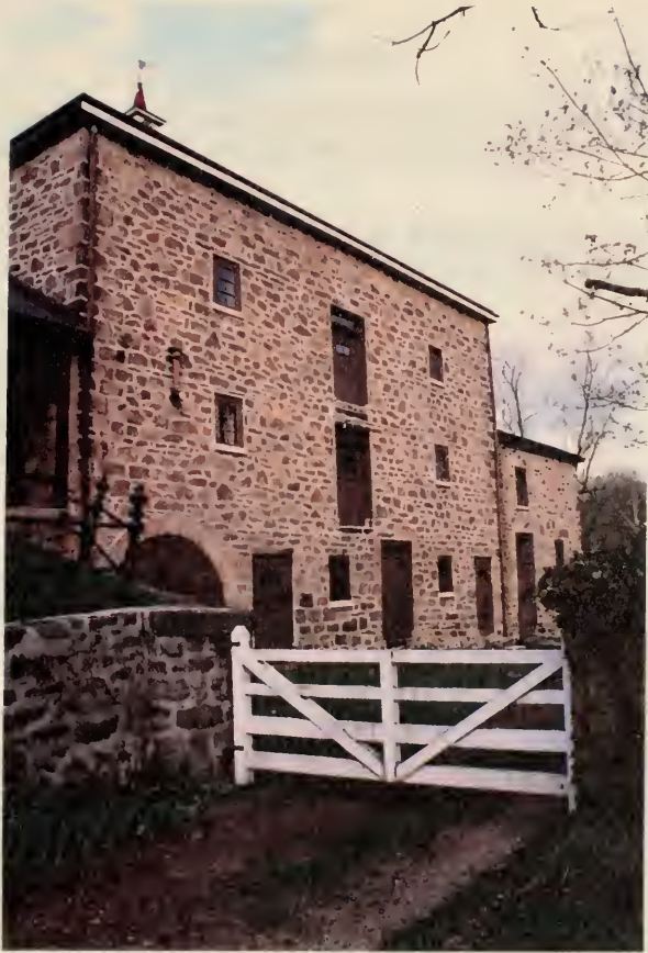
Figure 84. South elevation of original portion of the unique "double-decker barn." (1994)
