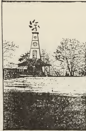
Figure 64. Windmill on terrace behind main house, first half of the twentieth century. (Mrs. William Francis, "Mill Grove - Home of John James Audubon," Mill Grove, Audubon, PA)
