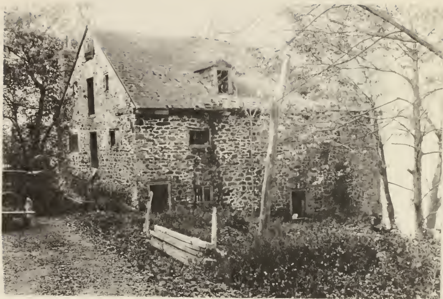
Figure 72. Latest known view of mill prior to its demolition in 1929. This photograph reveals the deteriorated condition of the building. (Mill Grove Files, Audubon, PA)
