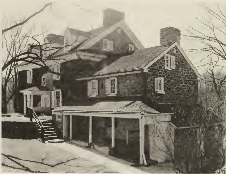
Figure 78. North and west elevations, circa 1952. (Mill Grove Files, Audubon, PA)
