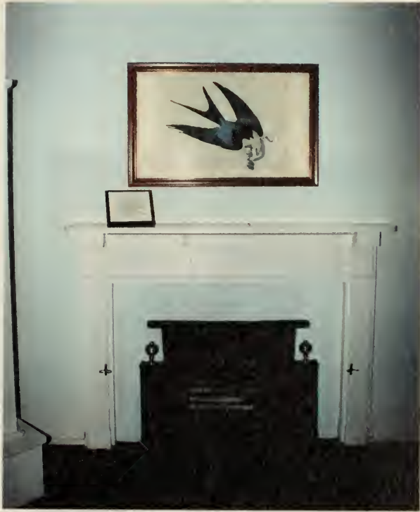
Figure 42. Corner fireplace in first floor southeast room illustrating the type of fireplace surround and coal grate added in the 1820s. (1993)
