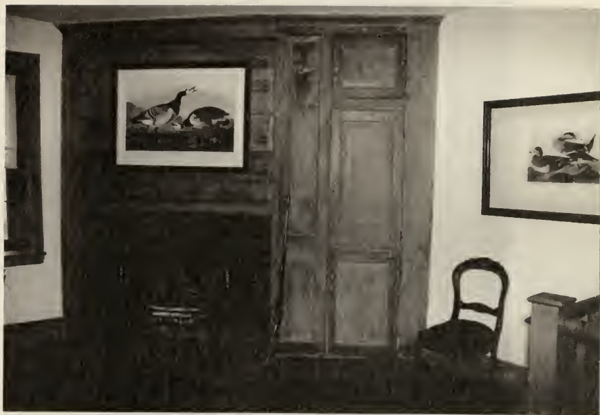
Figure 11. Eighteenth-century fireplace wall paneling in second floor northeast room. (1993)
