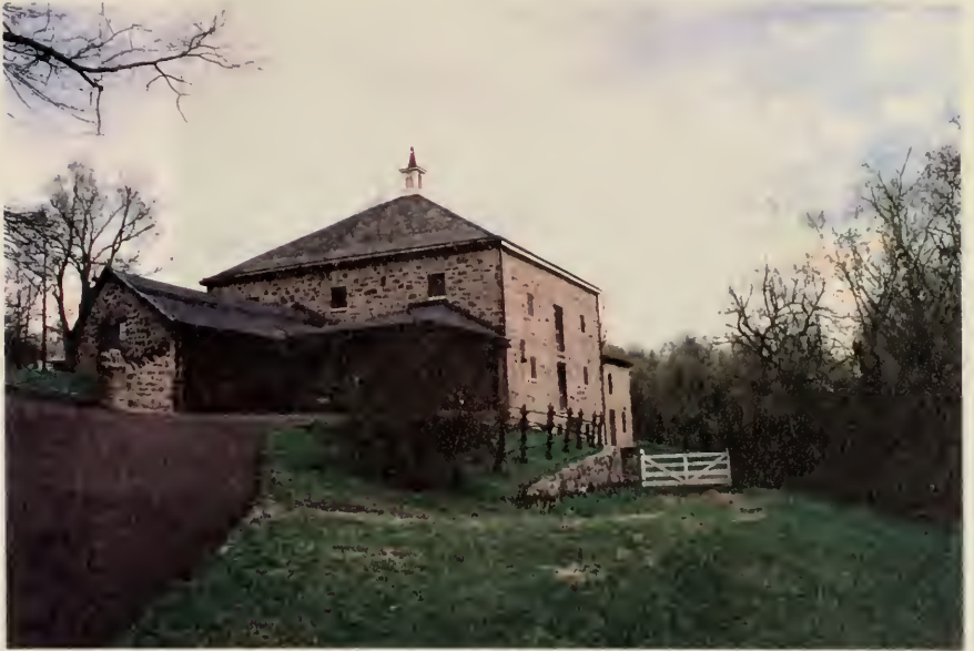
Figure 83. South and west elevations of the Mill Grove barn. (1994).
