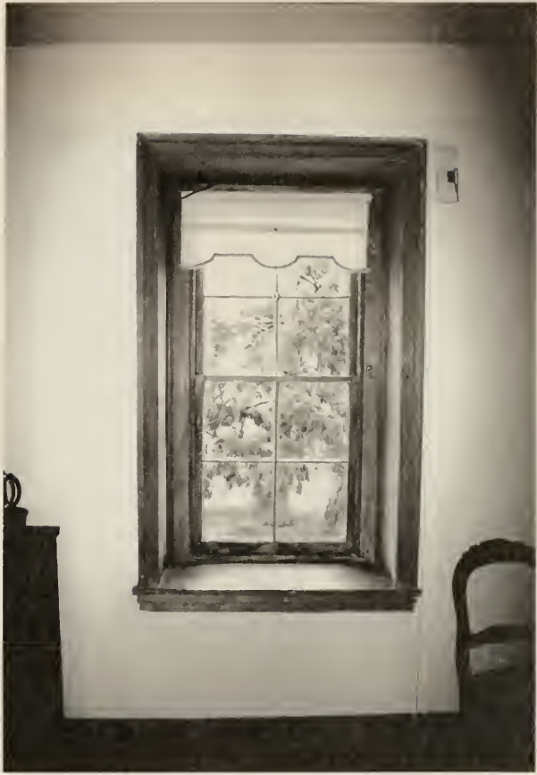
Figure 41. Interior view of north window in second floor northeast room illustrating an example of the type of windows that were installed in the 1820s. (1993.)
