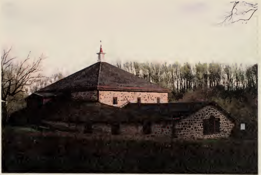
Figure 82. Northwest elevation of Mill Grove barn. (1994)
