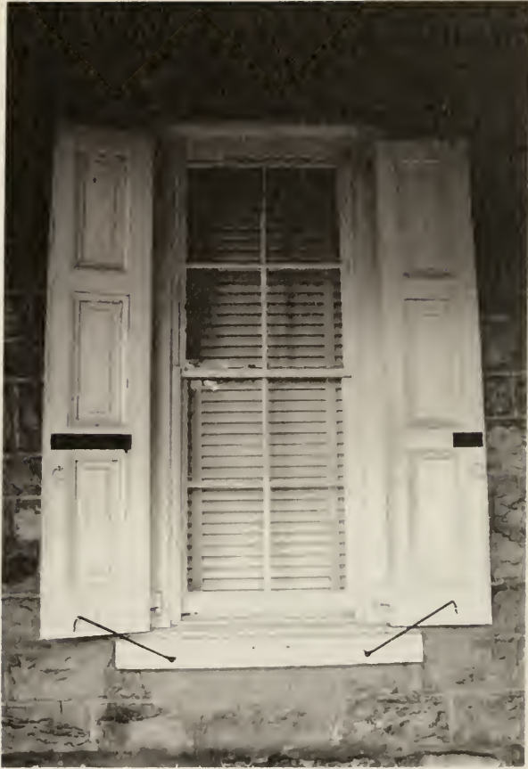
Figure 39. First floor window on south elevation of main section, illustrating an example of the type of window and shutters that were installed in the 1820s. (1994)
