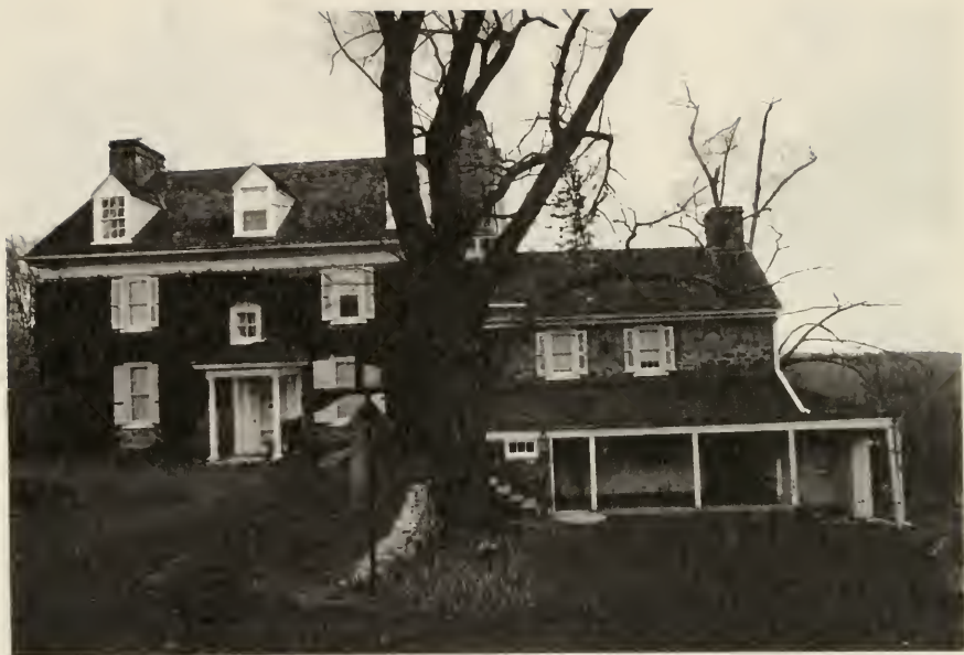
Figure 14. North elevation of Mill Grove mansion showing the kitchen wing attached at a significantly lower grade. (1994)
