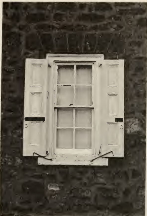
Figure 40. First floor window on south elevation of kitchen wing showing the type of window that was installed in the 1820s. (1994)
