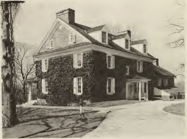
Figure 77. North and east elevations, circa 1952. (Mill Grove Files, Audubon, PA)
