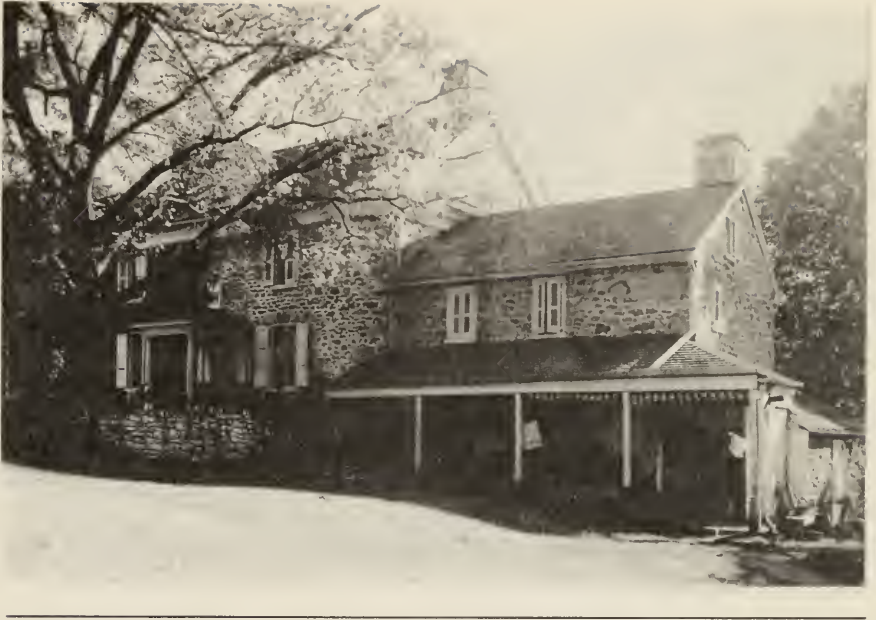
Figure 56. North elevation showing kitchen porch with stove and rolled awning, believed to date to late nineteenth or early twentieth century. (Mill Grove Files, Audubon, PA)
