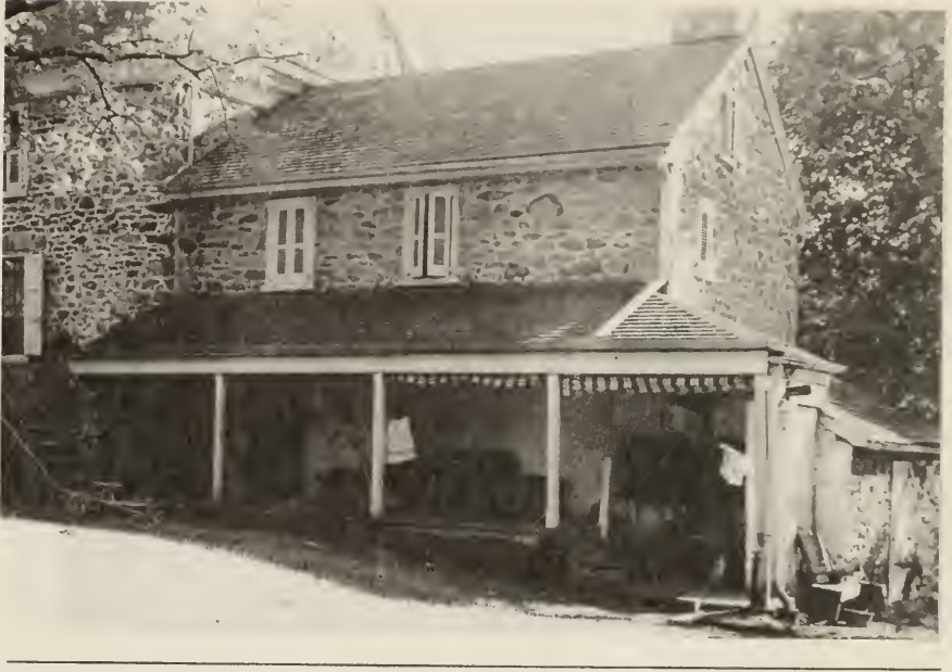
Figure 57. Detail of kitchen porch in figure 52. (Mill Grove Files, Audubon, PA)
