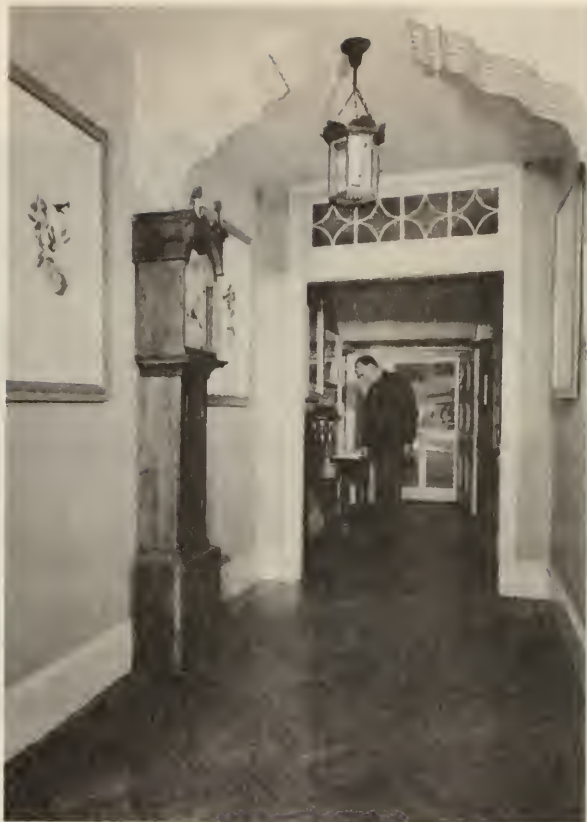
Figure 80. First floor center hall, looking north, showing the parquet floor and ornamental brackets installed by the Wetherills to conceal pipes, early circa 1950s. (Mill Grove Files, Audubon, PA)
