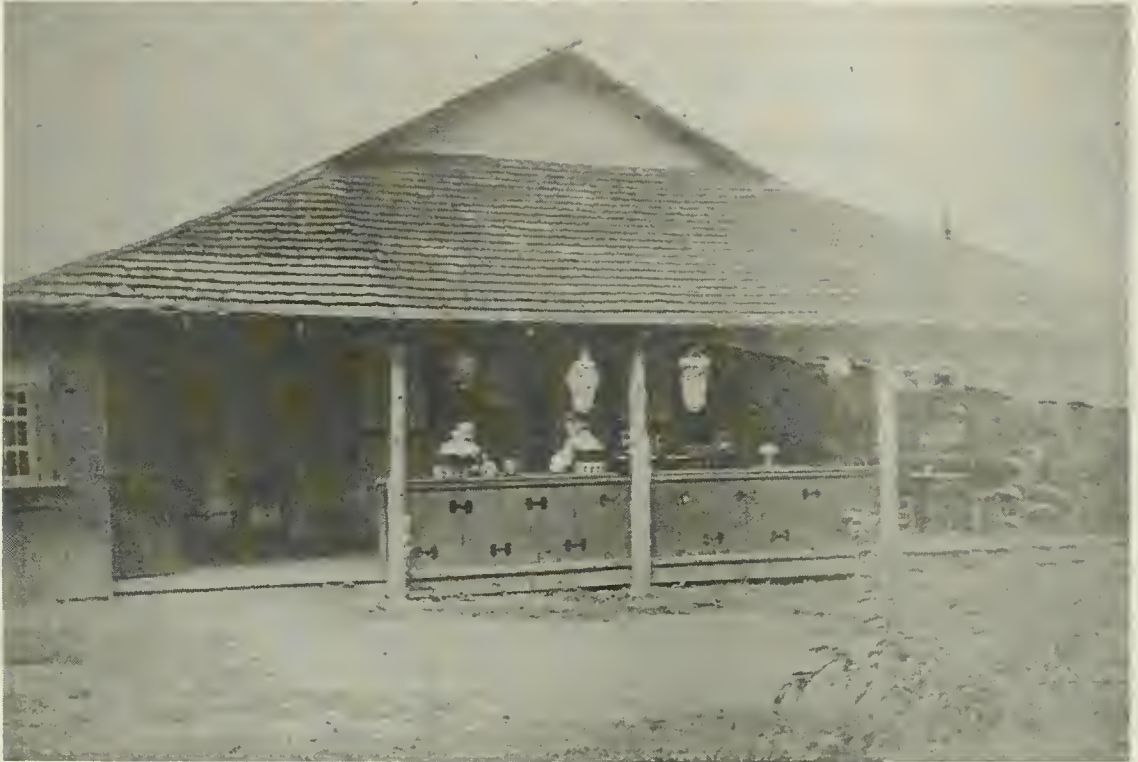
Plate 71. The Cooler. Built as an ice cream parlor. Courtesy Peg Aumack.
