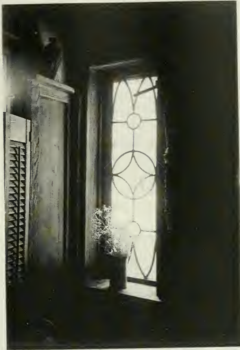
Plate 59. Katherine Ross Bungalow. Interior view illustrates the use of unpainted woodwork and leaded glass windows. Photograph by author, 1992.
