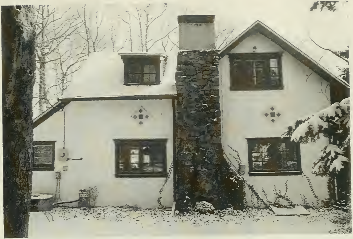
Plate 45. Green Gate. North facade. Built in 1909. Designed by William Price, this house incorporated a number of his signature details including the rough stone chimney, the plaster construction and, most notably, the decorative tiles embedded in the exterior plaster. Photograph by author, 1993.
