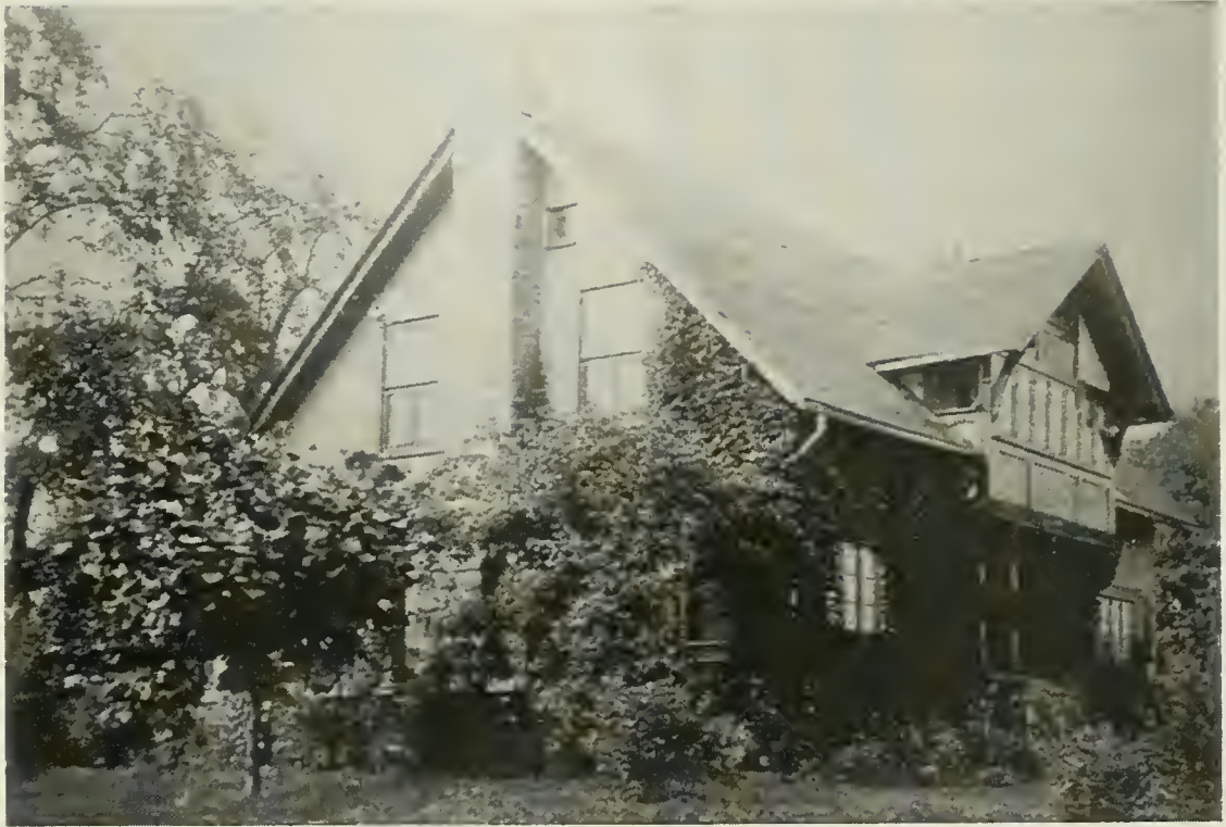
Plate 52. The Lodge. Southwest view of The Lodge, early photograph, exact date of photograph unknown. This house was built for Miss Lucy Darling who had previously been residing in the Red House. The Lodge, designed by William Price, was started in 1910. This house, like the Second Homestead, Rest Cottage, and Friendly Gables, was constructed of hollow tile and plaster. But unlike the other structures it is symmetrical with a broad center dormer projecting from the front facade and a chimney at both the east and west ends of the house. Courtesy Don Holcomb.
