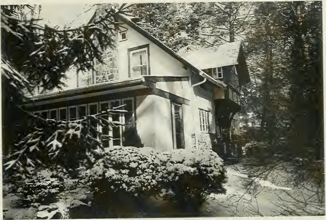
Plate 53. The Lodge. West facade. Photograph by author, February 1993.
