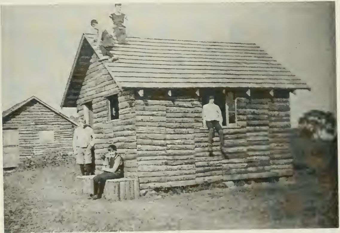
Plate 36. First Cabin. This building was one of a series of cabins designed during Arden's first phase of building. It is a very simple dwelling, built of plywood with a log veneer. The cabin has no chimney. Courtesy Peg Aumack.
