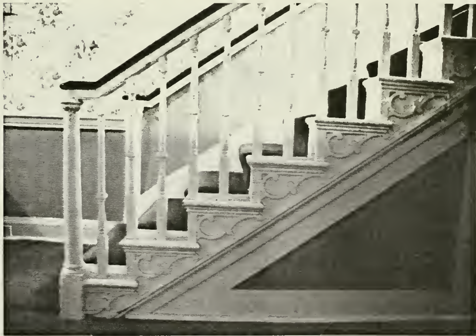
Plate 24 [above]: Entry Hall [Room 103], looking south towards transomed front entry Plate 25: Staircase in Entry Hall, showing tread profile detail and wainscoting, and in background, handrail pilasters on wall, looking west
