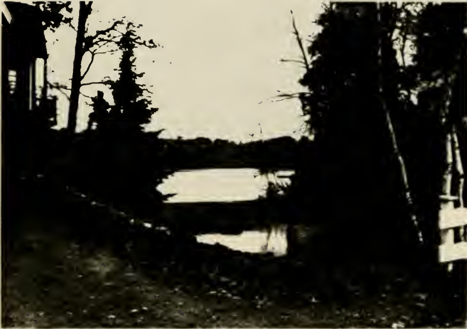
Fig. 23. The dam at Lake Arrowhead.
