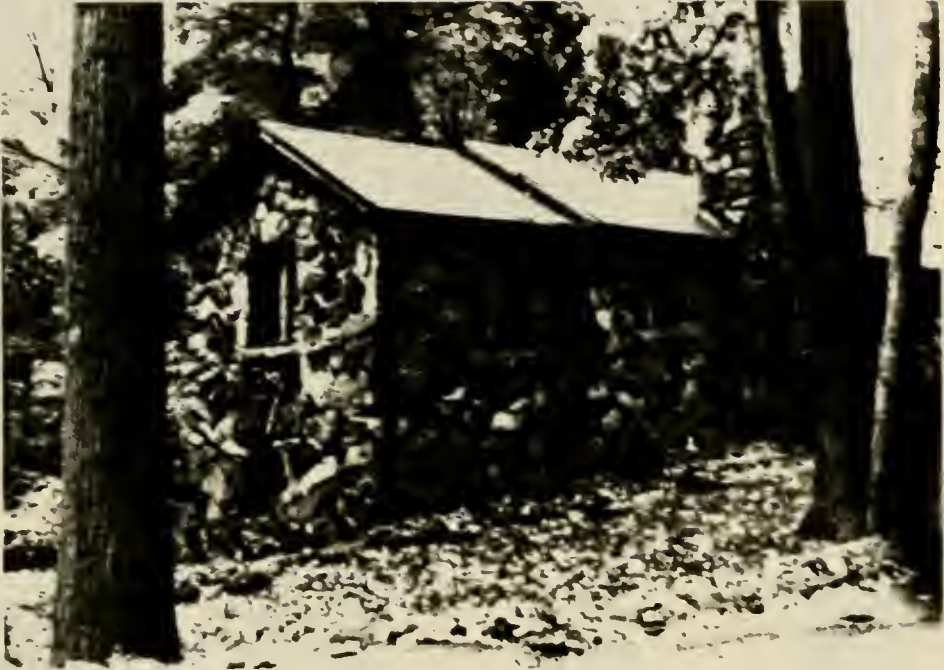
Fig. 45. One of the small, year-round, stone cottages built near Lake Valhalla in the 1930s.
