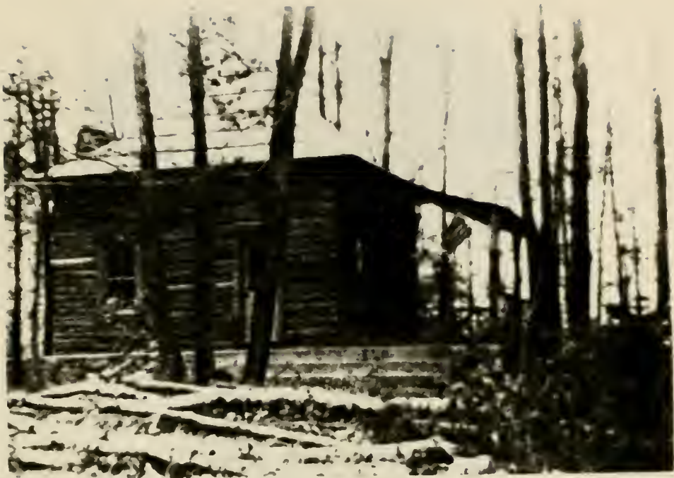
Fig.15. The first crudely-built, log-sided cabin on Cedar Lake, 1907.
