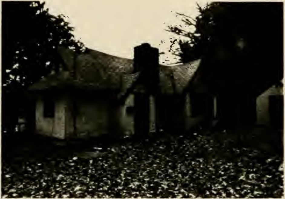
Fig.30. A Lake Arrowhead English cottage with "sagging roof," field stone chimney, and oriel window.
