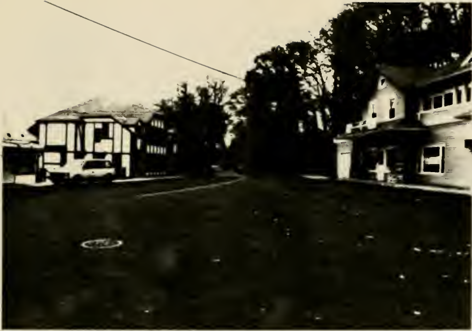
Fig.36. The small commercial strip inside the entrance to Indian Lake. Building on right originally clad in shingles.
