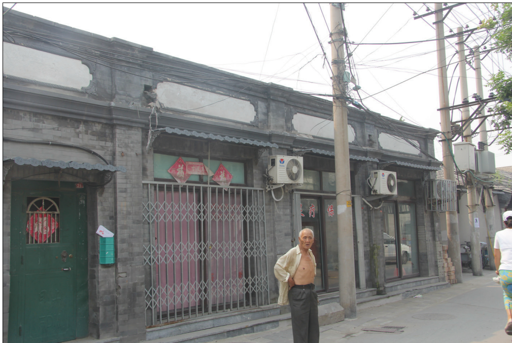
FIGURE 1-11: BUILDINGS CAN BE REPAIRED, REUSED, RATHER THAN DIRECT REMOVAL
