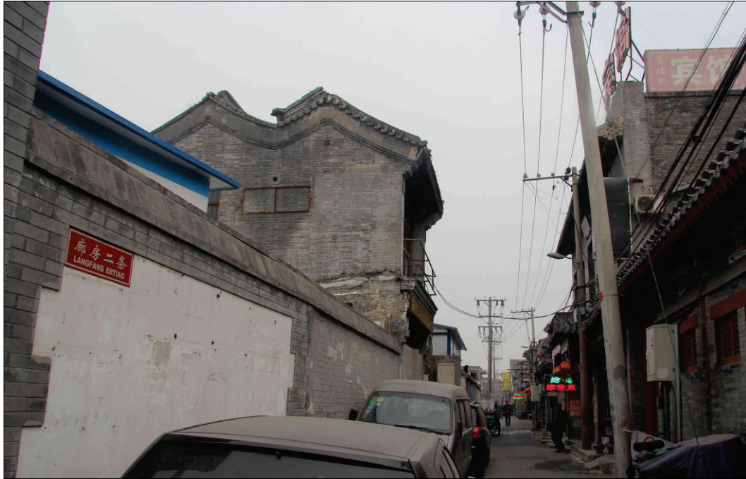
FIGURE 5-12: THE CURVED SLOPING ROOF (COMPARING TO THE REGULAR ONE ON THE LEFT)
