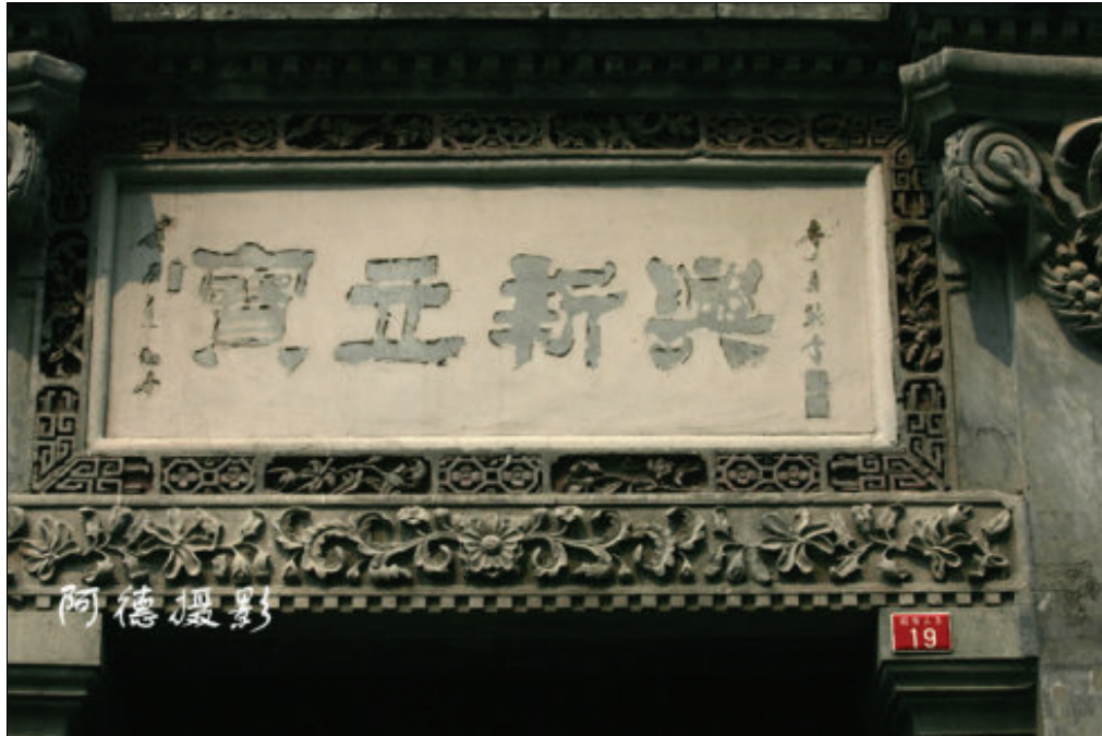
FIGURE 4-15: BRICK DETAILS ON A DEMOLISHED EXQUISITE BUILDING
