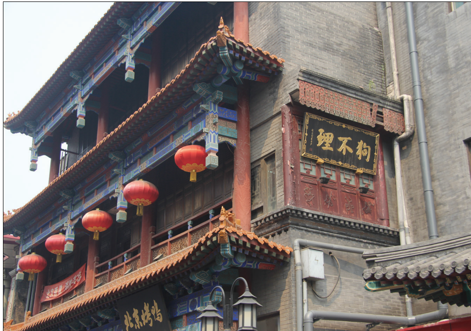
FIGURE 1-13: IS THIS FAÇADE ORIGINALLY THERE?
