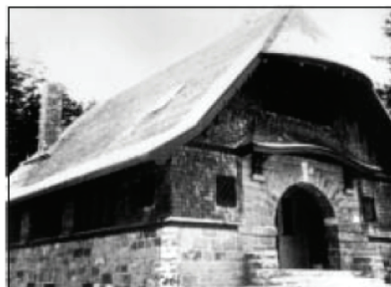
Shingle-Style church. North and east elevations after rehabilitation.
