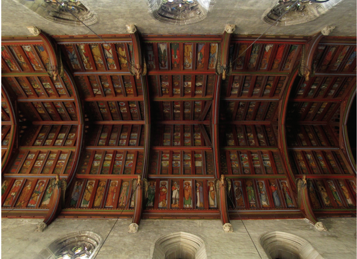
Figure 22: St. Andrew's Chapel "Panel and hammer beam ceiling depicting biblical figures" (photo courtesy of The University of Pennsylvania Graduate Program in Historic Preservation, fall 2010)
