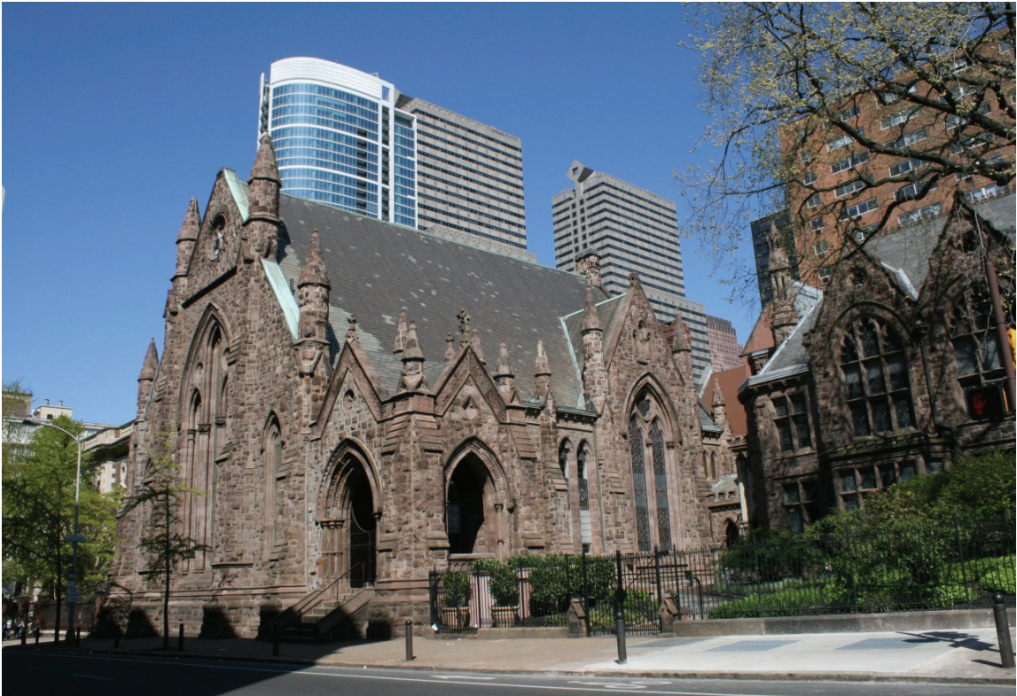
Figure 10: Exterior view of the former Church of the New Jerusalem, currently Corporate Facilities Offices (photo by the author, April 2012)
