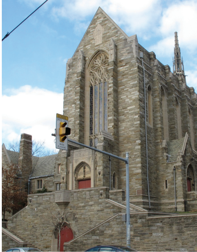
Figure 20: St. Andrew's Chapel South façade, Philadelphia (photo courtesy of the University of Pennsylvania Graduate Program in Historic Preservation, 2010)
