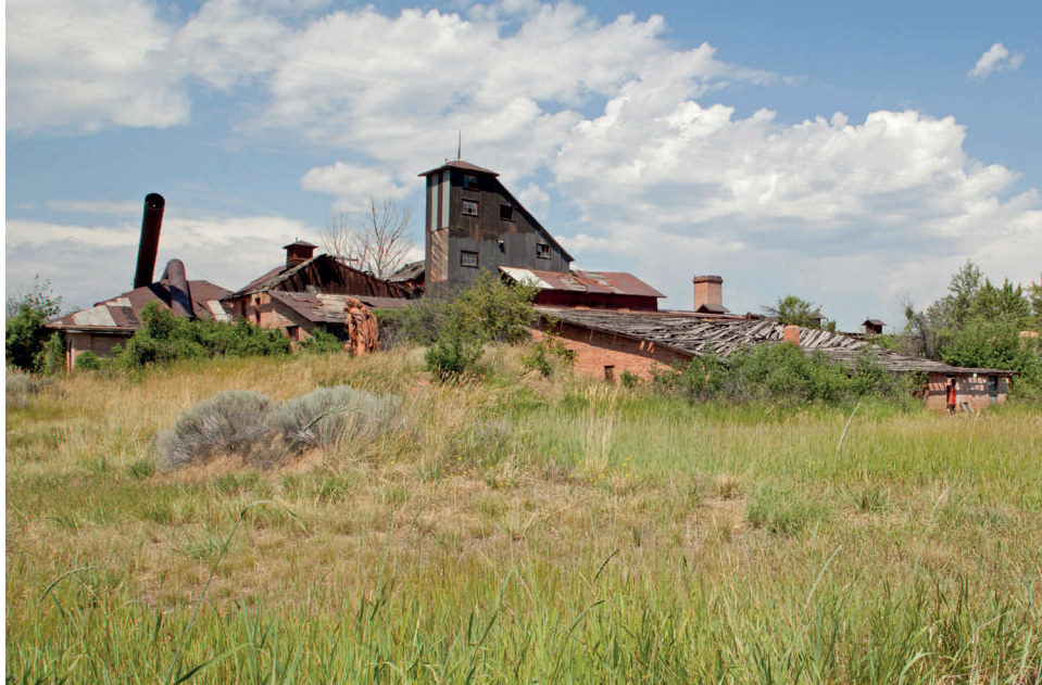
Figure 3.5: Compilation of buildings comprising part of the Western Clay Tile Works. Pictured are the power House, the machine shop, the elevator tower, and a section of the clay storage room. Joe E. B. Elliott, photographer, July 2011. Courtesy of the University of Pennsylvania Architecture Conservation Laboratory.
