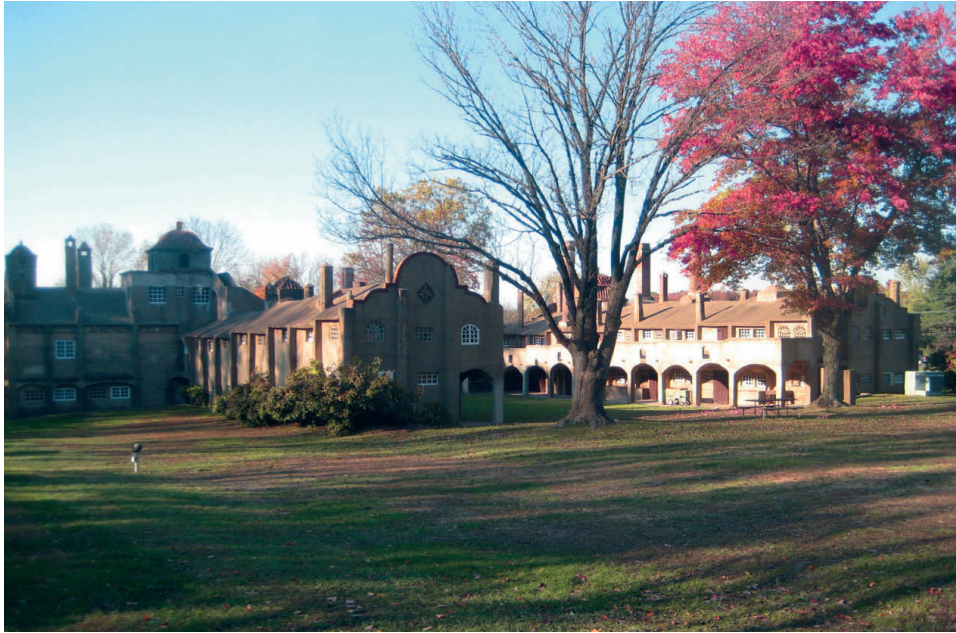
Figure 3.11: Moravian Pottery and Tile Works. Image courtesy of author, 2011.
