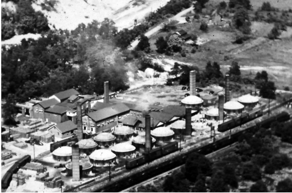
Figure 2.18: Image showing the location and arrangement of beehive kilns. Image of the North Mountain Brick Plant in Eastern West Virginia. Photographer unknown, circa 1950. Image Courtesy of Jeff Hollis, Continental Brick Company, Martinsburg, WV.
