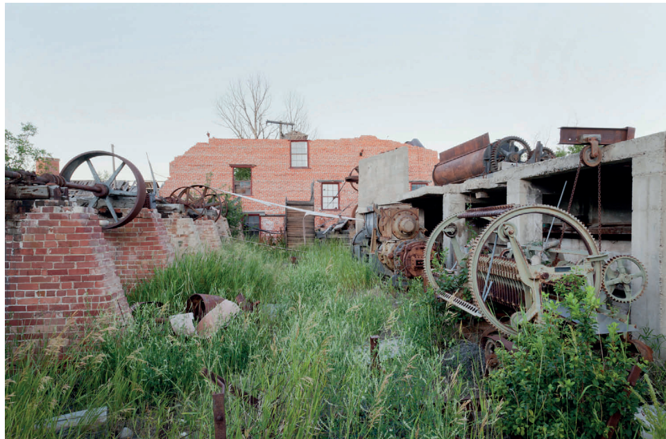
Figure 3.22: Brick shop remains. Joe E. B. Elliott, photographer, July 2011. Courtesy of the University of Pennsylvania Architecture Conservation Laboratory.
