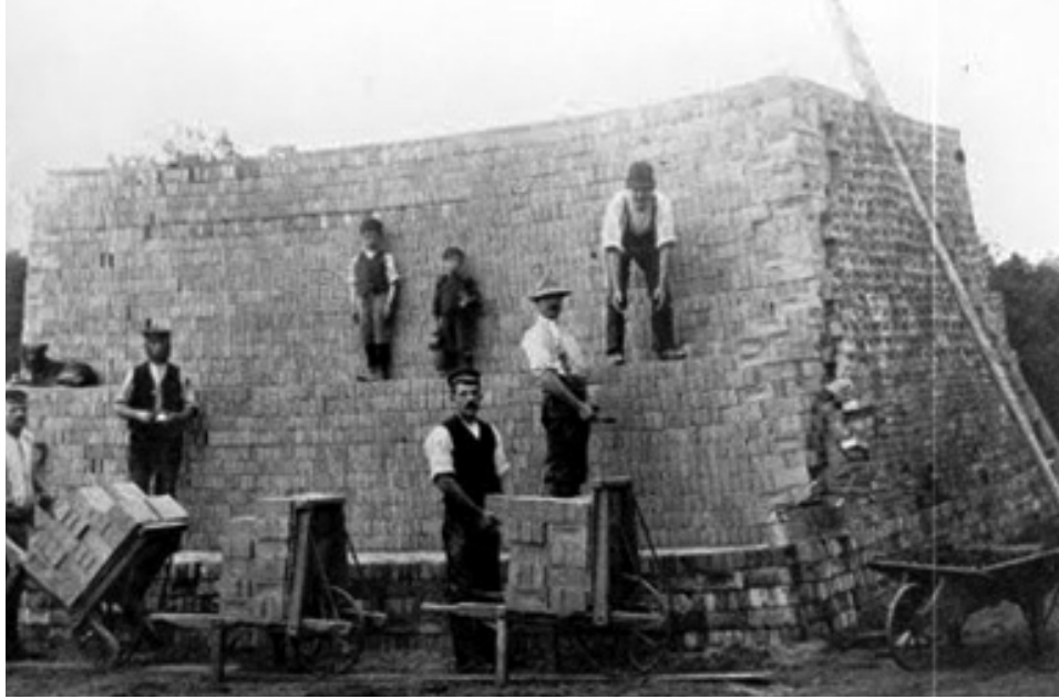
Figure 2.12: "Men building a clamp kiln to fire the raw brick. Photographer unknown, circa 1900. From Old Canal Pottery, http://madpotter-oldcanalpottery.blogspot.com/ .
