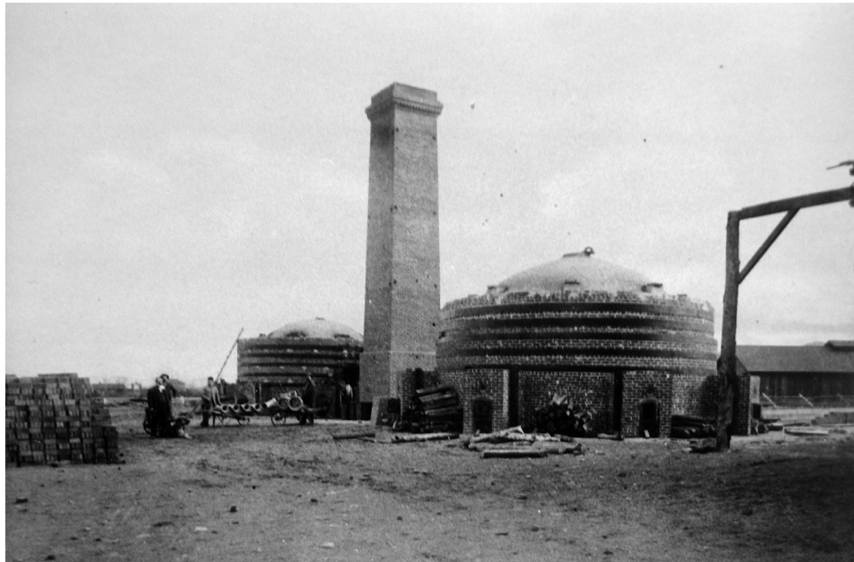
Figure 2.16: "Early beehive kilns at either the Kessler or Western Clay Works." Courtesy of the Montana Historical Society, Helena, MT.
