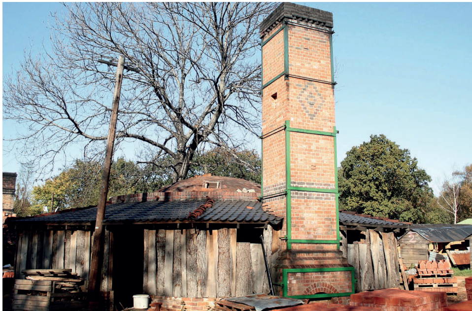
Figure 2.19: 1890s era beehive kiln with shed roof. Bulmer Brick and Tile Company, Ltd., Suffolk UK. Peter Minter, photographer, date unknown. Image courtesy of Peter Minter.
