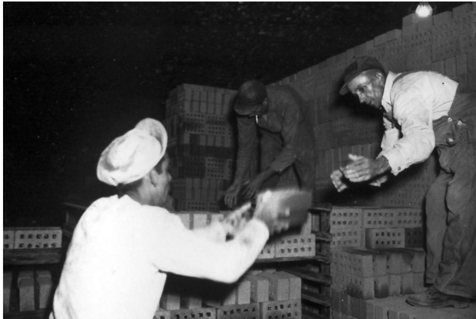
Figure 2.42: Image of a setting gang. "Continental Brick, Arlie's Gang." Photographer unknown, circa. 1940. Image Courtesy of Jeff Hollis of the Continental Brick Company, Martinsburg, WV.
