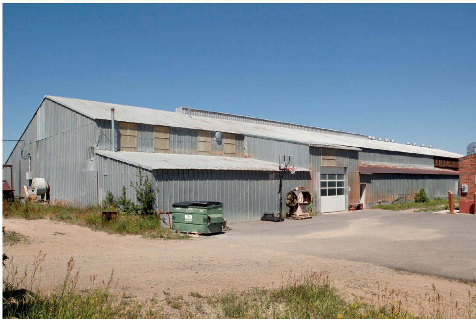
Figure 3.20: Building housing the Western Clay tunnel kiln. Joe E. B. Elliott, photographer, July 2011. Courtesy of the University of Pennsylvania Architecture Conservation Laboratory.
