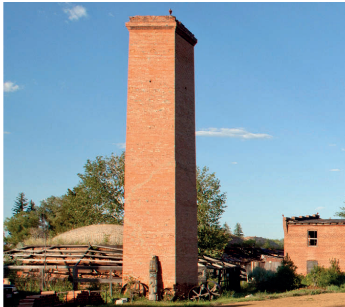
Figure 3.14: Chimneystack associated with Western Clay’s kiln “Number 6.” Joe E. B. Elliott, photographer, July 2011. Courtesy of the University of Pennsylvania Architecture Conservation Laboratory.
