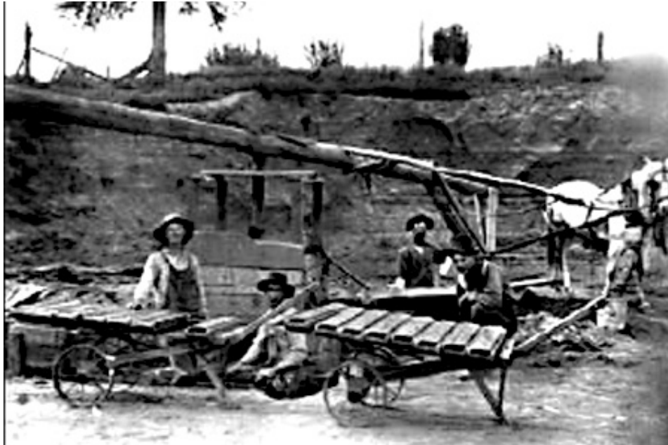
Figure 2.10: Horse operated pug mill at the Soft Salida Brick Company. Image courtesy of the Salida Library. From http://cozine.com/2009-october/the-story-of-soft-salida-brick/ .
