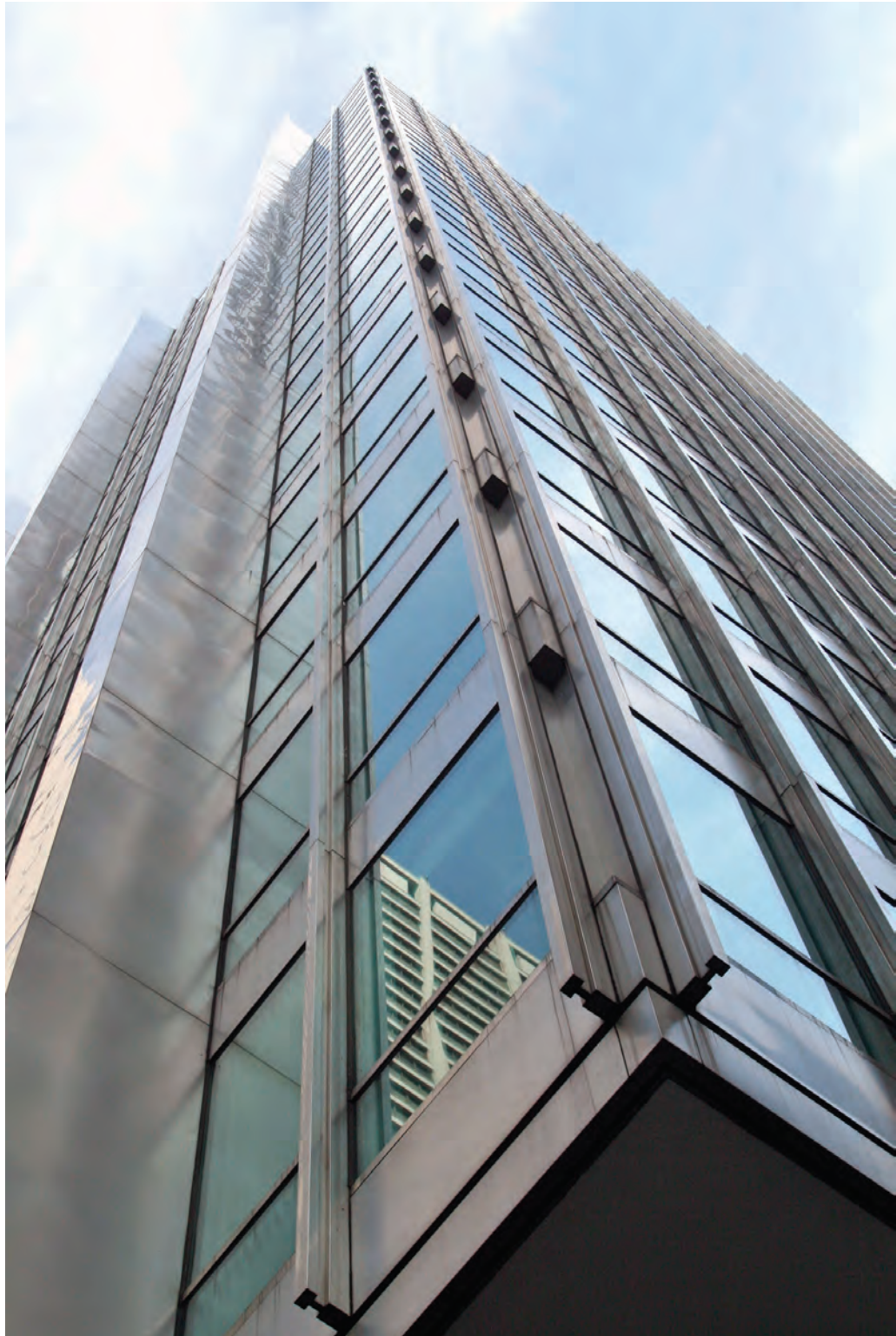
Figure 5.16: Corner Detail of Office Tower. Source: the author, 2012.
