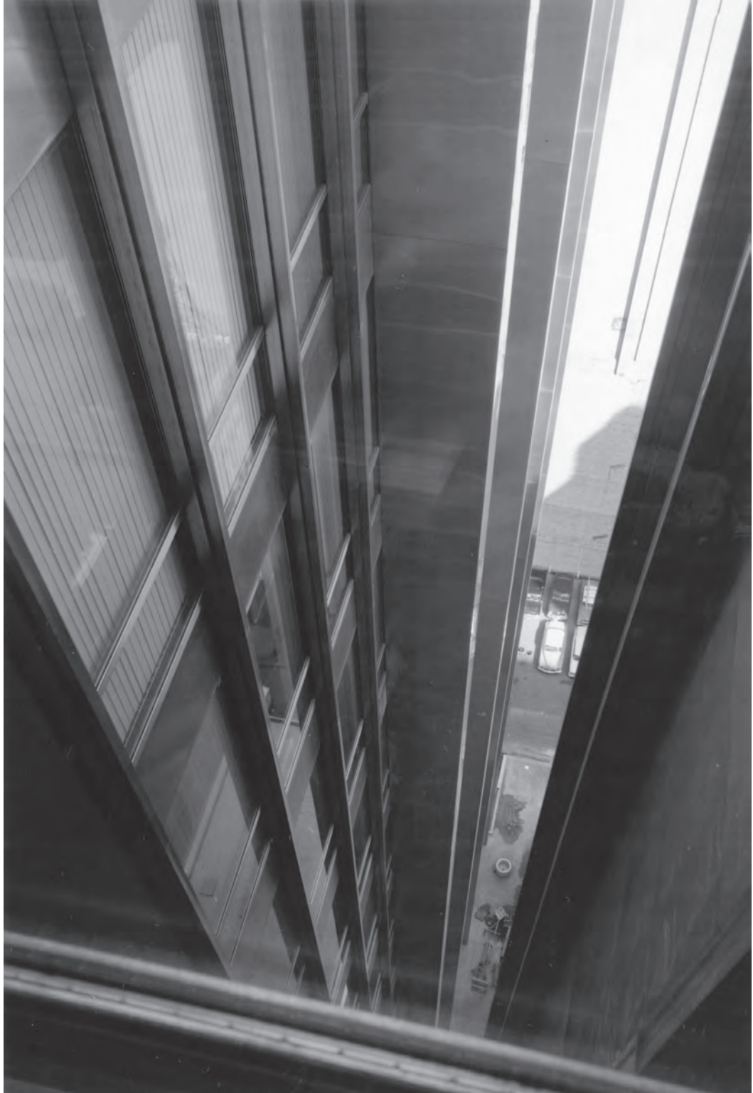
Figure B.11: View Looking Down between Office and Service Towers. Source: Ezra Stoller, SOM Archives, 1958.
