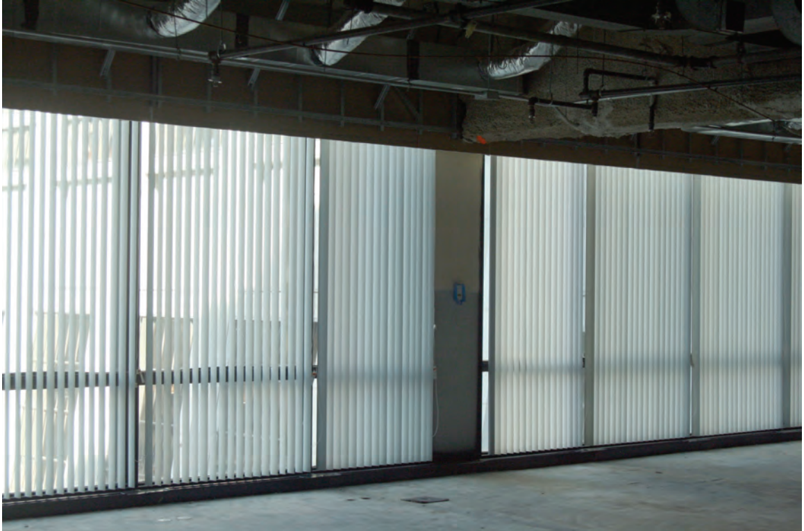
Figure 5.10: Venetian Blinds Shading the Windows on an Unfinished Tenant Floor. Source: the author, 2012.
