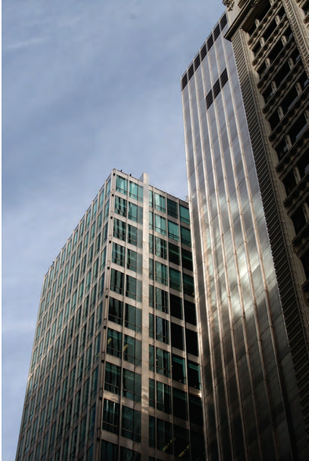
Figure 5.15: Stainless Steel Cladding and Green-tinted Curtain Wall Glazing. Source: the author, 2012.
