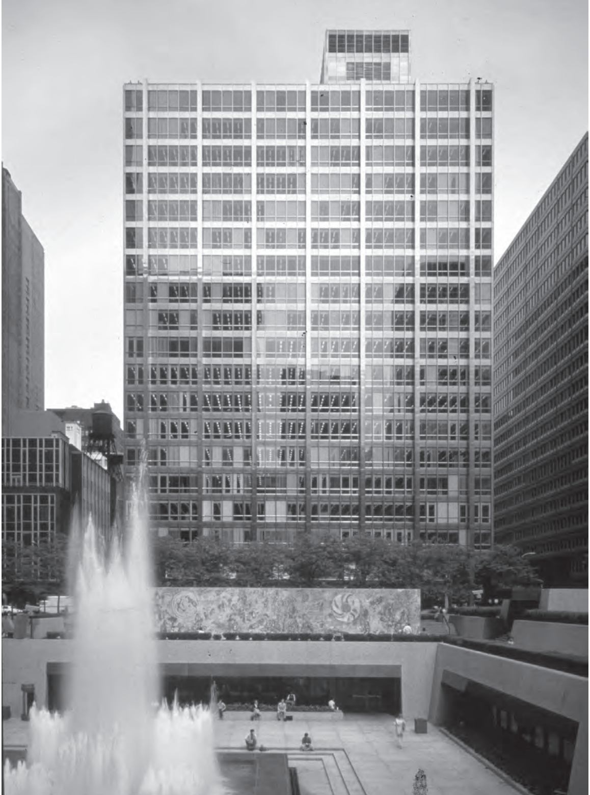
Figure B.12: View Looking East of Inland Steel Building. Source: SOM Archives, 1958.
