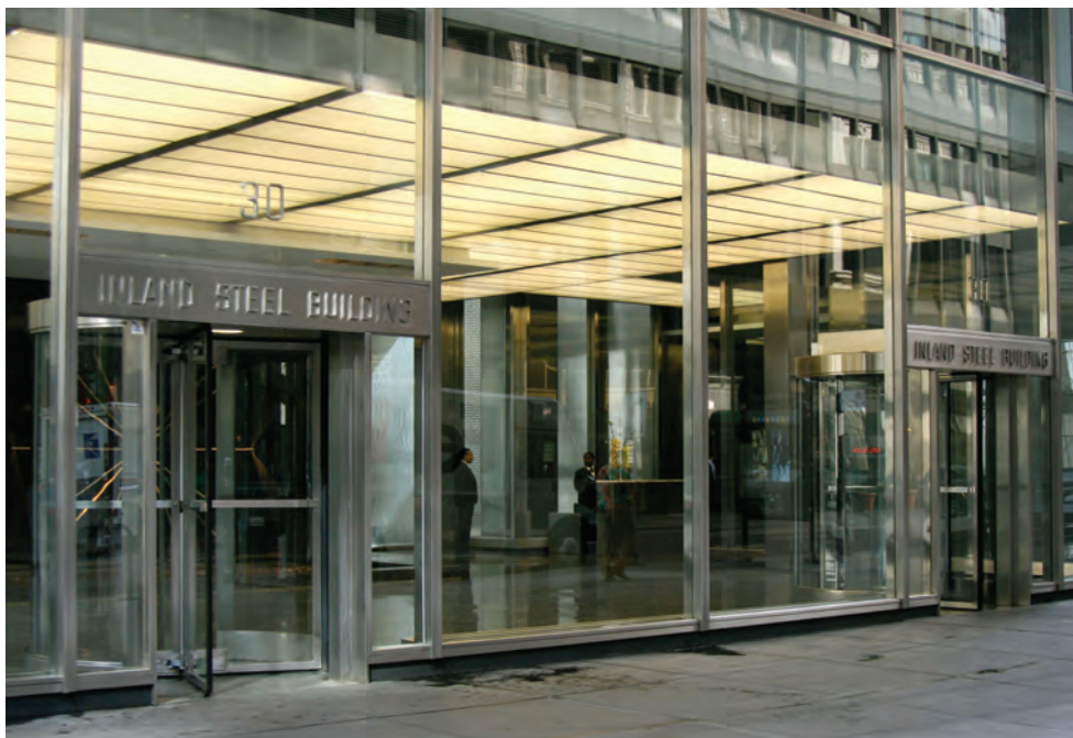
Figure 5.6: Entrance to Inland Steel Today. Source: the author, 2012.
