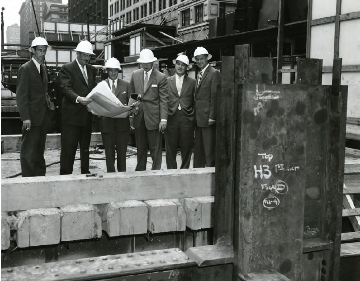
Figure B.4: Completed excavation and steel columns of the new Inland Steel Company building are inspected by a group from Inland and Skidmore, Owings and Merrill, architects of the building, who yesterday signed a lease for occupancy of its sixth floor. L-R: Bruce Graham, architect of Skidmore, Owings and Merrill; John O. Merrill, senior partner of the architectural firm; Joseph L. Block, president of Inland Steel company; William E. Hartmann, partner of the architectural firm; Neele E. Stearns, vice president of planning of Inland, and Fred Kramer, of Draper and Kramer, Inc., rental agents for the Inland building. Source: SOM Archives, 1957.
