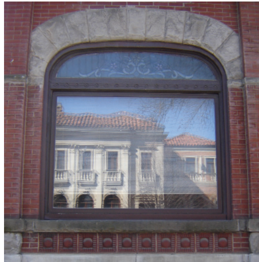
Image 6.9-B: Leaded glass window, pressed brick, and reflection of 1955 N. Burling "palazzo" (see Image 6.6), 2007 - above
