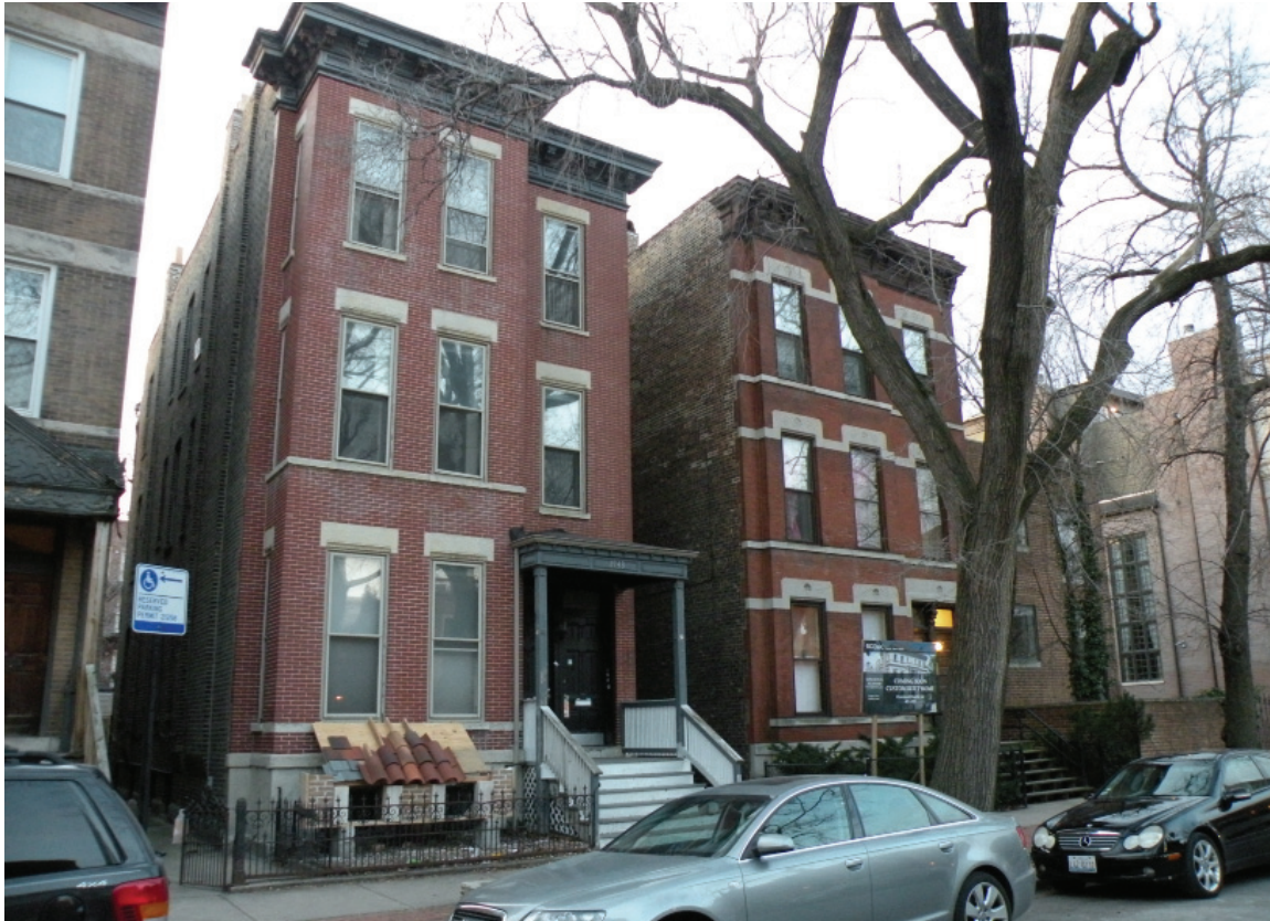
Image 6.7: Two three-flats at 1948 - 1950 North Burling Street, purchased as teardowns for a new wide single-family home, note the clay roof mock-up for the future Mediterranean-esque palazzo; 2012
