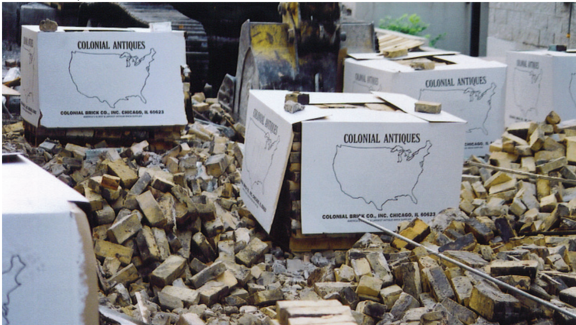
Image 8.8: Bricks being sorted and stacked following the demolition of the two-flat at 3532 North Fremont Street; Chicago common brick is sold across the country through the architectural salvage industry for construction, patios, and other uses; 2002
