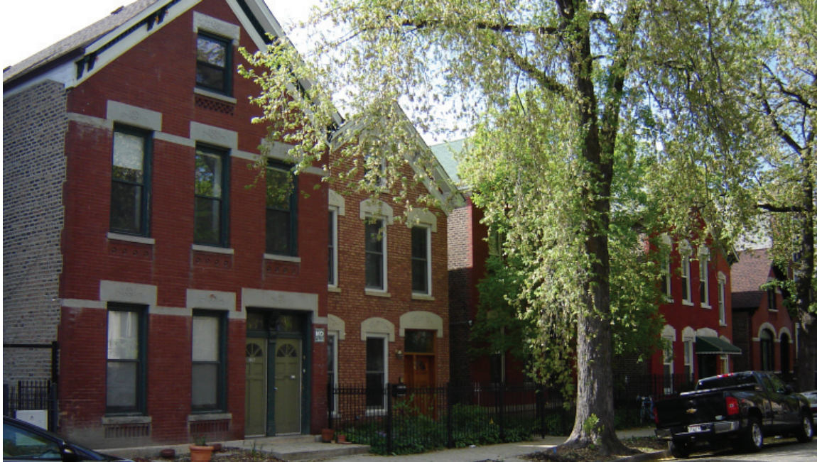
Image 7.2: East side of the 800 - 900 block of North Hermitage Street in the East Village District; only one side of the street was included due to the near complete redevelopment of the opposing side of the street; 2012
