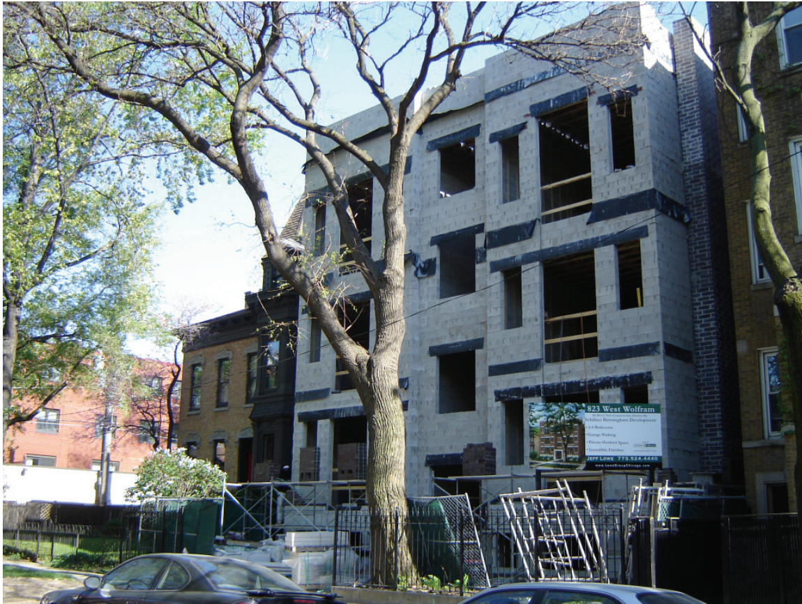
Image 8.15: A new six-unit condominium building rises at 823 West Wolfram Street without its final face brick veneer; May 2007
