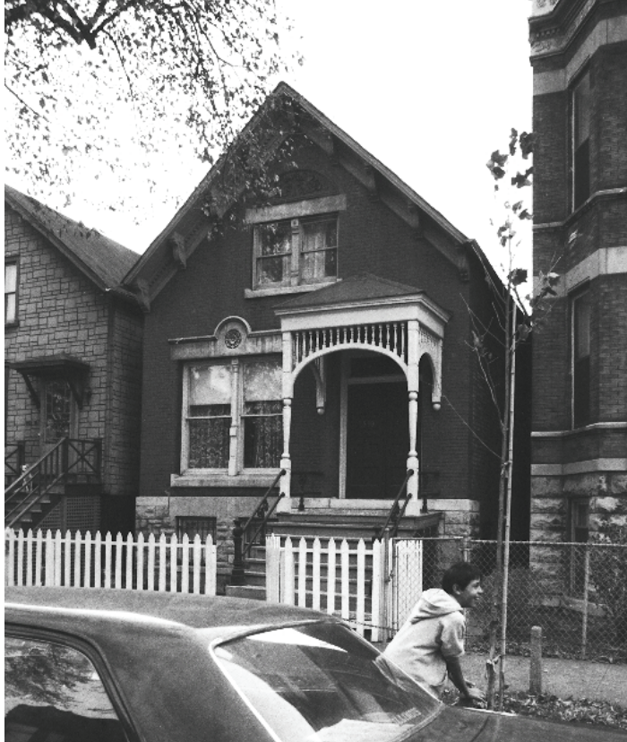
Image 8.4: (Left) 3530 North Fremont Street; orange CHRS-rated, well-detailed cottage house in Lake View photographed in the early 1970s for the Illinois Structures Survey
