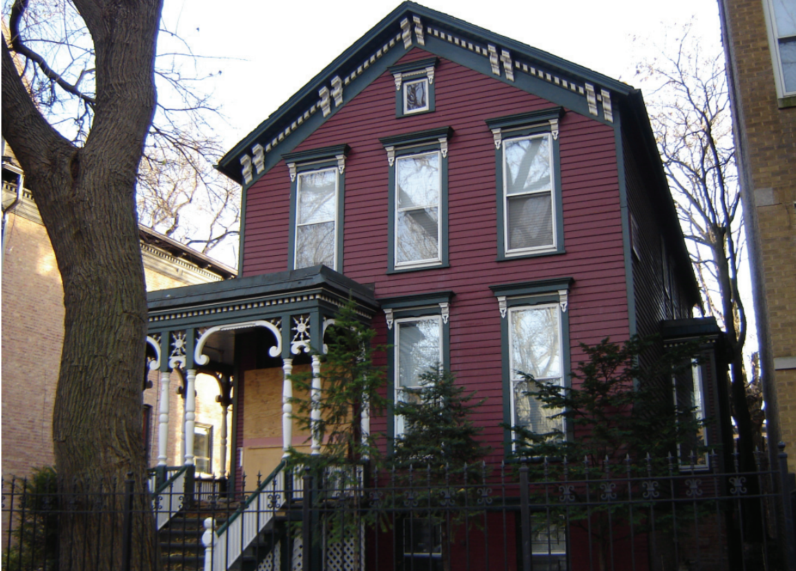
Image 8.13: 823 West Wolfram Street following a demolition sale of interior finishes and elements; November 2006
