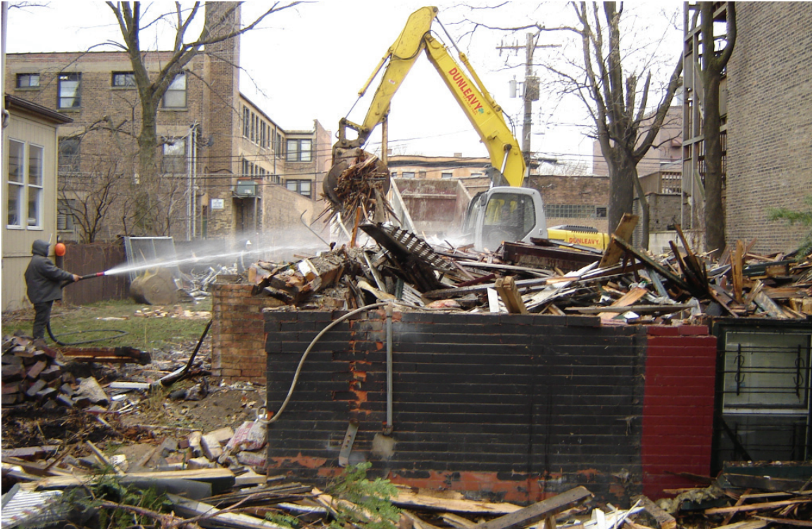
Image 8.14: 823 West Wolfram Street during speedy demolition; January 2007
