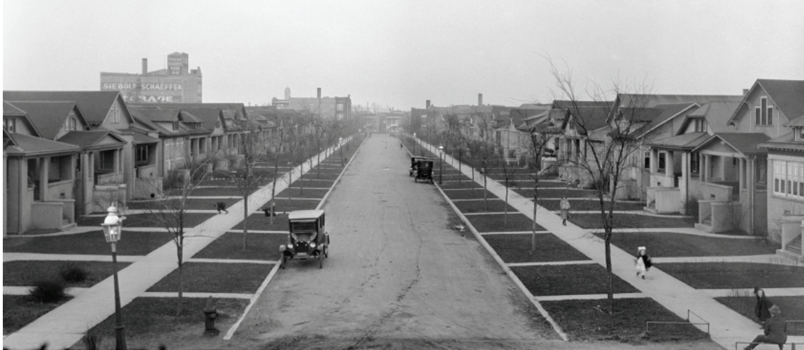
Image 2.12: New stuccoed bungalows on the 1700 block of West Arthur Avenue; c.1923 www.shorpy.com
