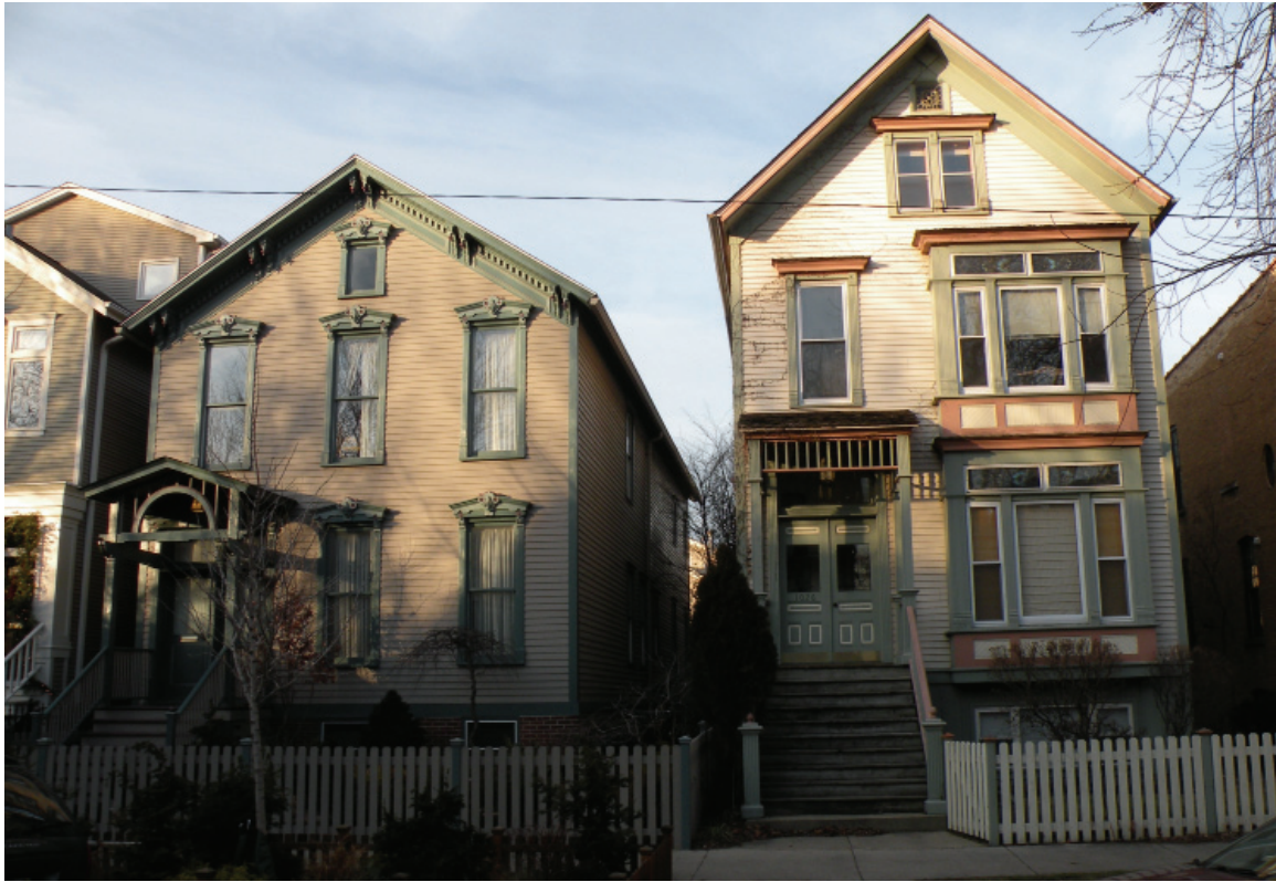
Image 2.3: Frame House (left) and later frame two-flat (right) at 1026-1028 W. Montana Street; 2012
