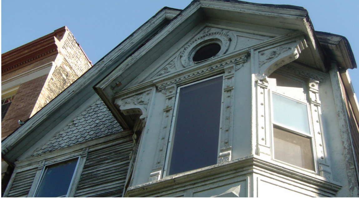
Image 8.8: 902 West Roscoe Street; gable detail showing pressed metalwork on bay window, May 2005
