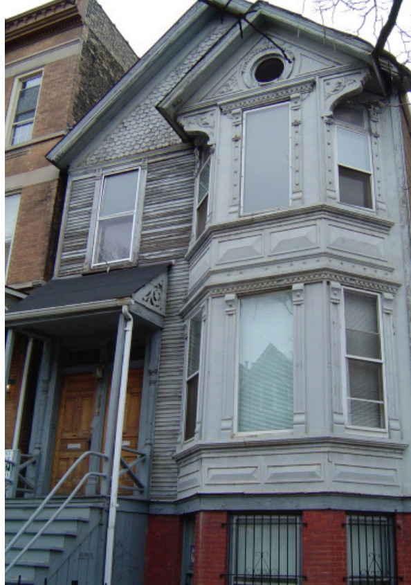
Image 8.10: 902 West Roscoe Street with an intact gabled, pressed metal bay with brackets and oculus
