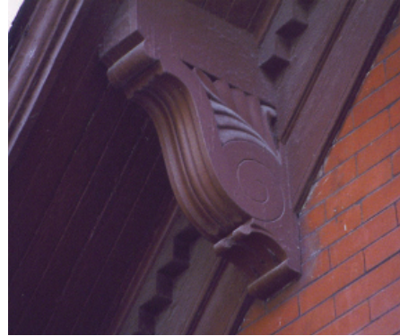
Image 8.5-C: (Above) The gable brackets featured uncommon simple incised details, 2001
