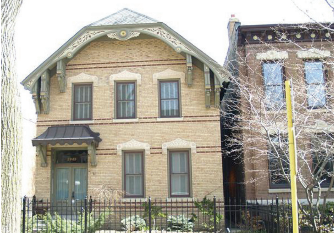
Image 8.3: 2049 North Mohawk Street, an atypical two-story brick home with intricate incised lintels and a elaborate barge board and brackets; the home was razed sometime after 2008, when this image was taken; see Image 8.2 for the house to the right at 2043; 2008
