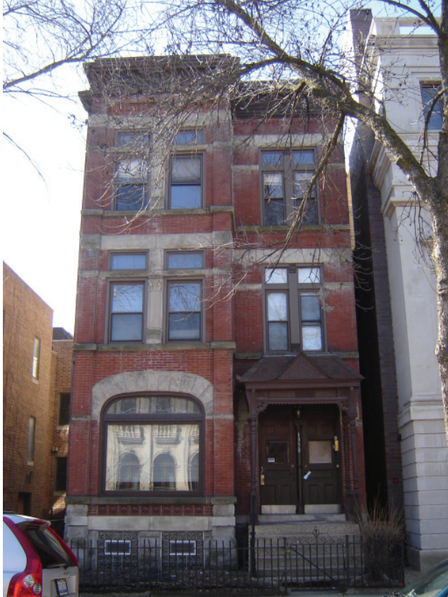
Image 6.9-A: 1958 North Burling Street ( before ), a three flat with pressed brick details, pressed metal cornice, and an intricate frame porch; the flat was razed in 2007, 2007 - left
