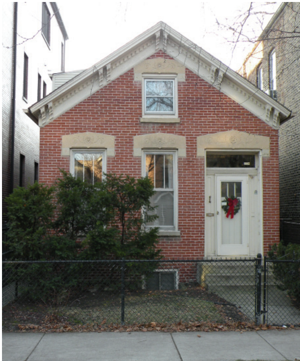
Image 2.6: Brick worker's cottage with incised limestone lintels and bracketed wood gable at 2234 N. Magnolia Street; 2012
