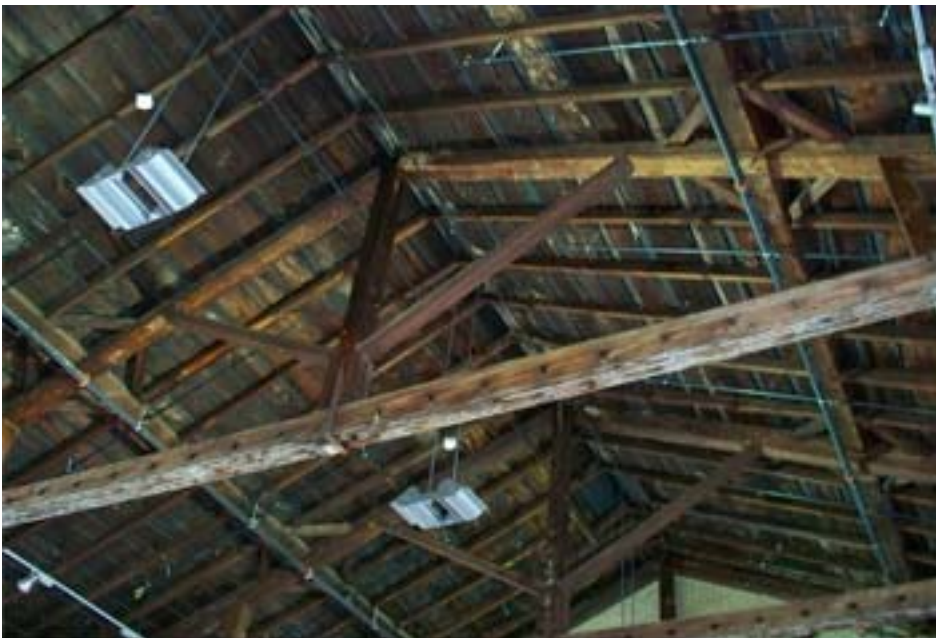
Figure 4: Exposed rafters in Chapel. www.nps.gov
