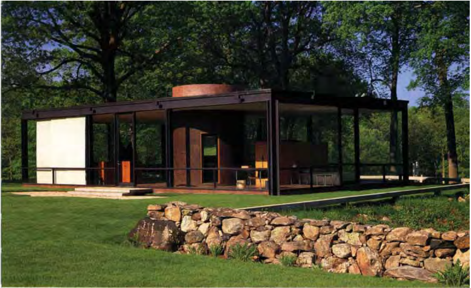
Figure 21. Philip Johnson Glass House (Image courtesy of S. Jenkins, The Houses of Philip Johnson )
