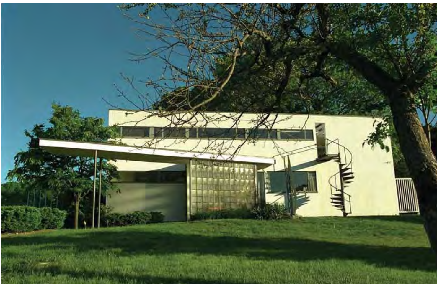
Figure 8. Walter Gropius House (Image courtesy of Historic New England)
