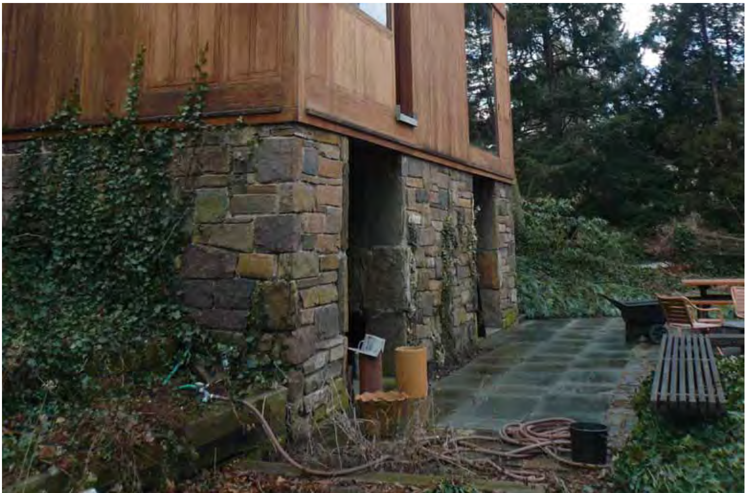
Figure 38. Fisher House stone basement level (Image author's own)
