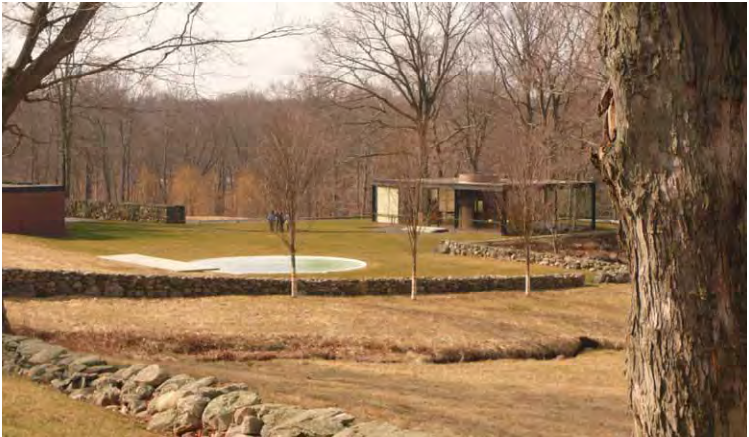
Figure 23. Glass House structure within site setting (Image author's own)
