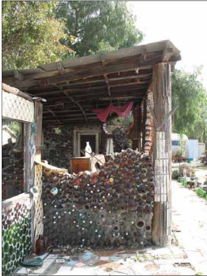
Figure 7.12: Cleopatra's Bedroom framing system. Recycled telephone poles constitute three vertical load bearing members of this structure (only one pole is pictured above). These poles are in direct contact with the cement ground (TSD 2007).
