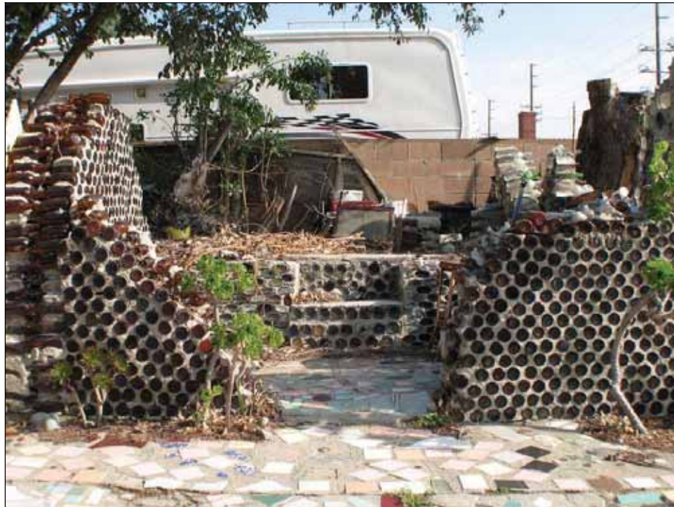
Figure 5.5: Bottle House constructed from Lucky Lager beer bottles. (TSD 2007)
