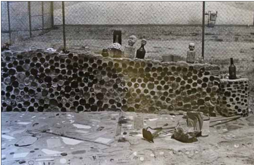
Figure 1.9: Original bottle masonry wall along east edge of property, ca. 1955. (CSUCI Archives)
