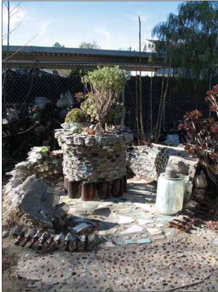
Figure 1.7: The Cabana (b. 1956), load bearing bottle masonry ruin. (TSD 2007)
