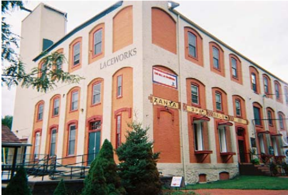
Figure 17-Laceworks in Lambertville-adaptive re-use project that now houses retail and services
