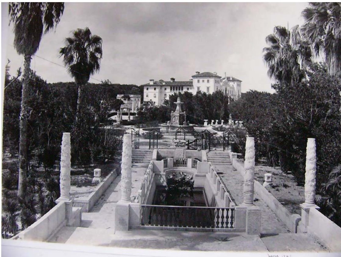
Fig. 15- Historic View of Marine garden form Peacock Bridge nearly completed showing historic plantings including Washingtonian palms
