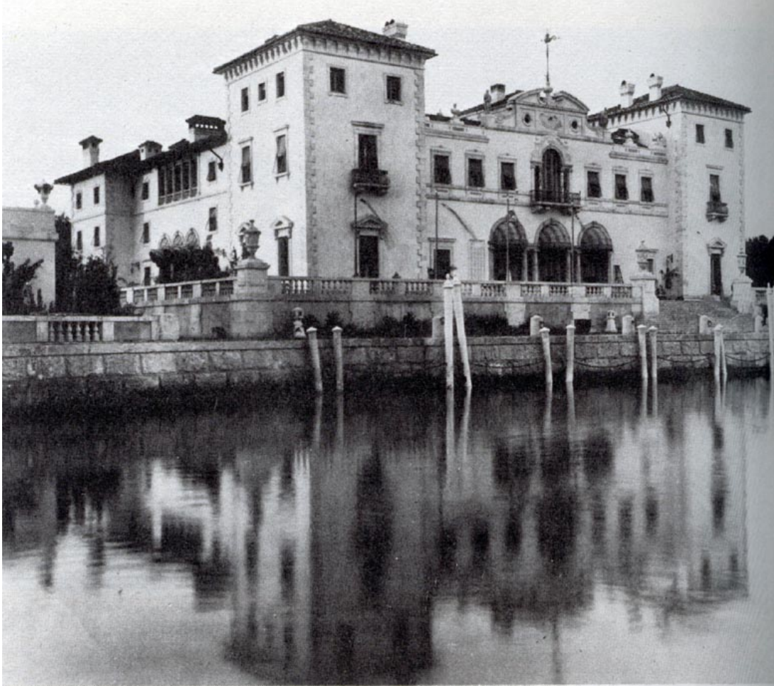
Fig.1- Historic view of East façade of the villa facing Biscayne Bay. (from Mahler)
