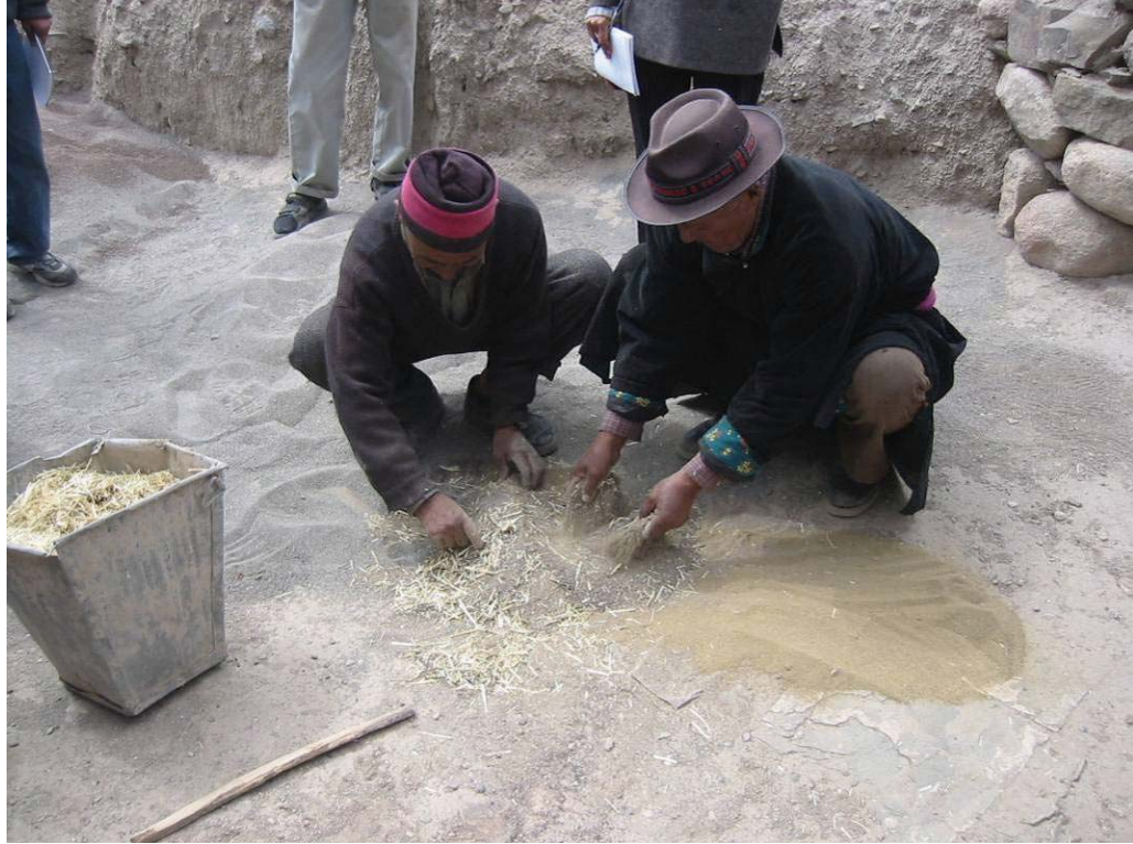
Figure 4 Preparation of raw material at site Source: Kuang Han Li
