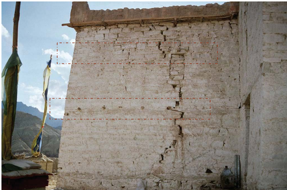
Figure 8 Wooden beams located at intervals, temple at Basgo Source: Kuang Han Li
