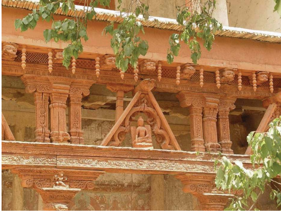
Figure 15 Wooden ornate porch, Alchi, Ladakh
