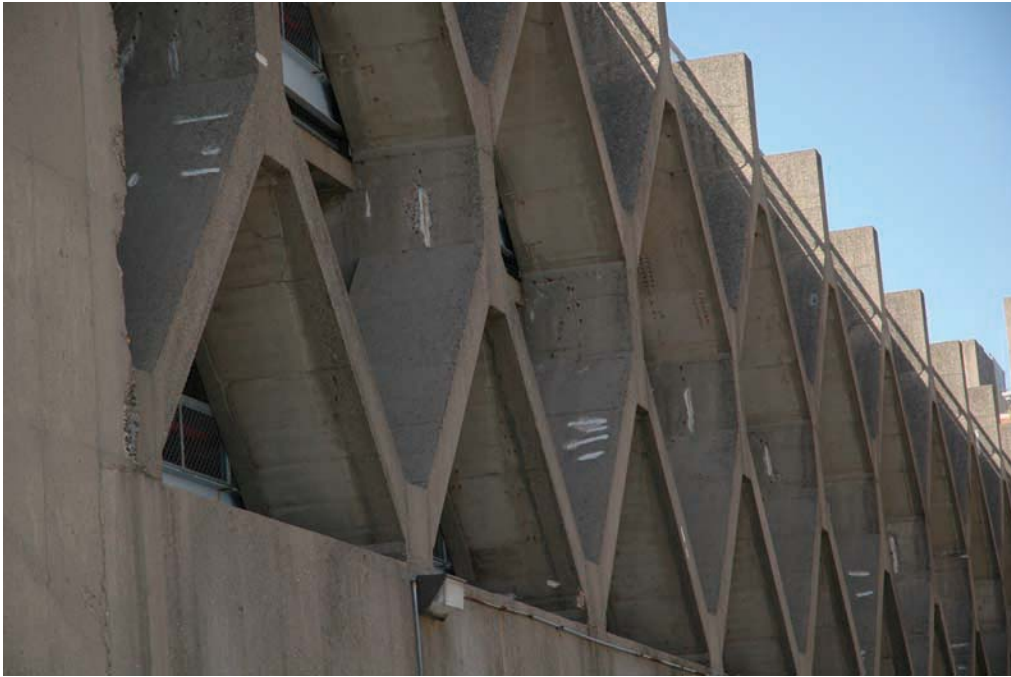
Image 37: Current appearance of concrete grid structure
