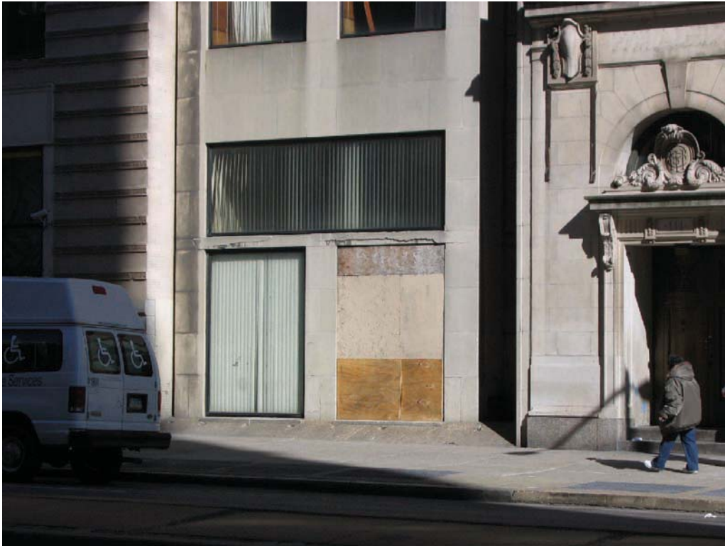
Image 40: Current condition of office annex
