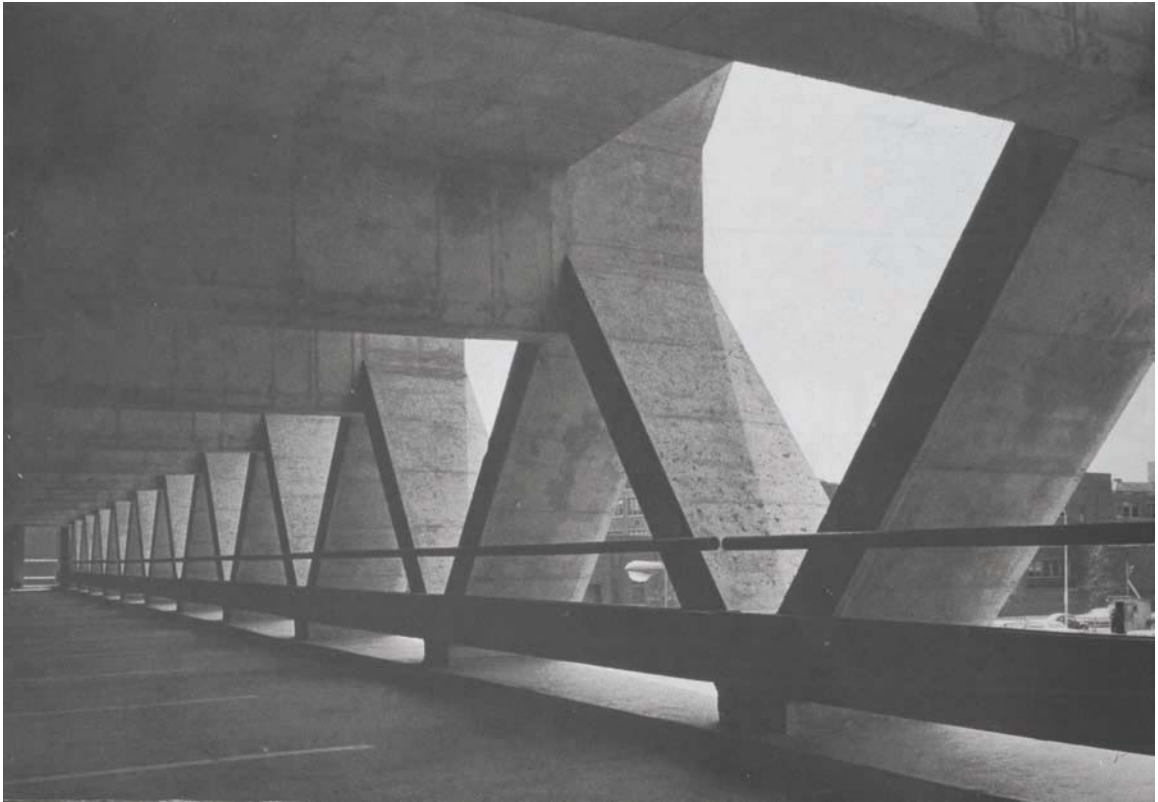
Image 35: View of concrete grid from the interior of the garage
