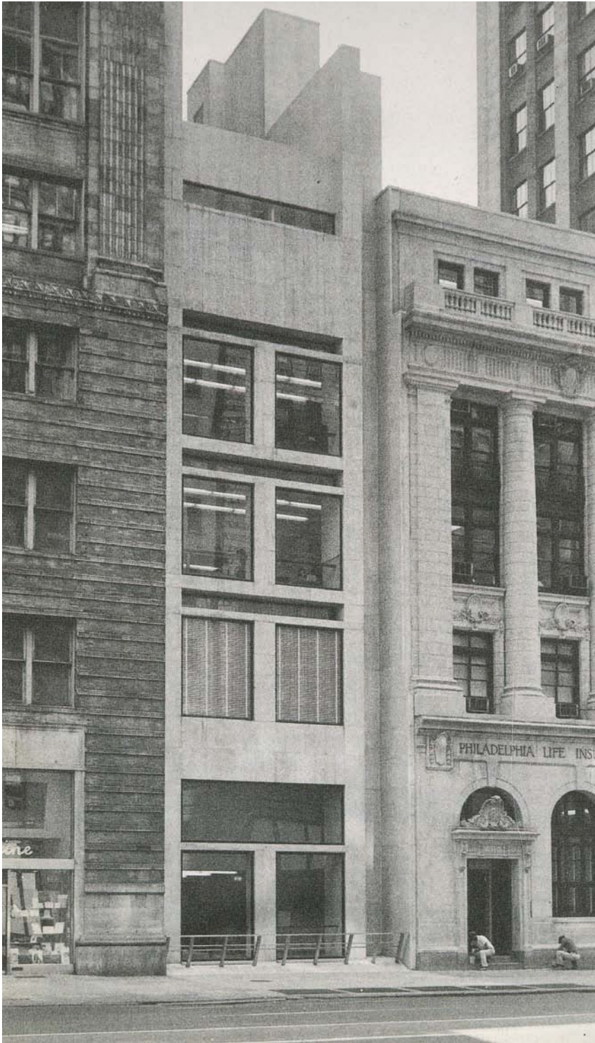
Image 39: Office annex to Philadelphia Life Insurance Company headquarters
