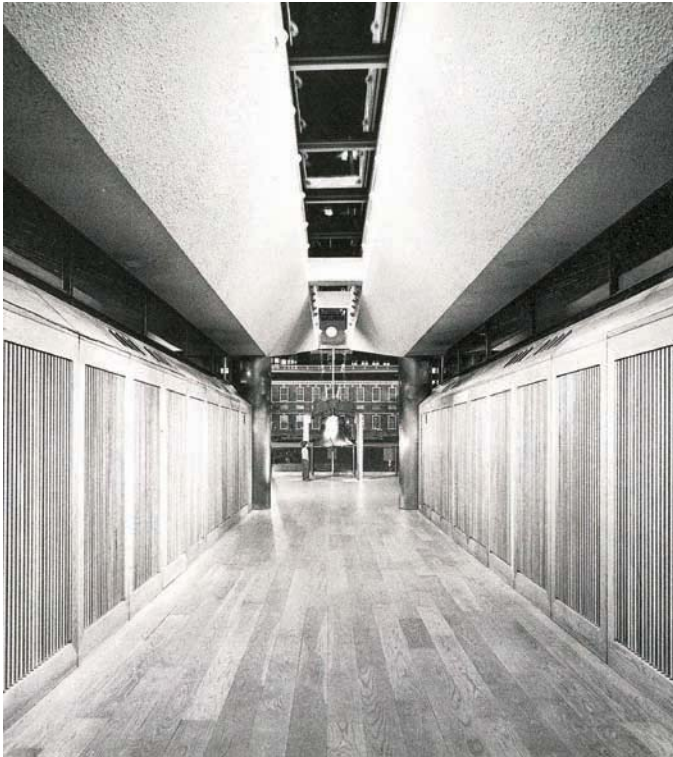
Image 15: Interior of Liberty Bell Pavilion
