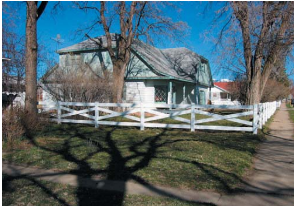
Figure 38-Preserved Residence on Grand Avenue, Mancos, 2005
