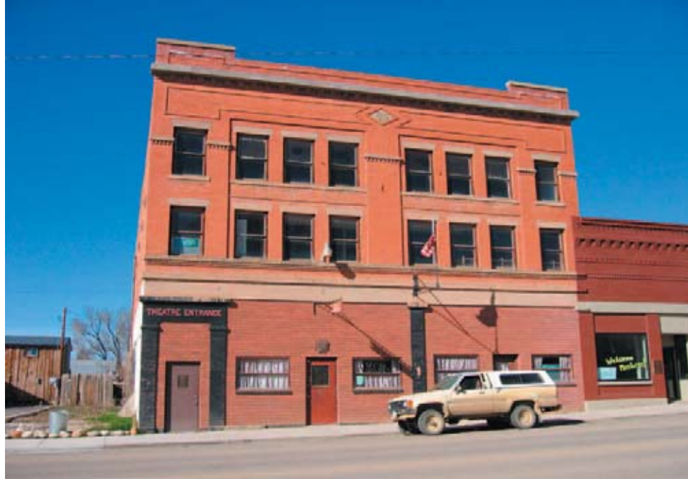
Figure 41-Mancos Opera House, Mancos, 2005
