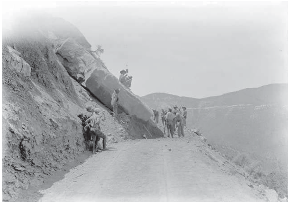
Figure 8-Road Repair c. 1923 (Source: Denver Public Library)
